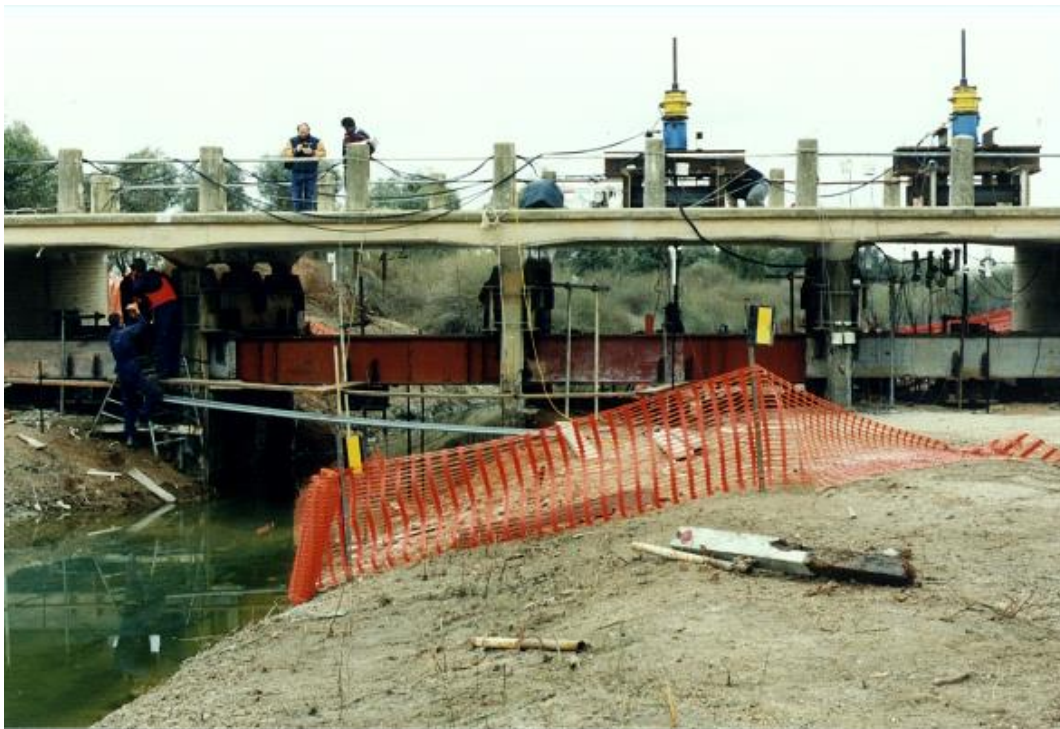
Load Testing of Disused Concrete Flat Slab Bridge using Ground Anchors
