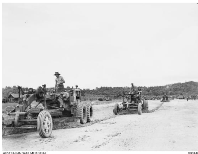
Graders operated by No 8 Airfield Construction Squadron, RAAF, at work building the airstrip at Tarakan Island, Borneo - May, 1945.
