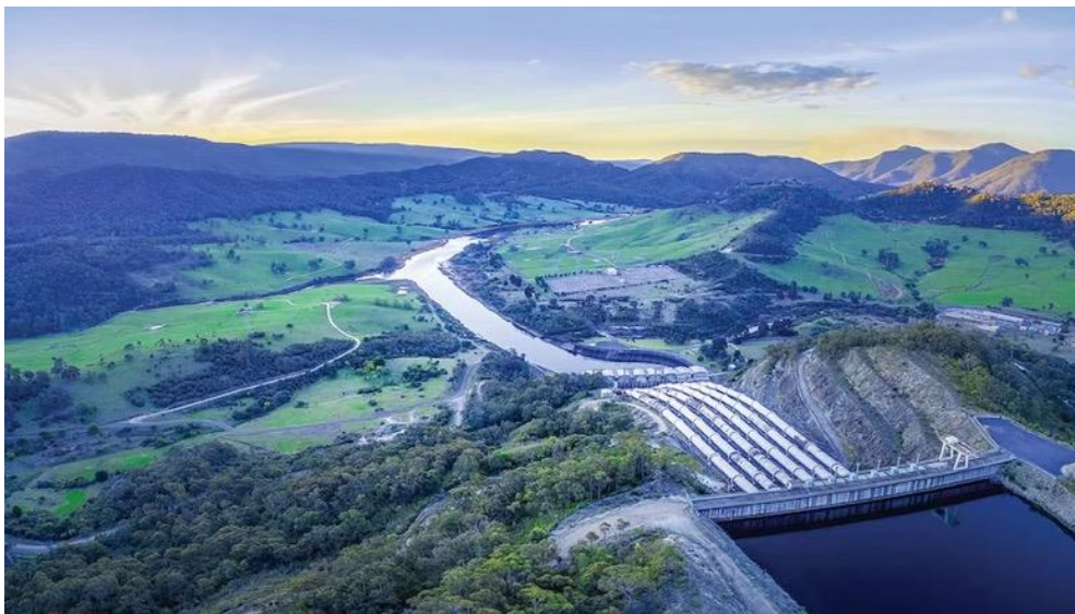
Snowy Hydro 2 Project.
