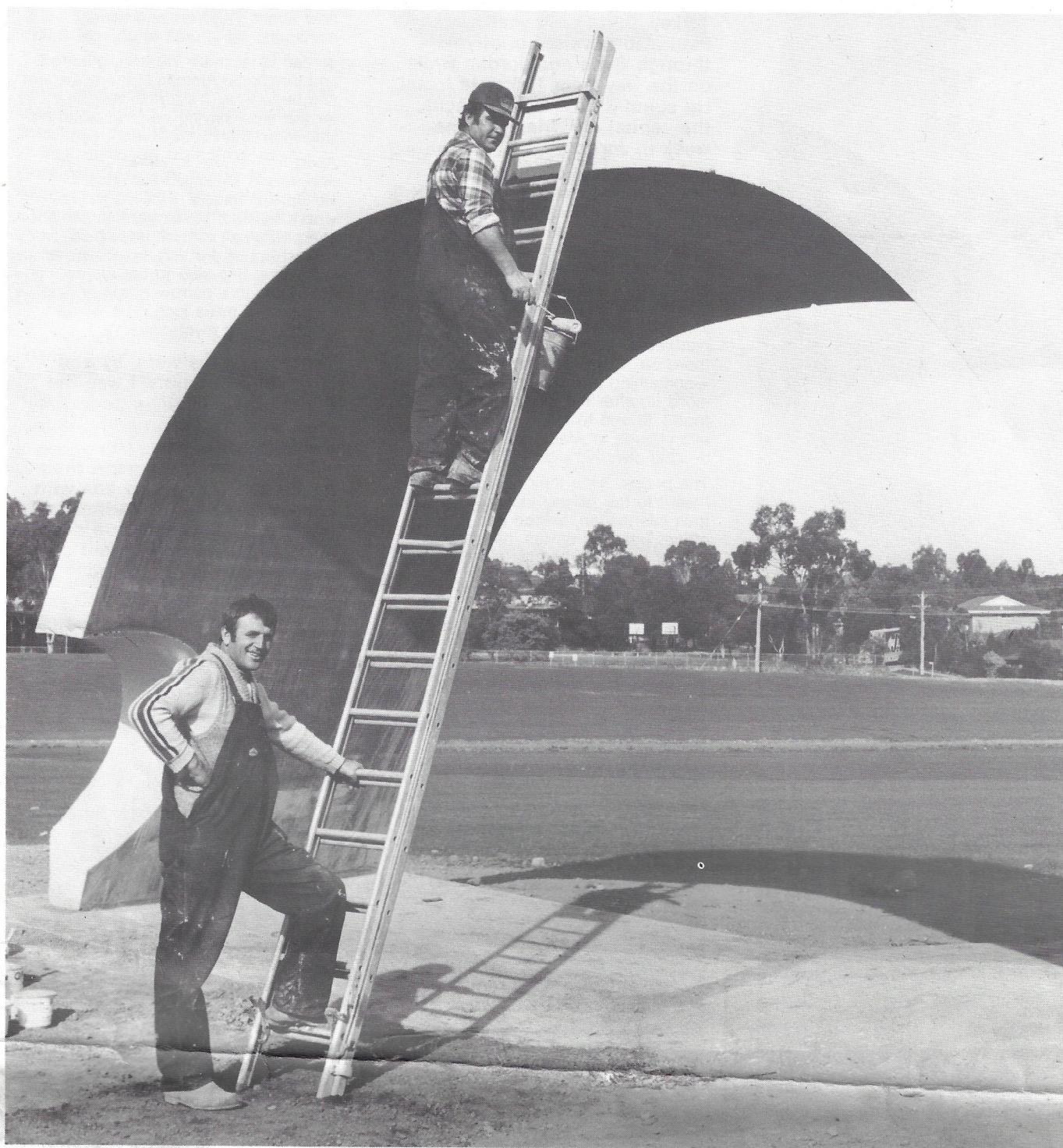
The Balwyn Peril? Two RCA workers, Dominic Plandido (on the ladder) and Ivon Cirjak, had a rather unusual task recently. They cleaned and painted a snail culvert section which has been installed above ground on the reserve adjacent to the Eastern Freeway in North Balwyn (near the pedestrian overpass). The culvert section is the same as those used in the undergrounding of Koonung Creek. It should prove to be of interest to members of the public—and to any children playing hide and seek
