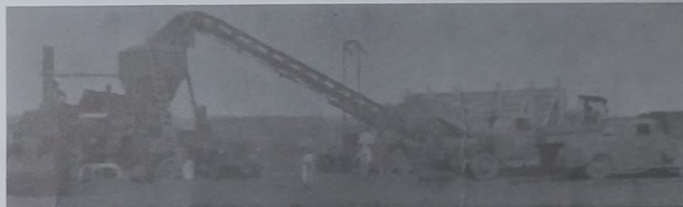
• Portable plant mixing gravel and bitumen at Banka for the Stuart Highway
