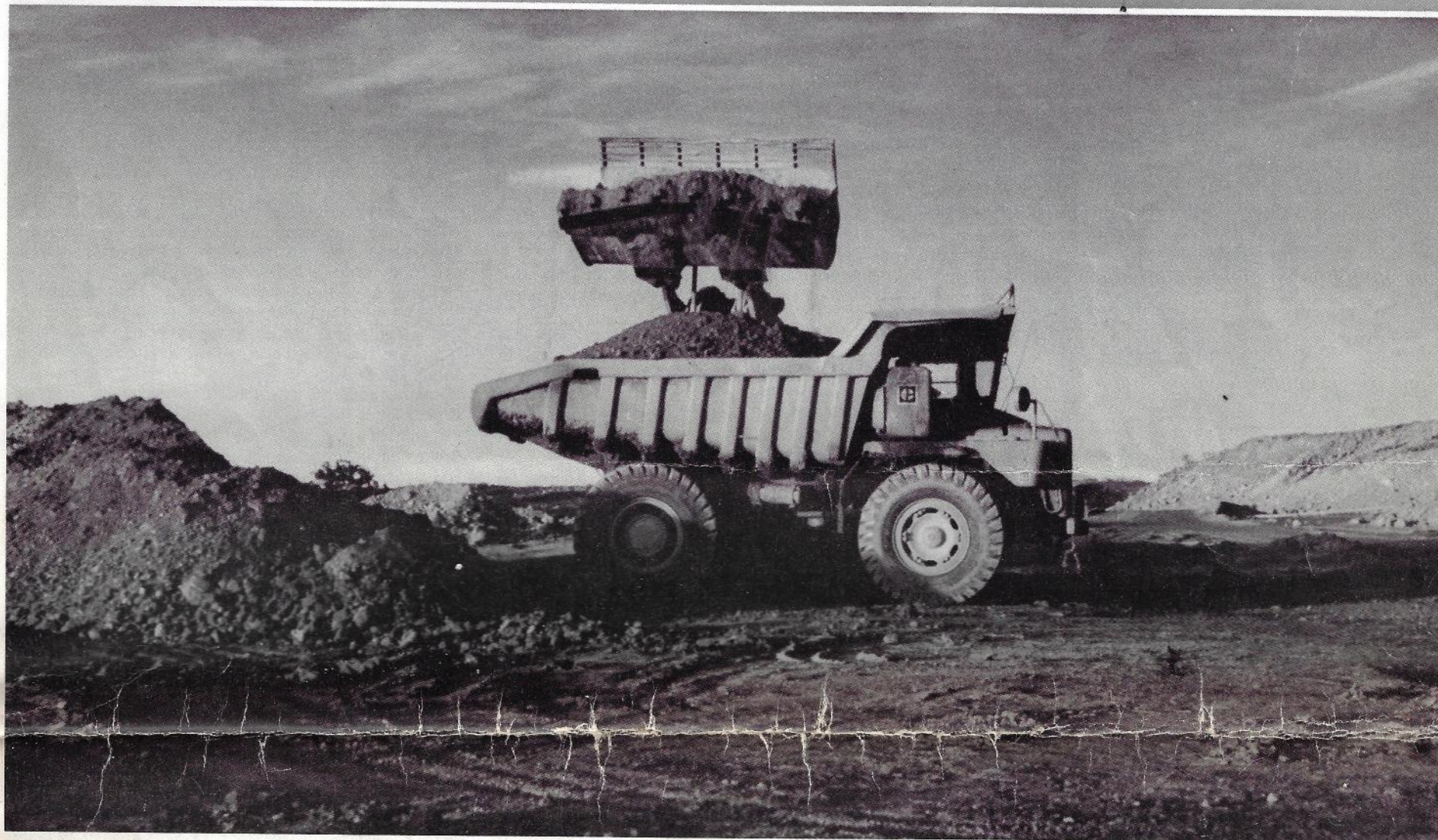
• Earthworks construction on the Bypass of Benalla.
