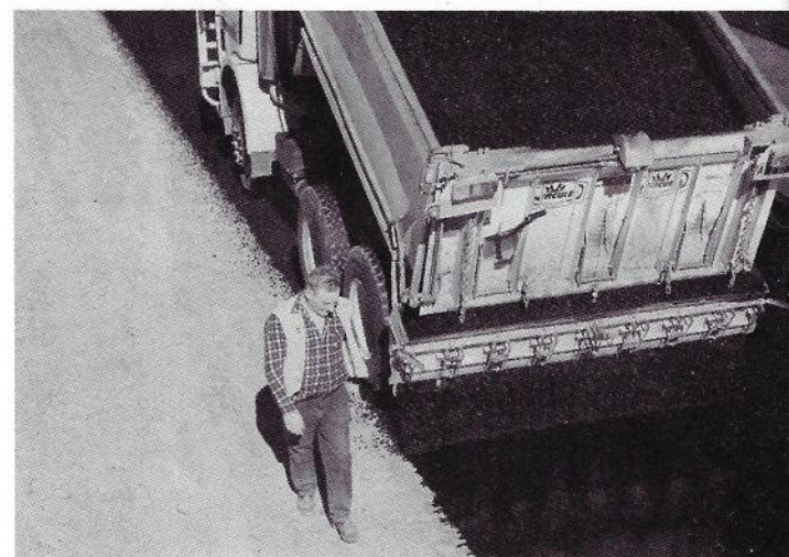
• Wally English, Spreader Operator, inspects his work on the bypass.
