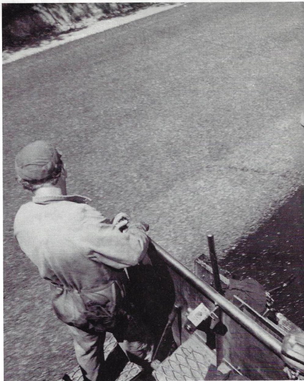
• It's teamwork that counts. Ernie Hade (Sprayer Operator) checks that the bitumen is evenly sprayed. Sandy (Spreader Operator) prepares to remove the starter paper.
