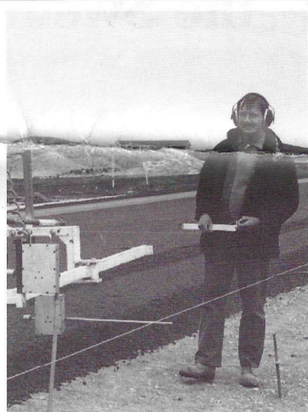
• Bruce Waixel ('The Boss') inspects the stringline to secure that the position is accurate.
