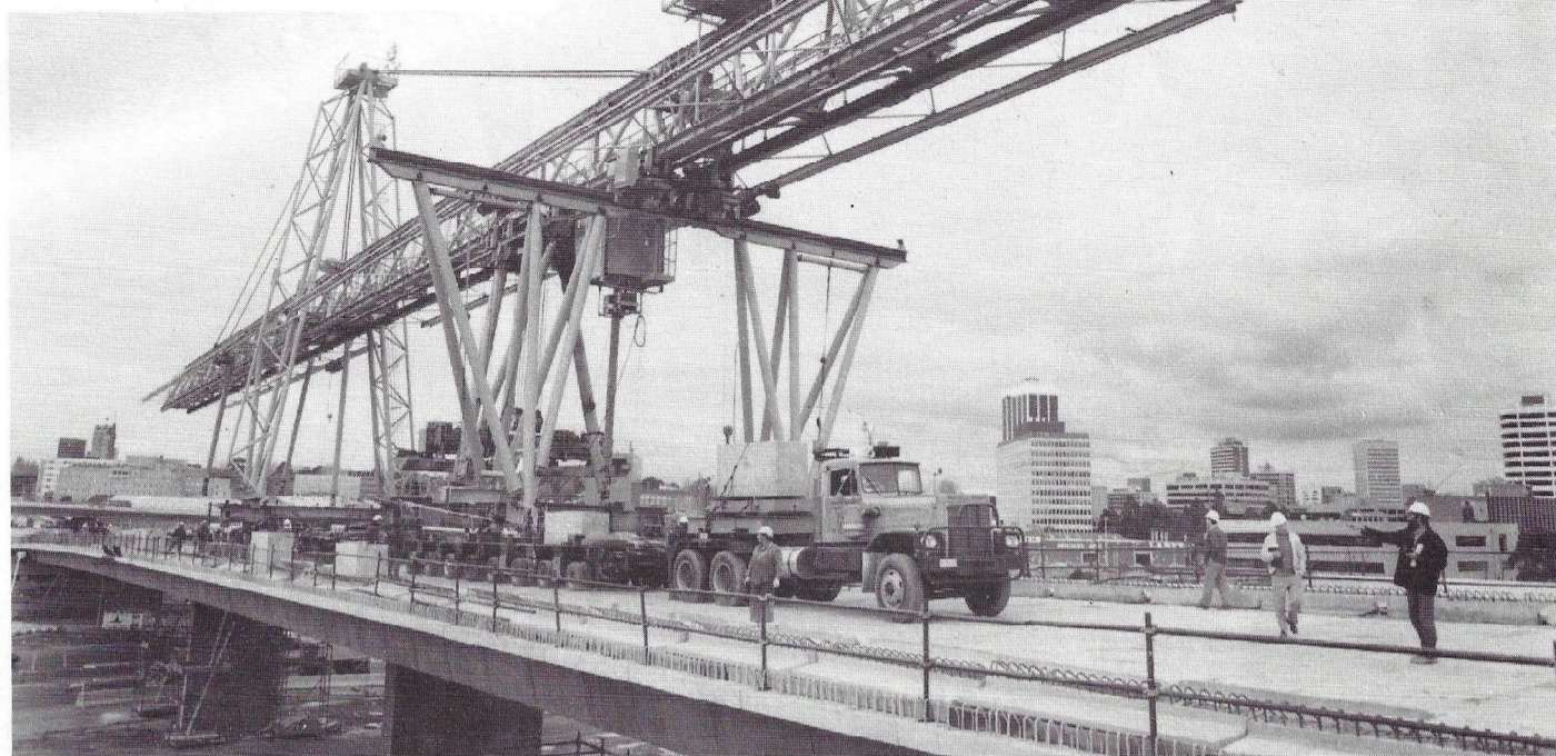
• You won't see this sight very often—a 200 tonne launching girder on the move!
