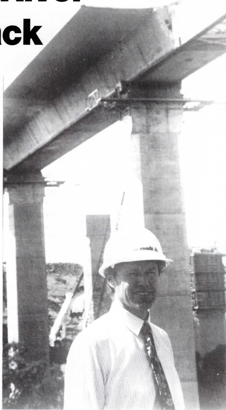
■ Graham Gilpin in front of Maribyrnong River Bridge in construction stage
