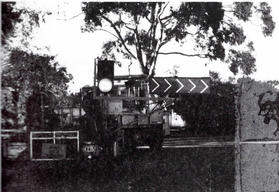
■ Trailer being used on the job
