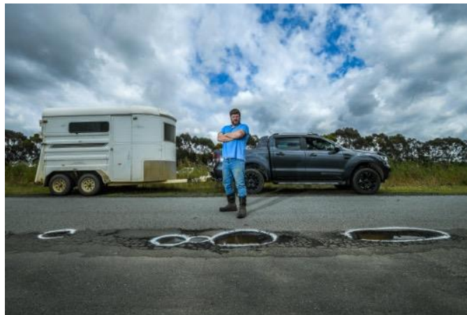
The Goulburn Valley Highway.
