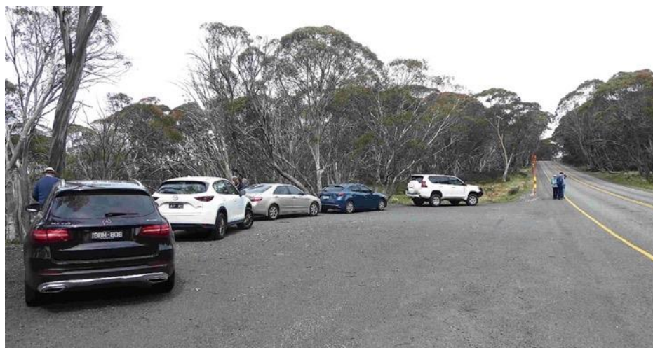
Inspecting the frost-free pavement at Brandy Creek.
