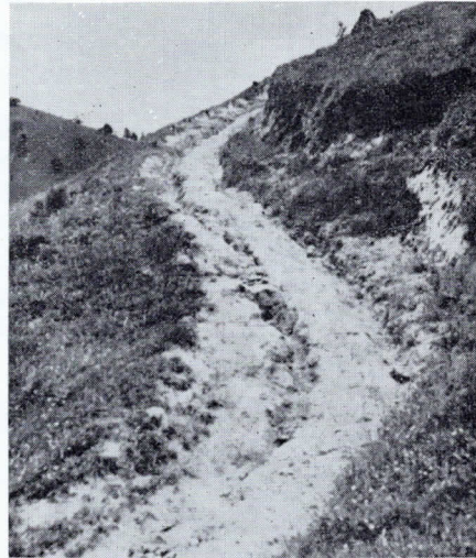
Typical isolated settlers road before reconstruction by C.R.B.
