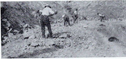
Road construction by pick and shovel methods.
