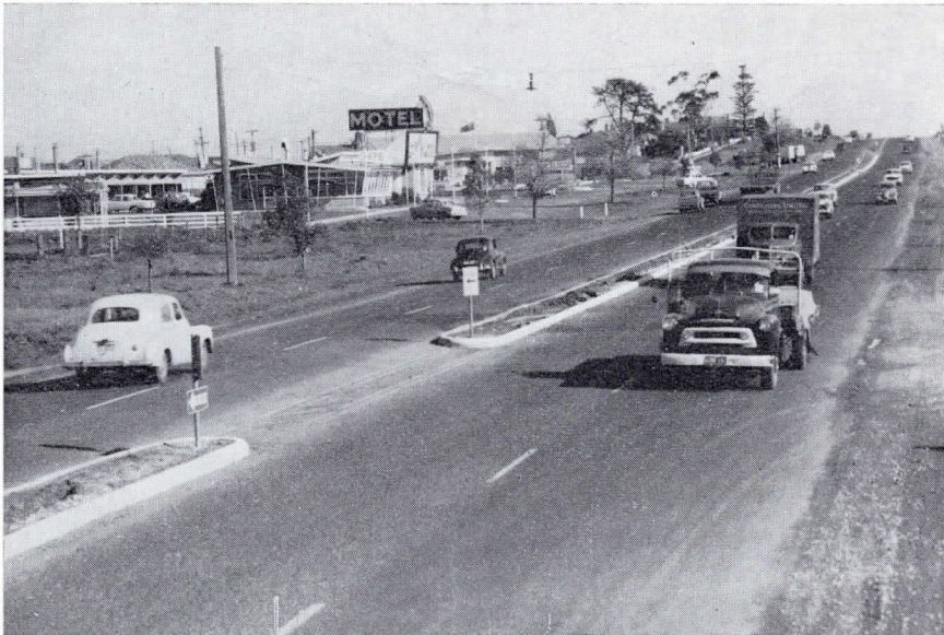
Princes Highway East — first stage of duplication between Oakleigh and Dandenong.
