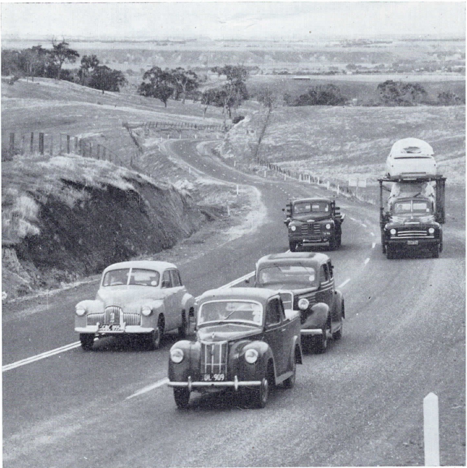
Additional climbing lane for slow moving traffic Western Highway near Bacchus Marsh.
