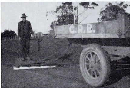
Triangular Webster drag used in road maintenance.
