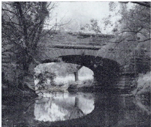
Masonry bridge on Calder Highway at Woodend, constructed 1862.
