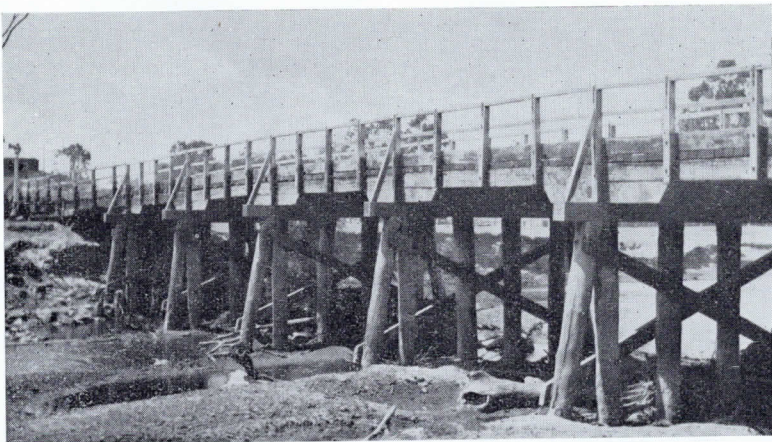
Typical timber bridge in existence 1913.
