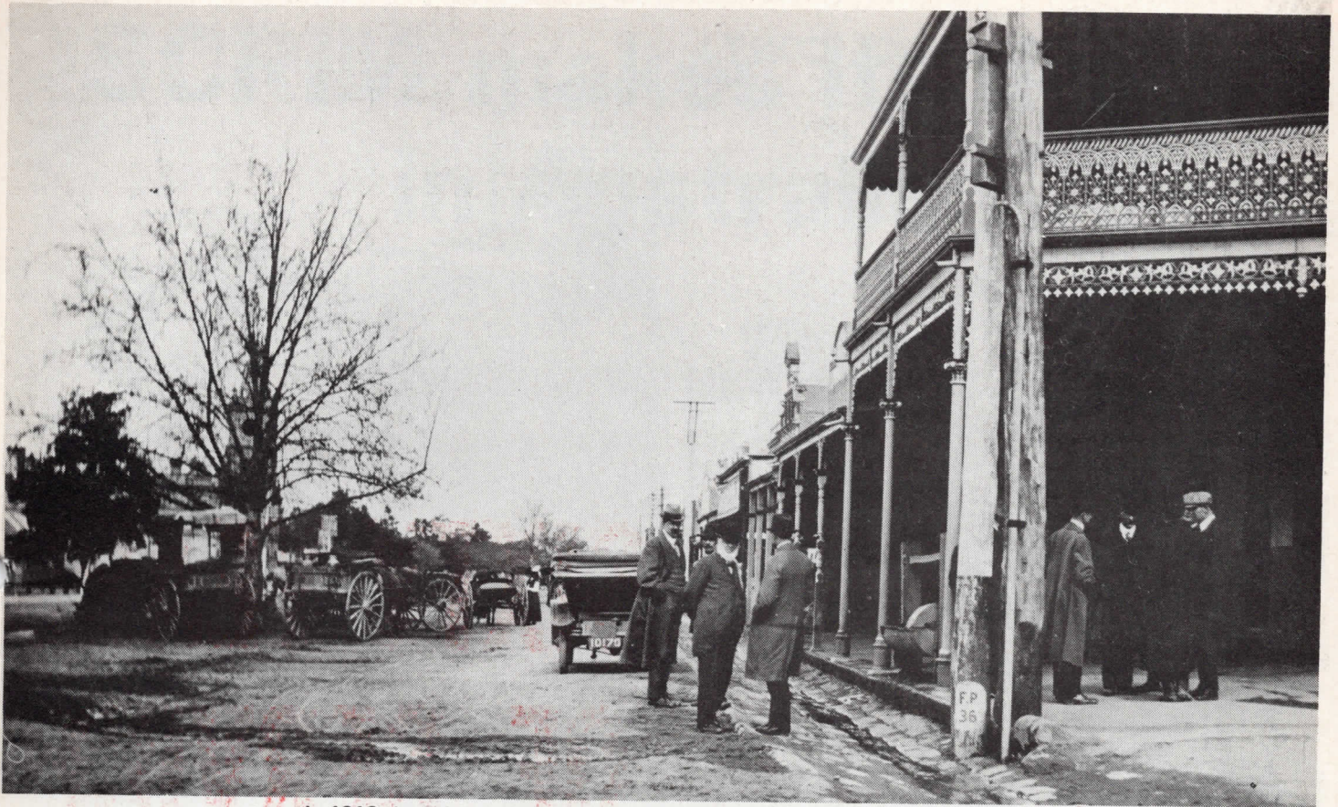
In 1913 the Princes Highway East in Dandenong looked a bit muddy.
