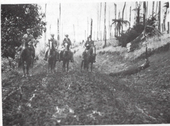
Board Members inspecting the Mirboo-Leongatha Road in 1913
