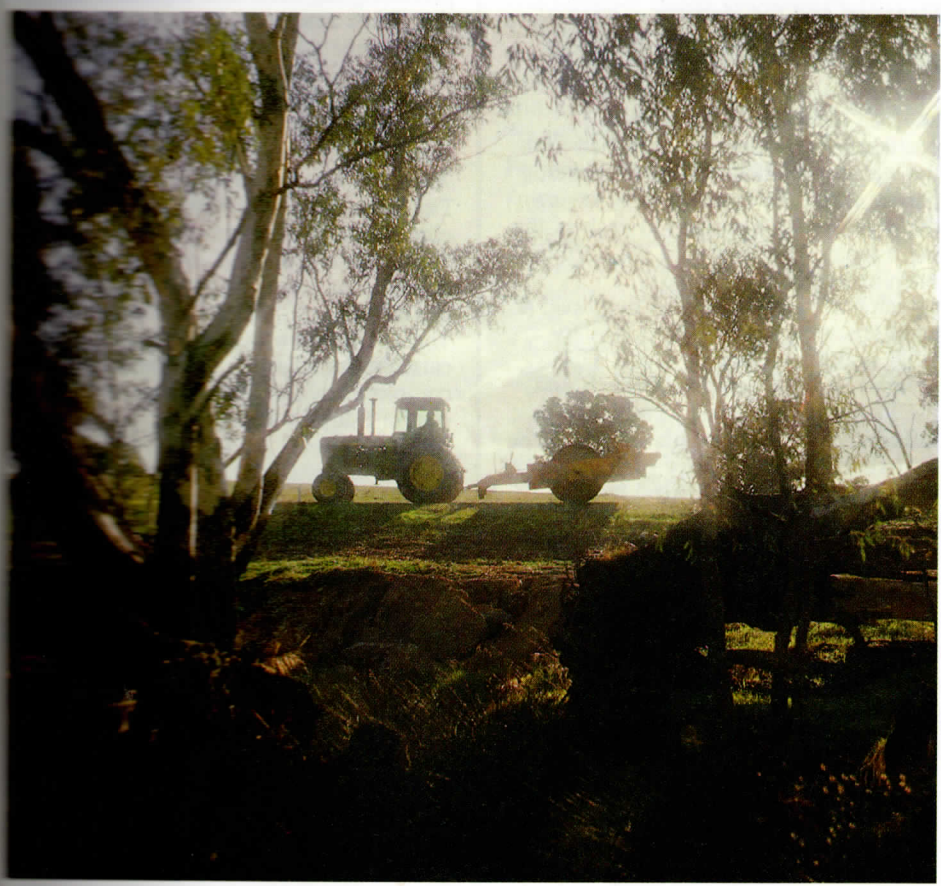
Left: Early morning sunlight filtering through the trees on the Calder Highway duplication project at Big Hill
