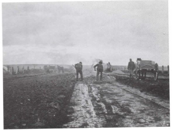
ABOVE: ROADS WERE BUILT MANUALLY WITH HORSE AND CART, 1913.
