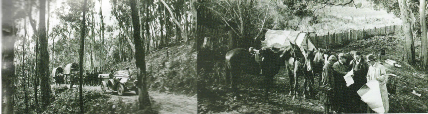
ABOVE: ENGINEERS DISMOUNT TO DISCUSS ROAD PLANS. LEFT: DARGO ROAD, 1913.
