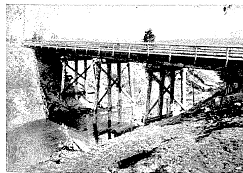
Bridge over Albert River. Constructed with flood damage grant, 1935-36.
