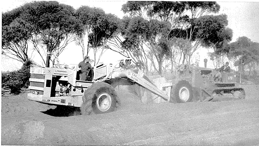
Loading a tournapull scoop with the assistance of an HD16 bulldozer. When loaded the tournapull scoop can transport material at relatively high speeds.
