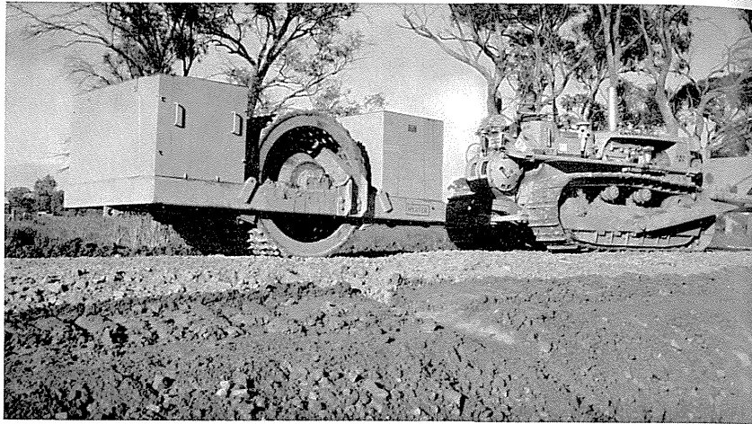
Loading a tournapull scoop with the assistance of an HD16 bulldozer. When loaded the tournapull scoop can transport material at relatively high speeds.
