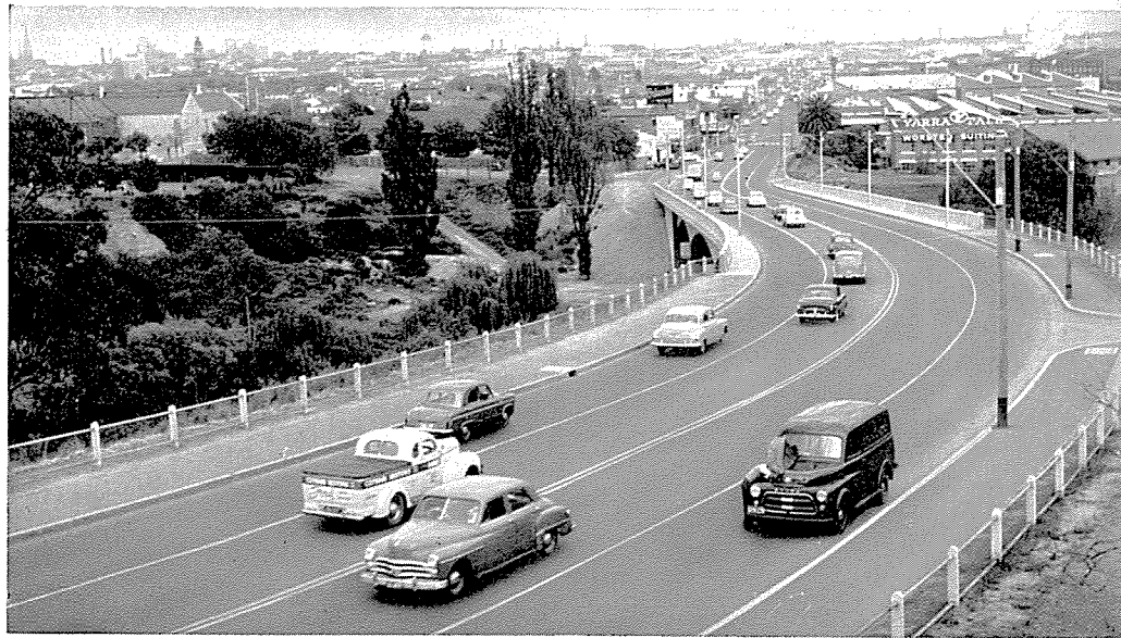
Johnston Street bridge, completed 1957.
