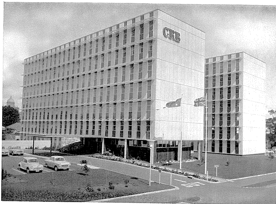
C.R.B. Head Office, Kew. From 1913 until 1929 the C.R.B. was accommodated in the Titles Office and from 1929 until 1960 in the Exhibition Buildings. The present offices were occupied in December, 1960.
