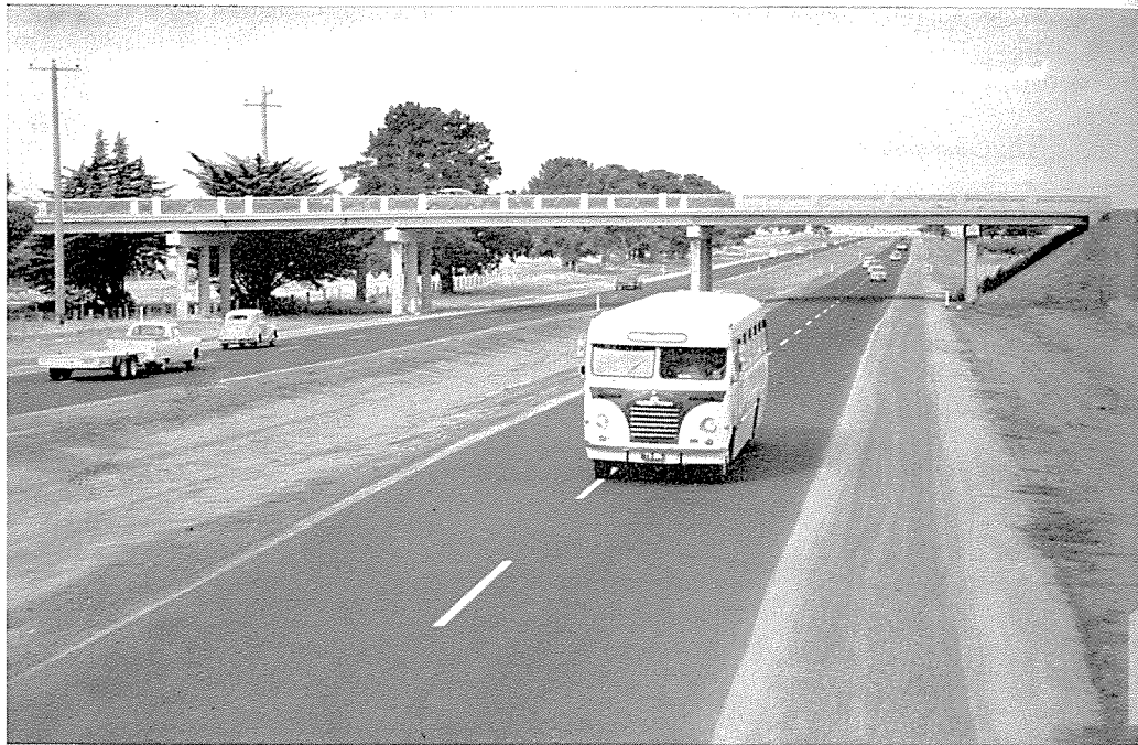
Maltby by-pass road at Duncans Road overpass, completed 1961.
