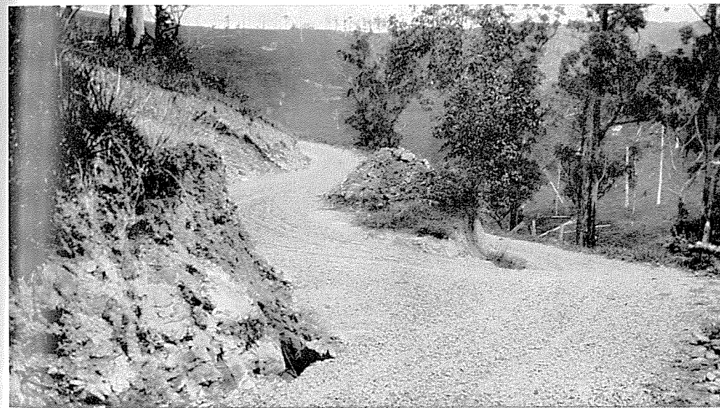
Typical isolated settlers' road constructed under C.R.B. supervision.
