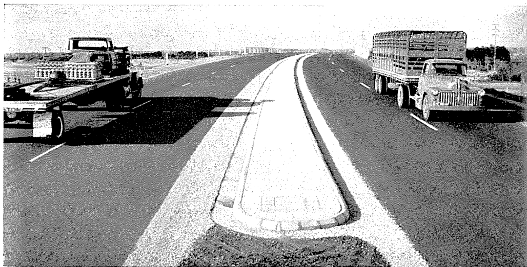
Princes Highway West—Corio Overpass, completed 1958.
