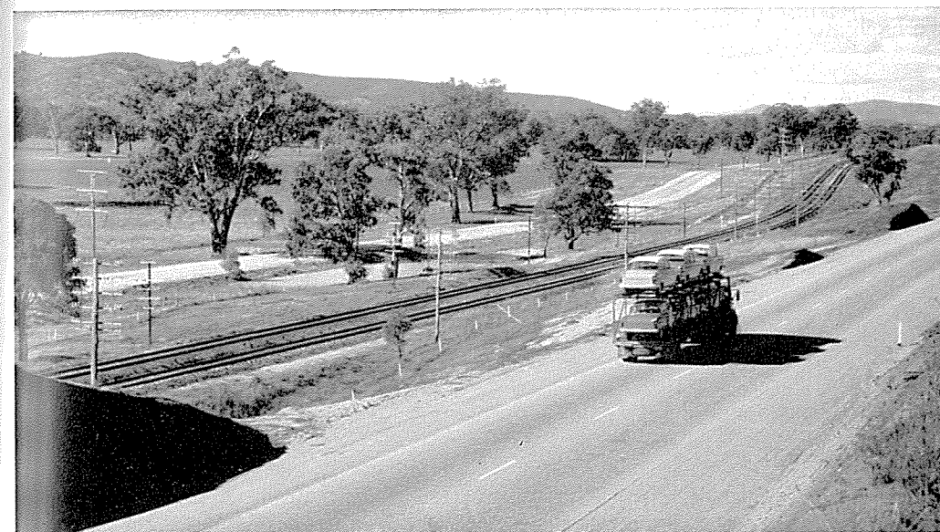
Hume by-pass road between Chiltern and Barnawartha, completed 1962.
