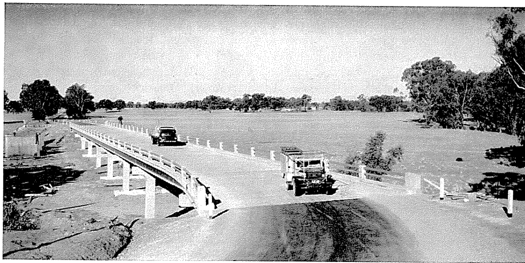
Bridge over the Campaspe River at Elmore, completed 1962.
