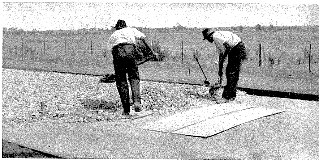
Hand-spreading road metal for waterbound Macadam, in early 1930's.
