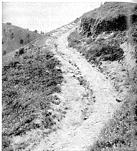
Typical isolated settlers' road before reconstruction.
