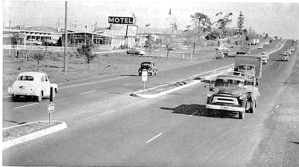
Princes Highway East. First stage duplication of pavement between Oakleigh and Dandenong.
