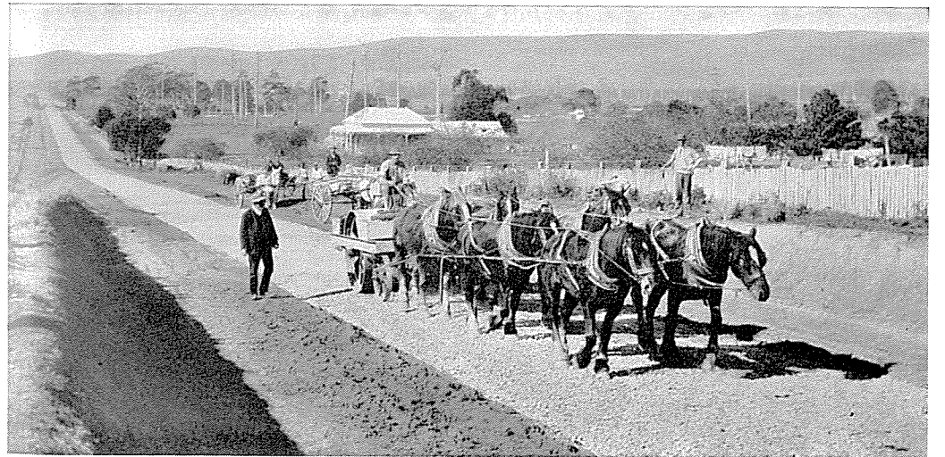
Horse-drawn roller in use on Main Gippsland road (now Princes Highway East) on Moe River flat, in second decade of this century.
