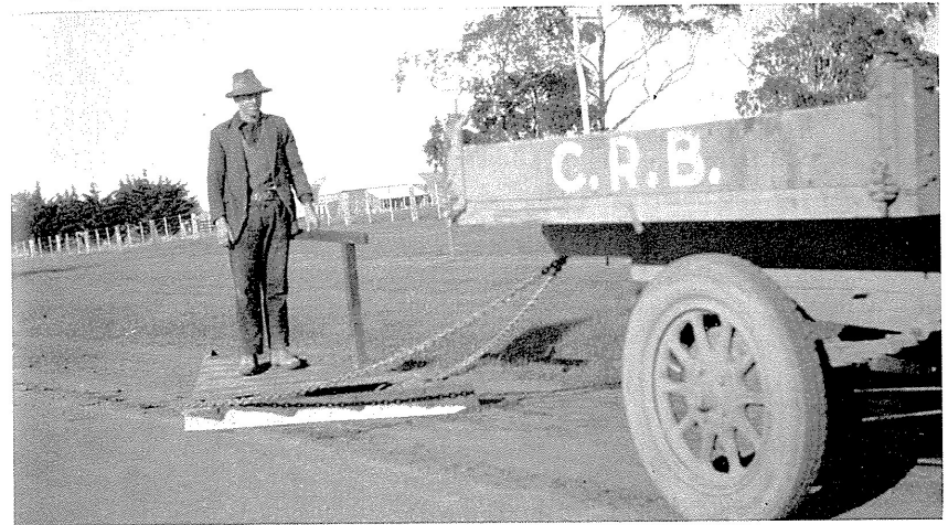
Triangular Webster drag used in maintenance.
