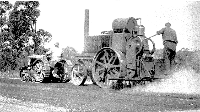
300-gallon, tractor-drawn sprayer, still used in late 1920's.
