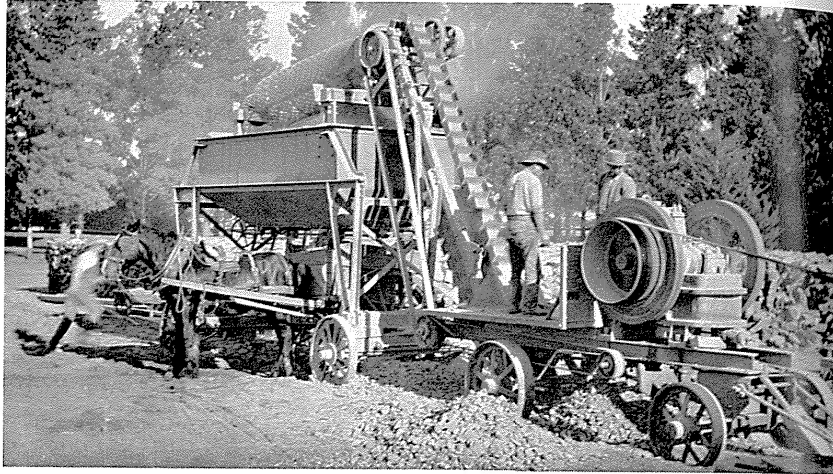
Typical early portable crushing plant for production of road metal.
