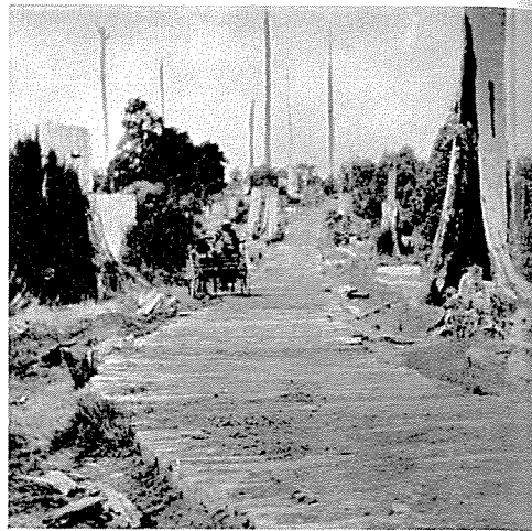
Corduroy construction on Beech Forest-Lavers Hill Road, 1913.
