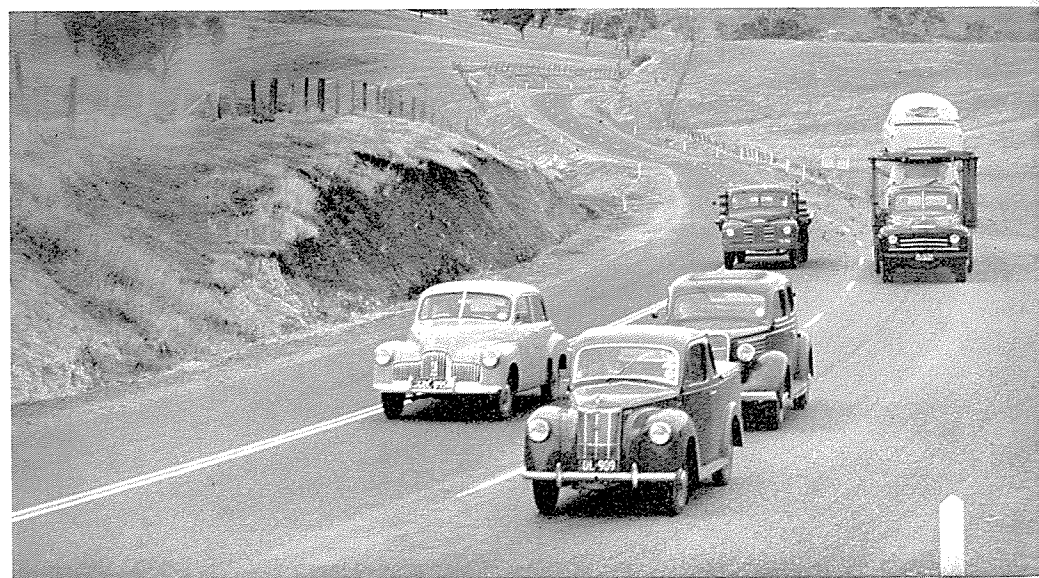
Additional climbing lane for slow-moving traffic, Western Highway, west of Bacchus Marsh, constructed 1955-56.
