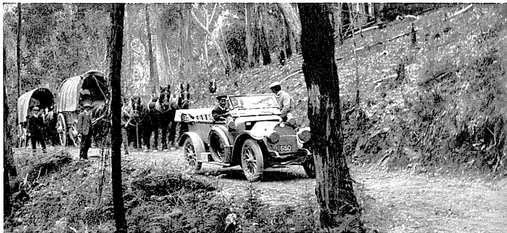
Insolvent track—Dargo Road. C.R.B. inspection, 1913.
