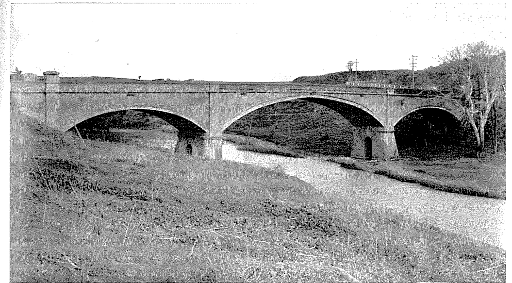
Concrete arch bridge over the Moorabool River at Fyansford; constructed 1899/1900.
