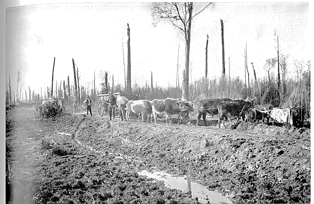
Road works in progress, Woorayl Shire, in the early 1900's.
