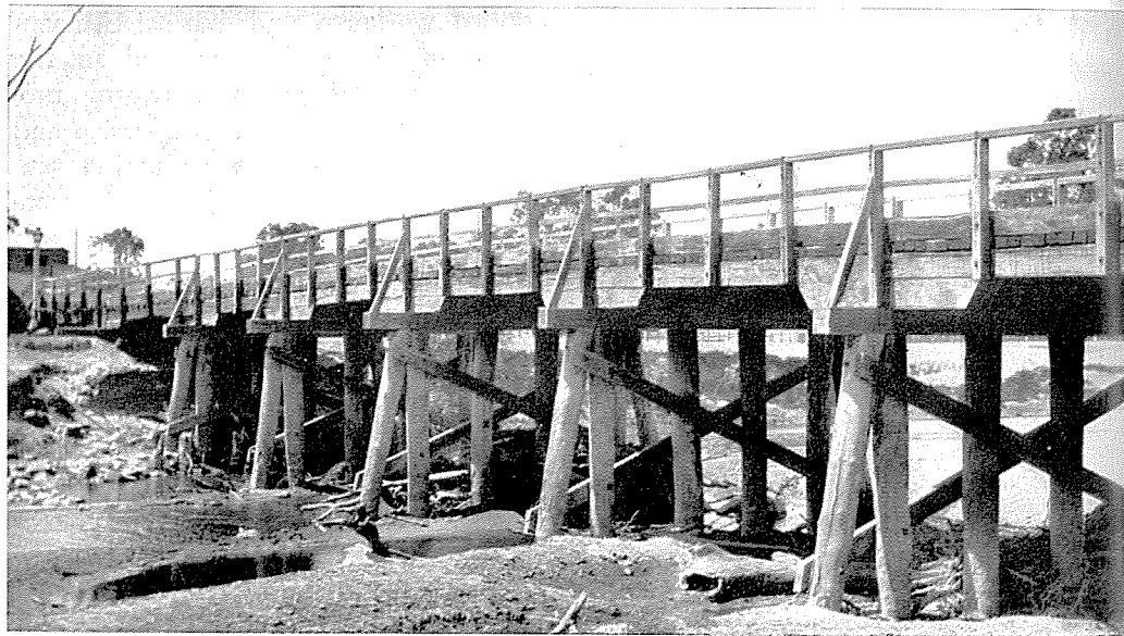
Typical timber bridge in existence, 1913.
