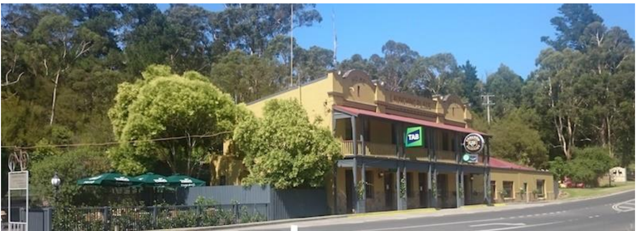
Launching Place. The proposed deviation would have been in the hills behind the Pub.
