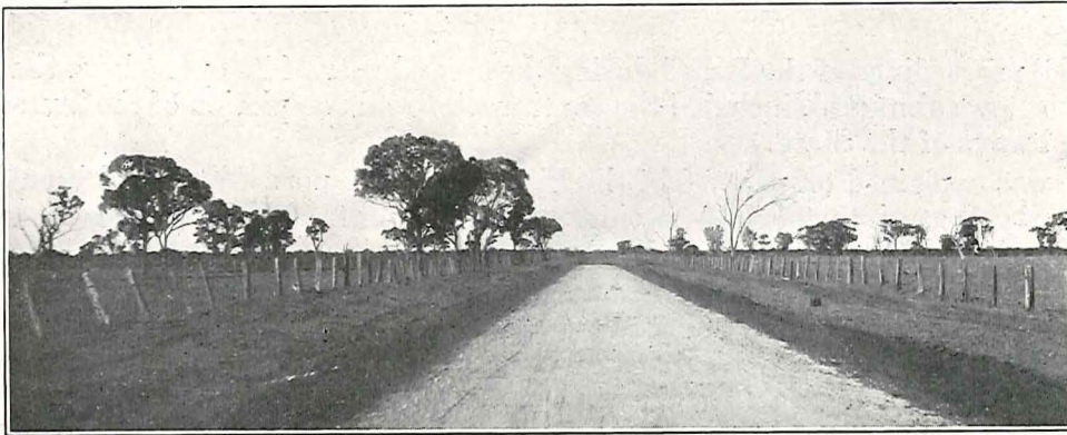
Plate 1. Limestone Road—Shire of Lawloit.
