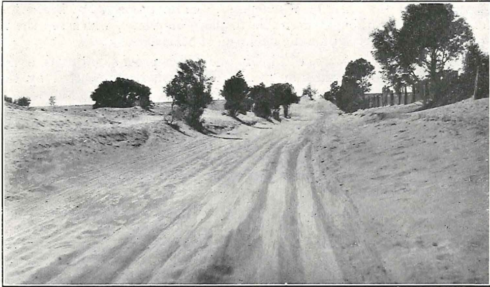
Plate 2. Showing sand drifts in cutting.
