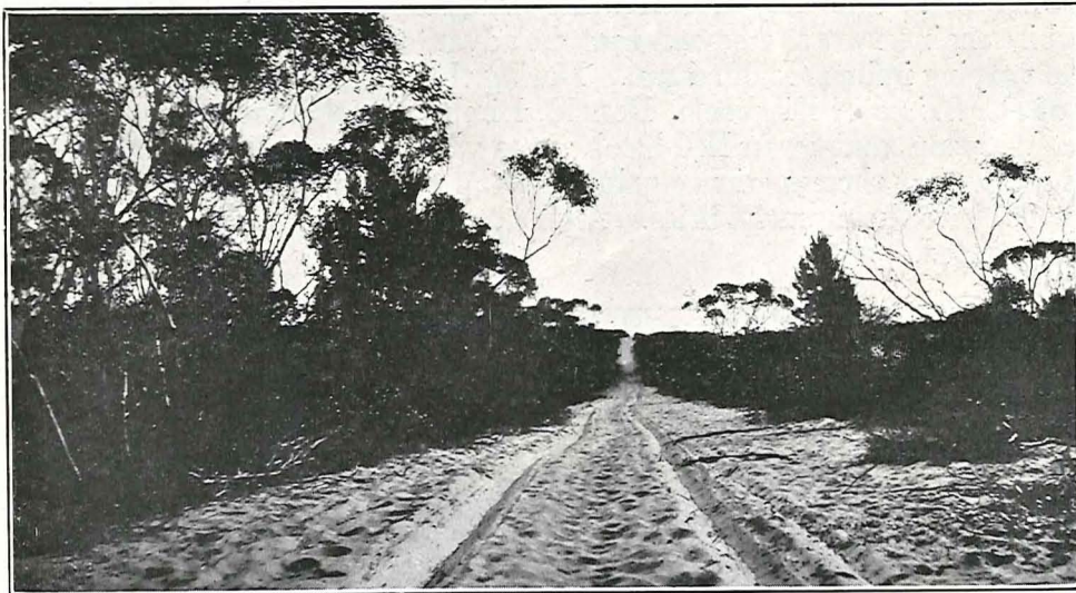
Plate 4. Loose sand on Sea Lake-Ouyen Road.
