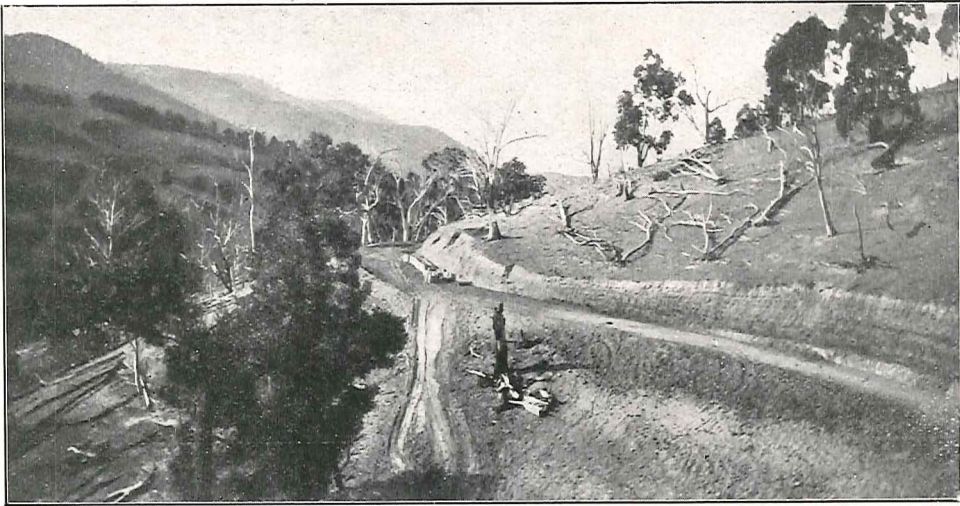
Plate 27. Showing graded deviation in progress, Omeo Shire.
