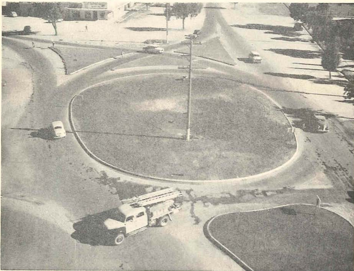
Plate 26.—Murray Valley Highway, Section 2. Channelized intersection at Beechworth-Wodonga Road.
