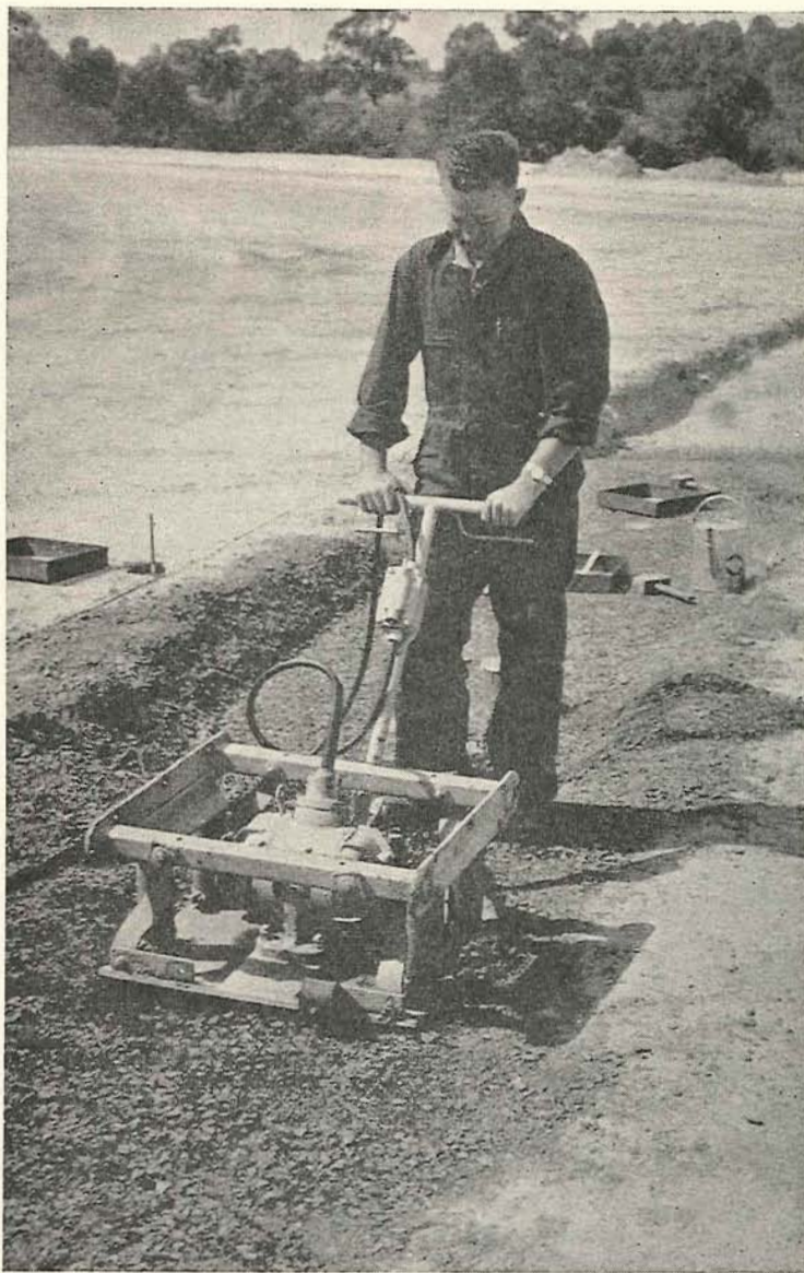
Plate 3.—“ Jackson ” multiple plate compactor showing one plate used separately.
