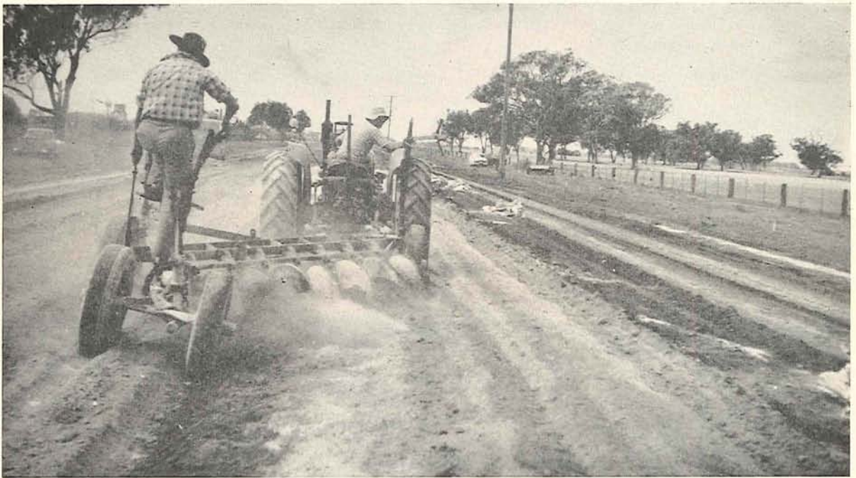
Plate 28.—Mixing "Limil" and soil by disc harrow.
