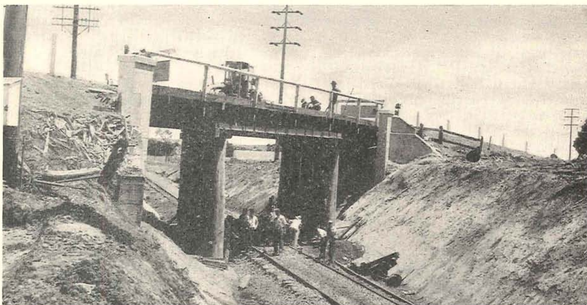
Plate 20.—Shire of Winchelsea. Princes Highway West, Section 2. Temporary replacement of bridge over railway at Armytage.
