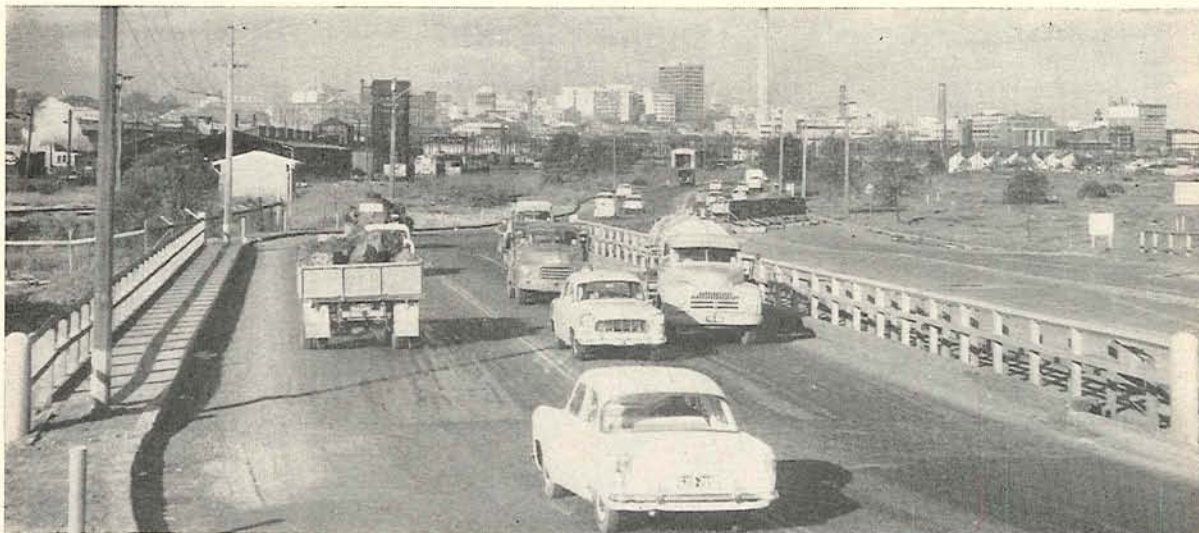
Plate 40.—City of Melbourne. New temporary bridge over Coal Canal on New Footscray Road.
