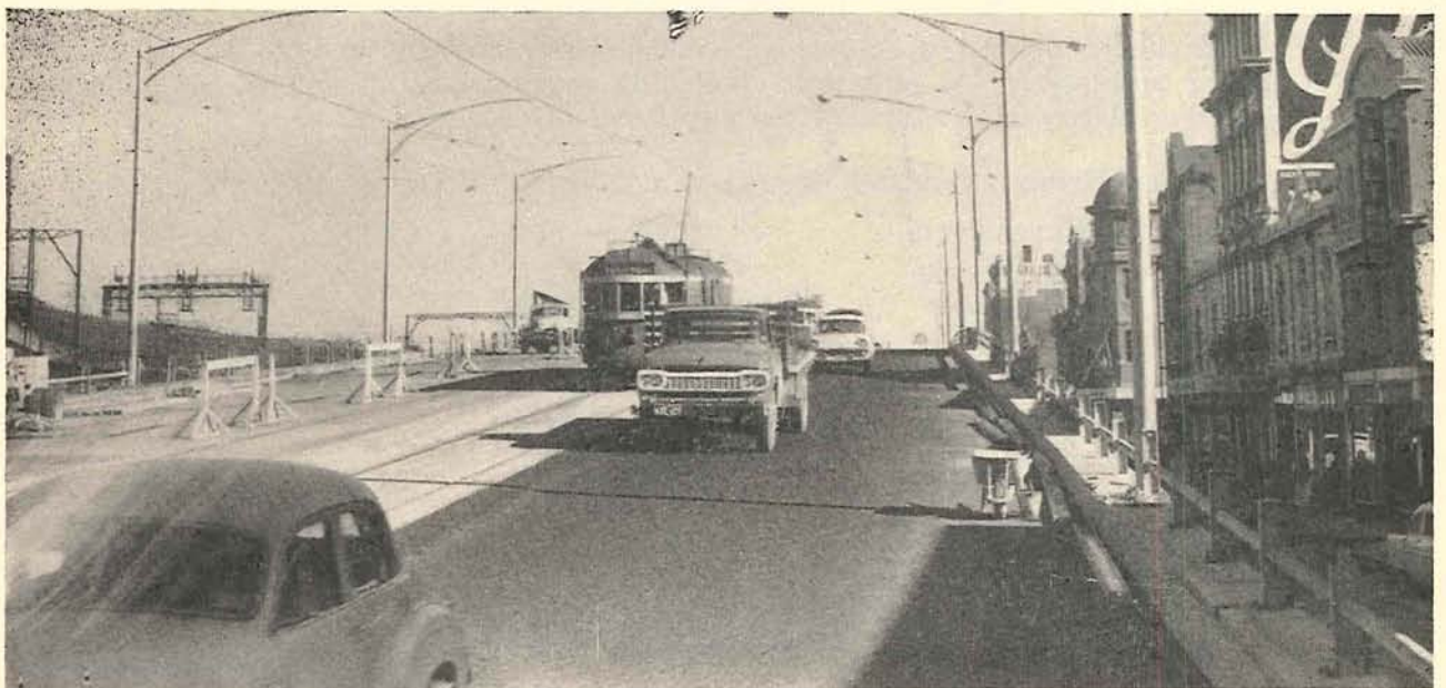
Plate 38.—King Street Bridge. City of Melbourne. Showing traffic using half of overpass in Flinders Street, late July, 1960.
