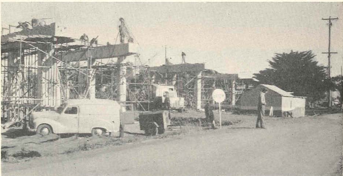
Plate 32.—Duncan's Road Overpass in course of construction.
