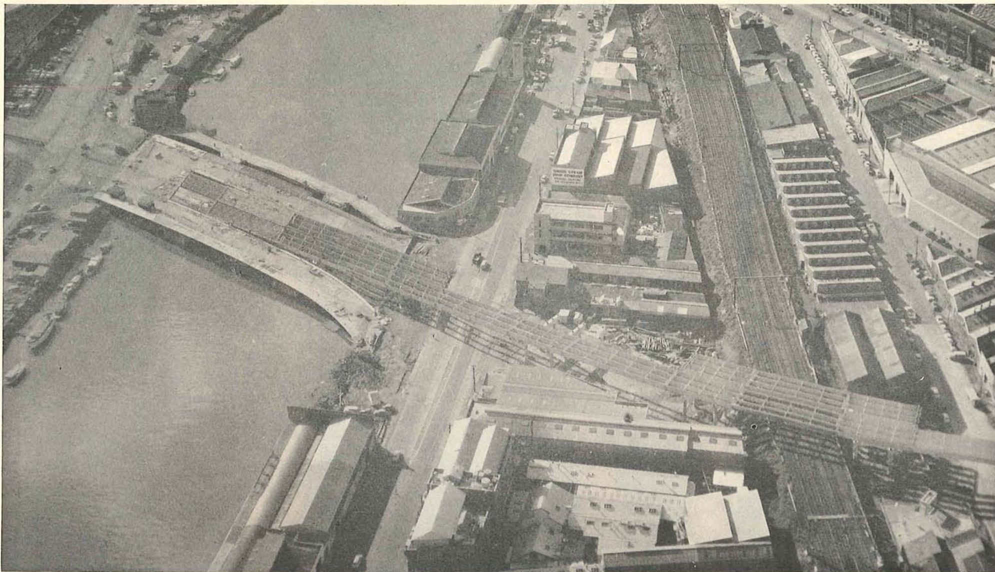
Plate 39.—King Street Bridge, showing almost completed Yarra River span and girders in place over Port Melbourne-St. Kilda railway on right.
