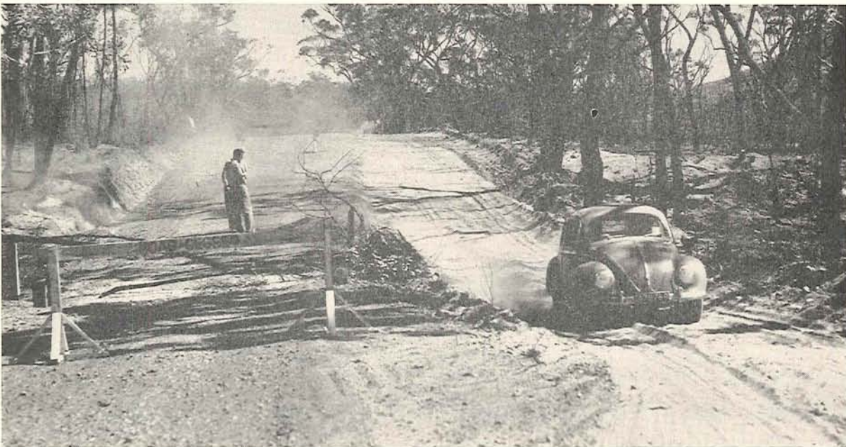
Plate 12.—Shire of Ararat. Grampians Road near Jimmy's Creek. Side track around a timber culvert burnt out by bush fire.
