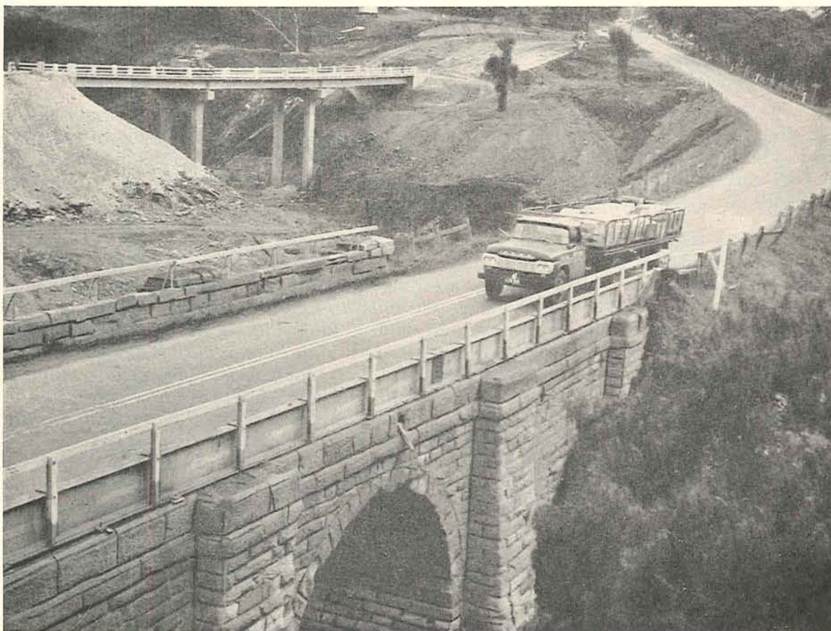
Plate 22.—Shires of Melton and Bacchus Marsh. Western Highway, Section I. Bridge on new alignment over Djerriwarrh Creek with old narrow bridge in foreground.
