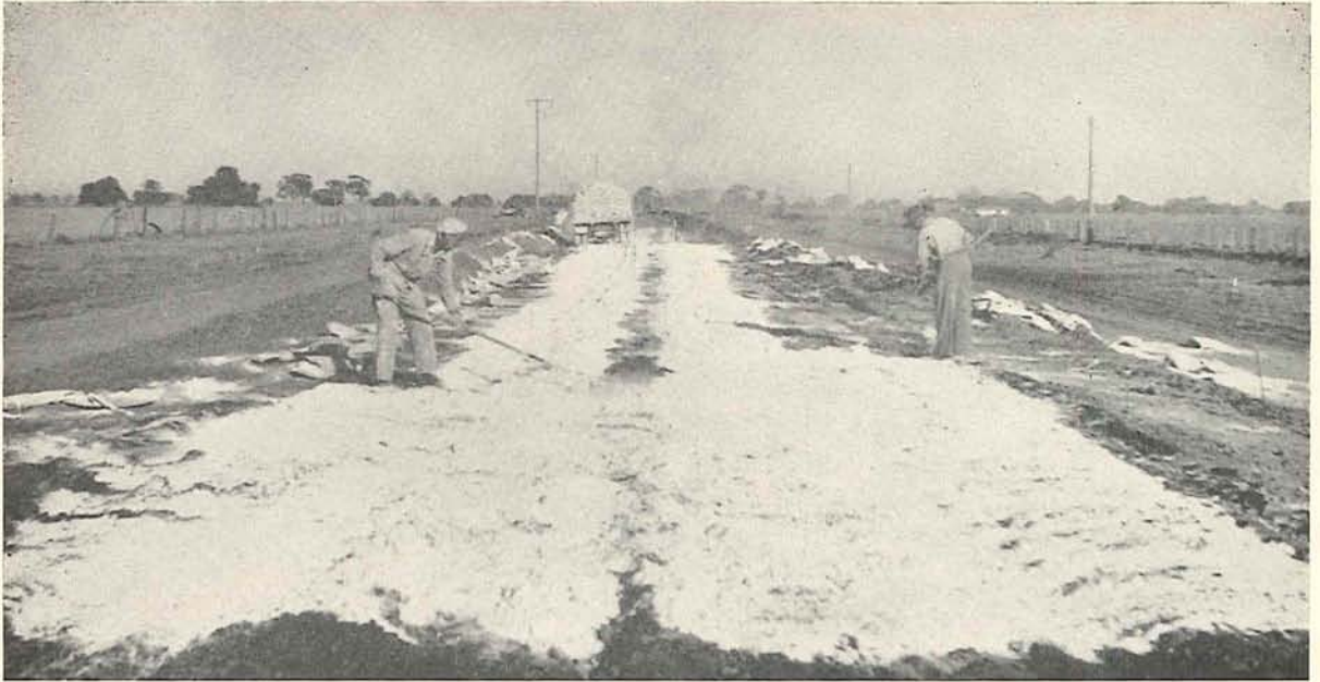
Plate 27.—Spreading "Limil" on loose soil.
