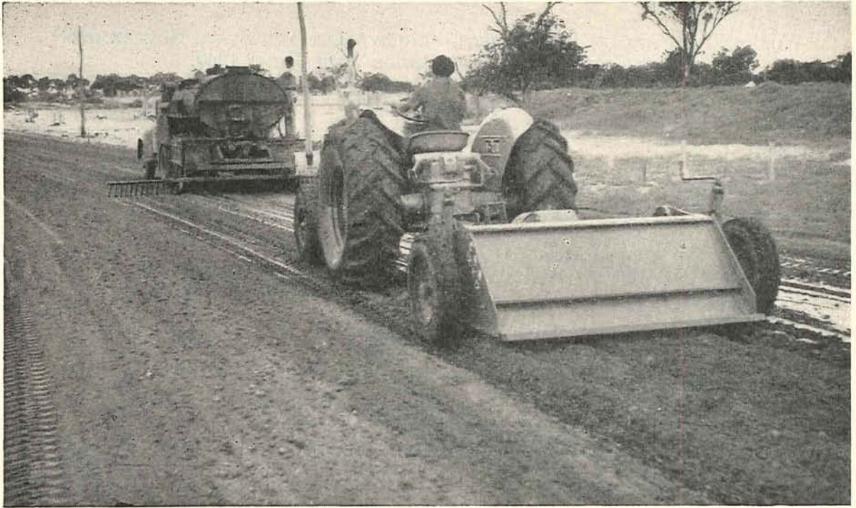
Plate 45.—Borong Highway, mileage 24. At Donald. Bituminous emulsion stabilizing, showing sprayer and tractor with attached rotary hoe.
