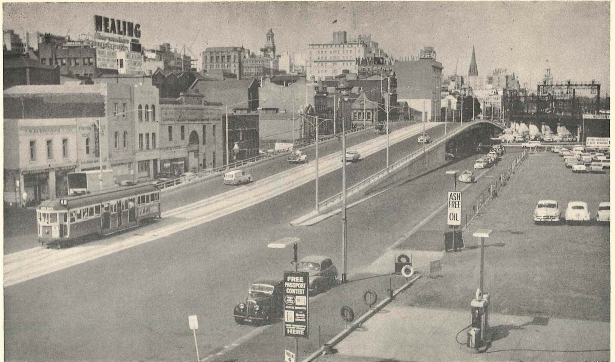
FRONTISPIECE: Overpass in Flinders-street—Portion of Kings Bridge Project.
