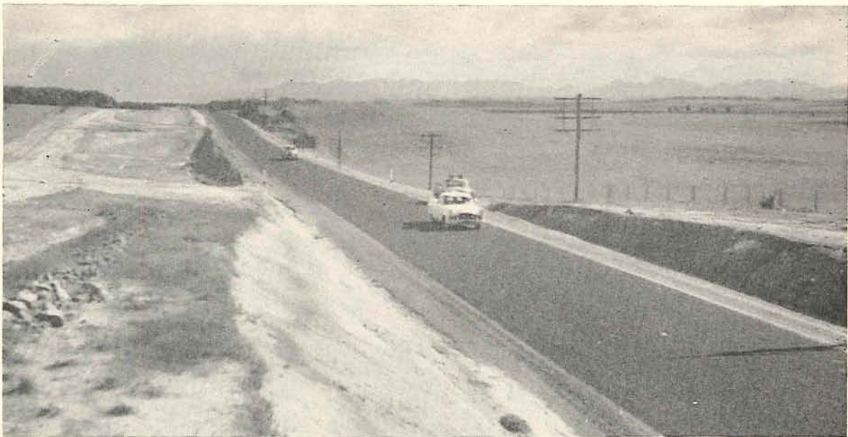
Plate 31.—Glenelg Highway. Approximately 146 miles east of Glenhompson, after realignment, reconstruction and sealing.
