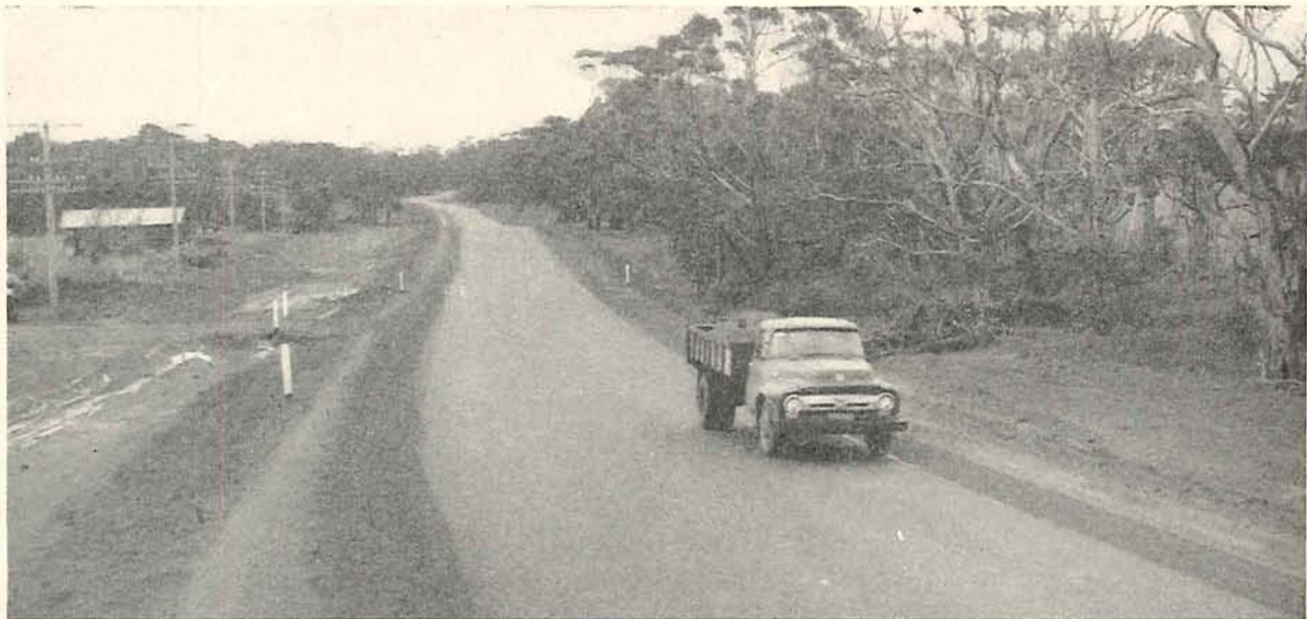
Plate 30.—Henty Highway, Section I. Reconstruction, widening and sealing completed on a section north of Portland.
