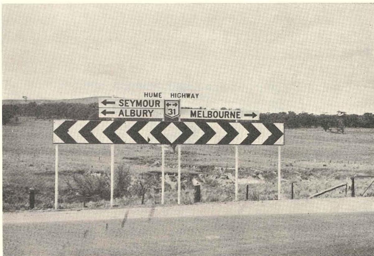
Plate 5.—Hazard marker providing directional information with horizontally pointed chevrons.
