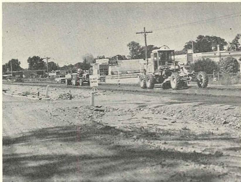
Plate 11.—Hume Highway—Construction of the approaches to the new bridges over the Ovens River at Wangaratta.
