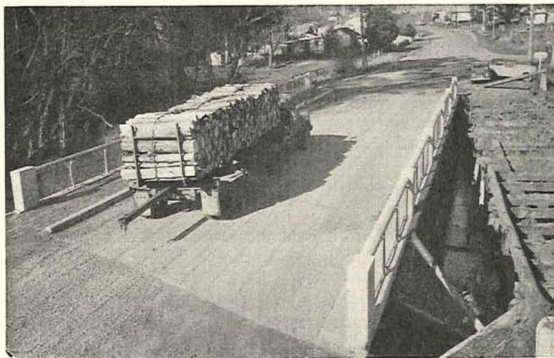
Plate 42.—Shire of Buln Buln—Four-span concrete bridge over the Latrobe River on the Loch Valley Road Noojee.
