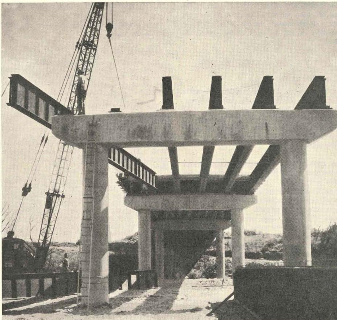
Plate 4.—Construction of Avon River Bridge at Stratford.
