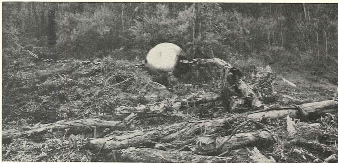
Plate 44.—Shire of Heytesbury—Clearing scrub near Coradjil with Ball and Chain.
