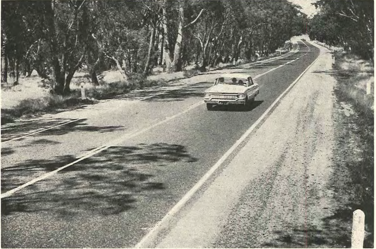
Plate 31.—Edge lining on the Calder Highway in the Black Forest area—Shire of Gisborne.
