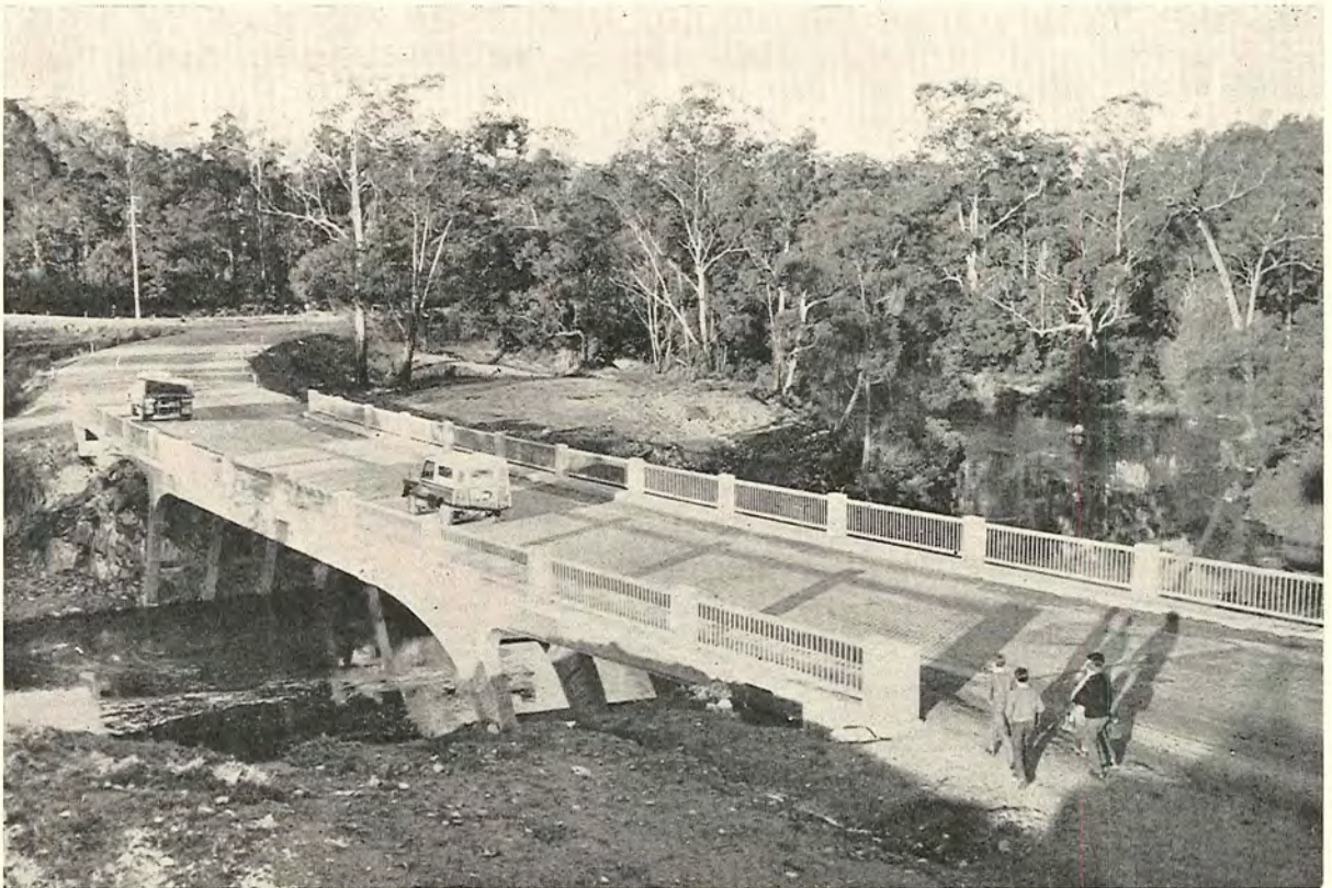
Plate 30.—New steel framed bridge with reinforced concrete deck over Boggy Creek at Nowa Nowa—Princes Highway East.
