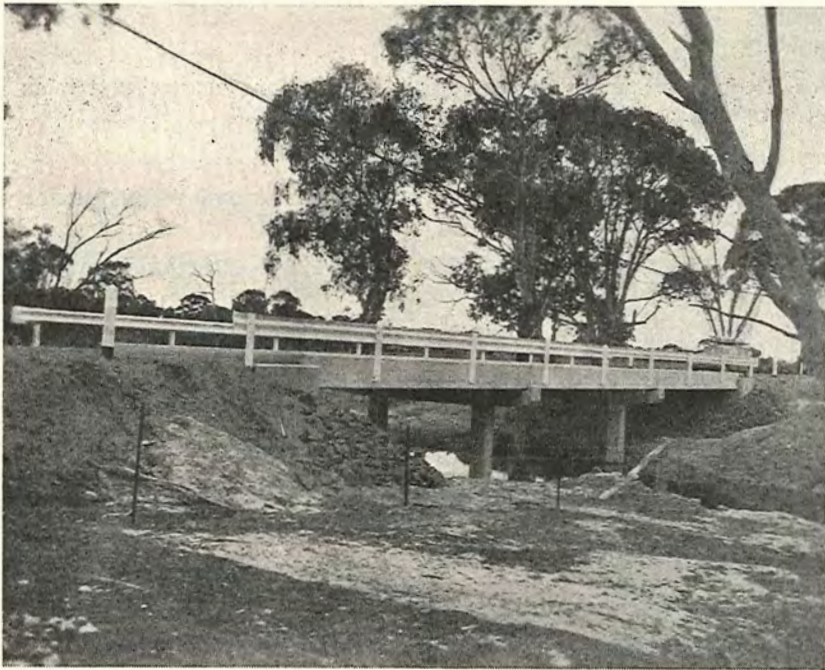
Plate 40.—Evans Bridge on Carapooee Creek on Carapooee Road—Shire of Kara Kara.
