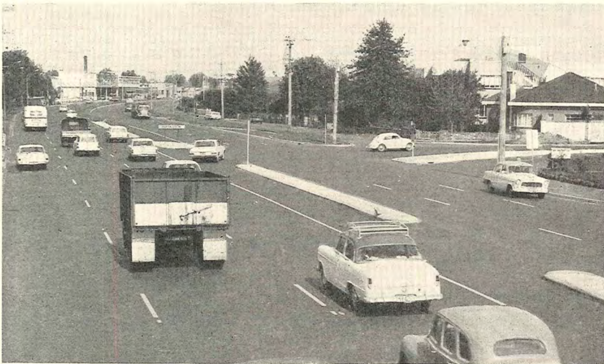
Plate 12.—New six-lane pavement on the Heidelberg-Eltham Road—City of Northcote.
