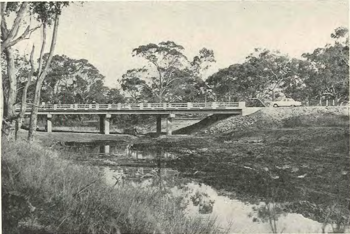
Plate 17.—The Lady Somers Bridge over Mount William Creek—The Halls Gap Road—Shire of Ararat.
