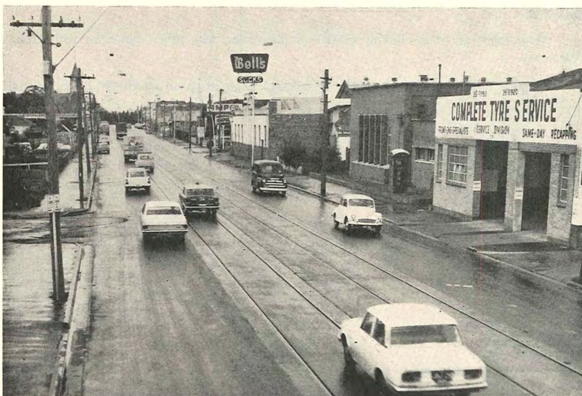
Plate 13.—Sydney Road. The reconstructed section north of Bell Street—City of Coburg.
