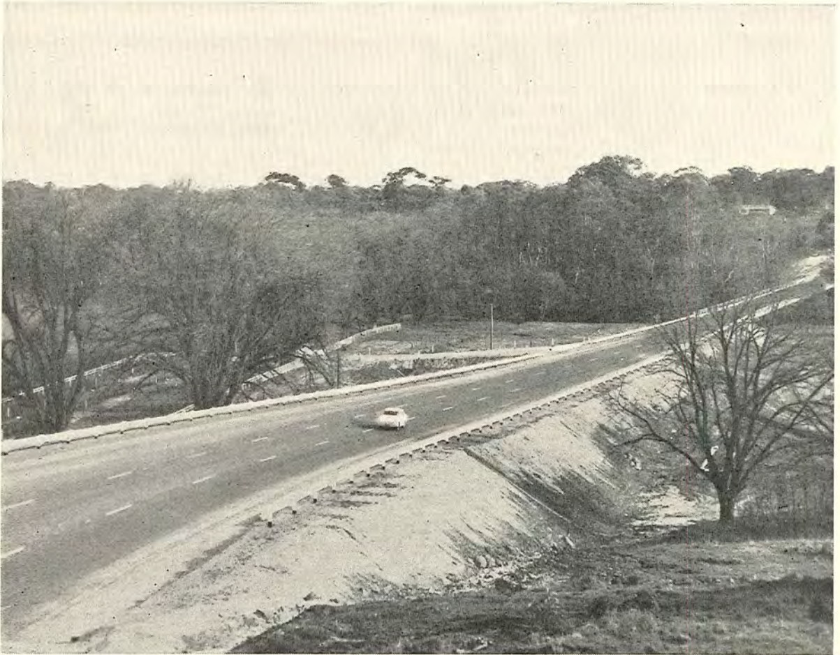
Plate 33.—Approach to new bridge over the Campaspe River at Axedale—Shire of Strathfieldsaye.
