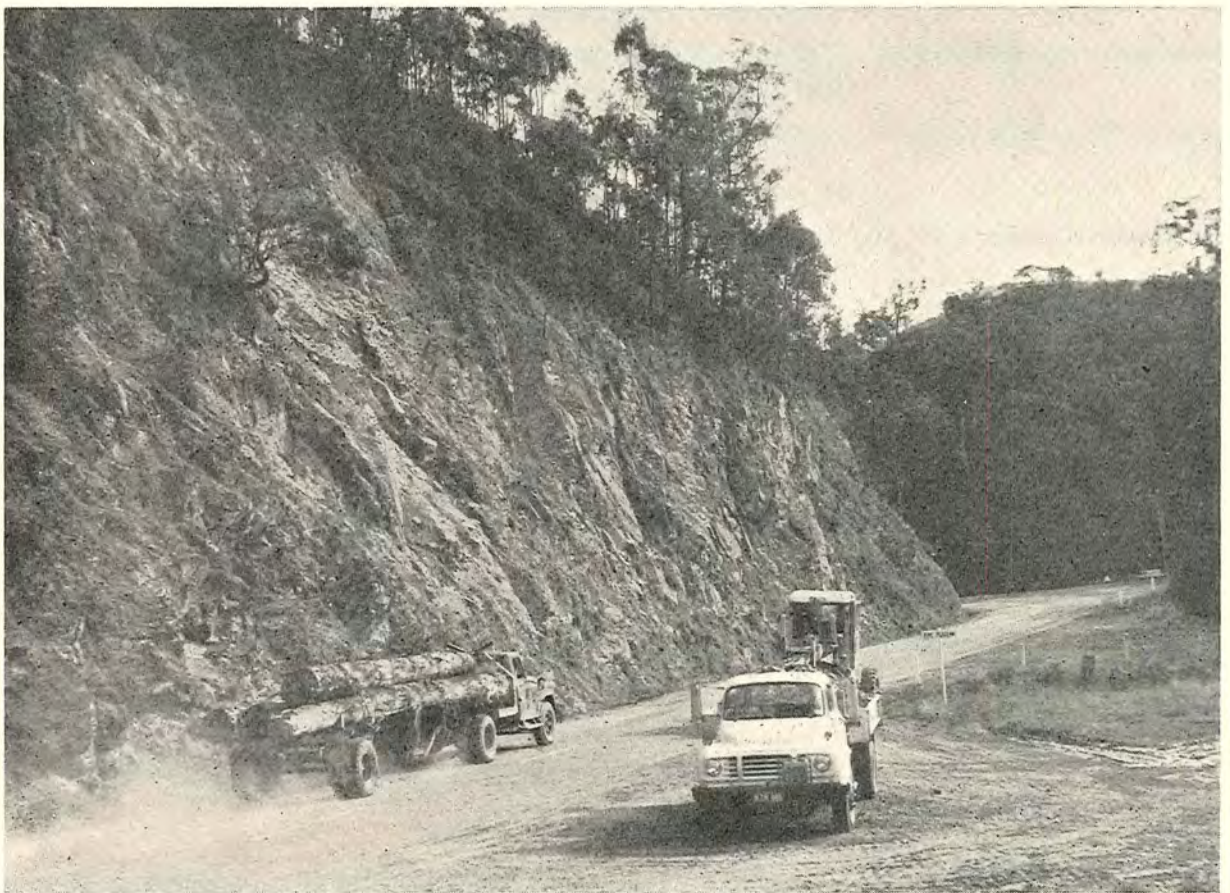
Plate 37.—Work under cutting—Warburton—Woods Point Road—Shire of Upper Yarra.
