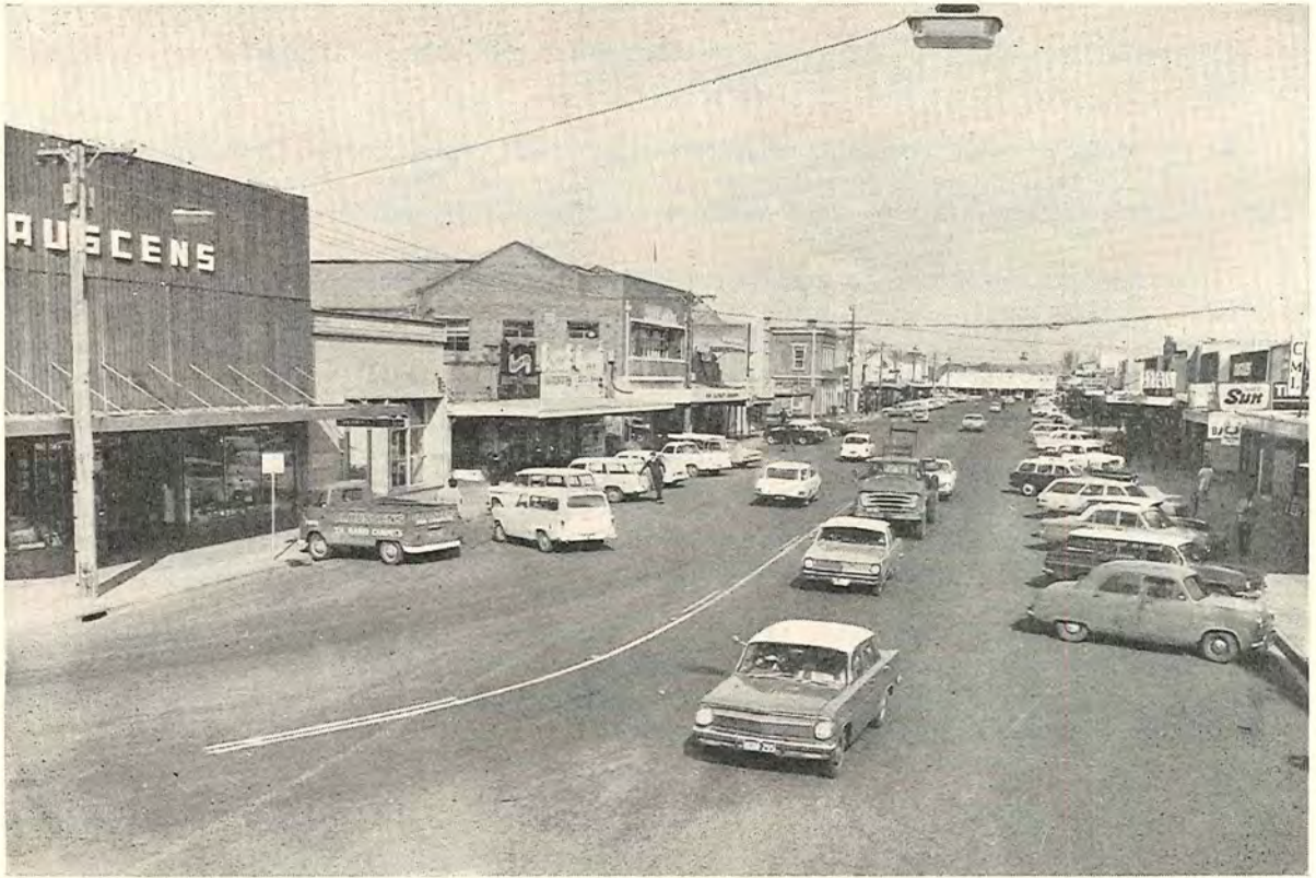
Plate 29.—Princes Highway East—Reconstructed section in the City of Traralgon.
