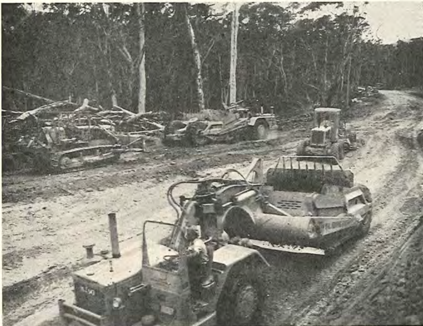
Plate 27.—Roadworks in progress on the Grampians Road—Lake Bellfield deviation.
