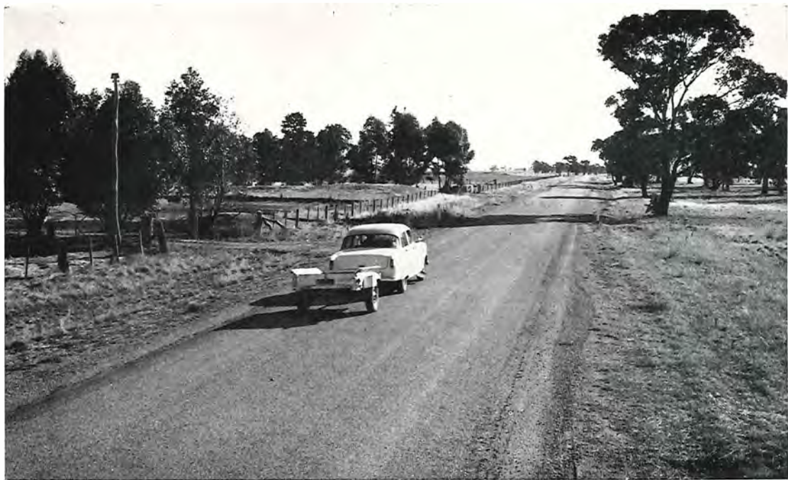
Charlton Road—Kara Kara Shire—Reconstructed section.
