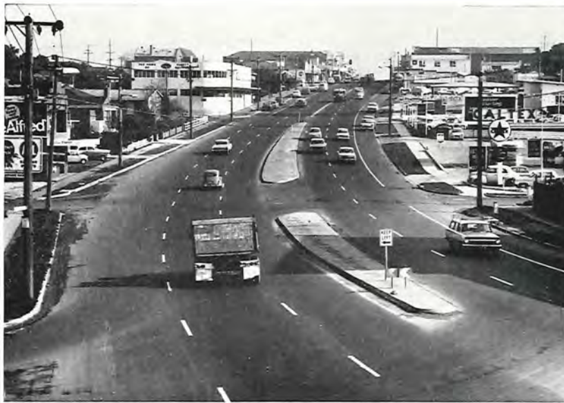
Burwood Highway—Dual carriageways east of Warrigal Road—City of Box Hill.
