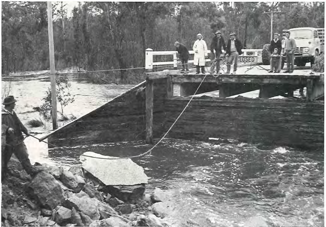
Princes Highway East—Washed away approach at the Reedy Creek Bridge—Orbost Shire.
