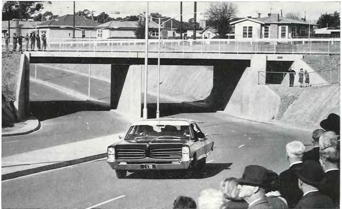
The Minister of Public Works, the Hon. M. V. Porter, M.L.A., becomes the first official traveller to use the Tuaggra Street underpass in Maryborough City. The opening ceremony was attended by the Chairman and Member of the Board, the Mayor of Maryborough and other invited guests.
