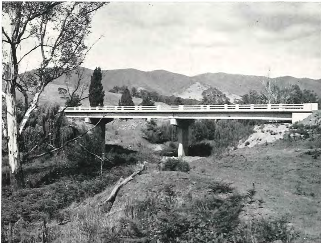
New bridge on Ramrod Flat Road over the Tambo River—Shire of Tambo.
