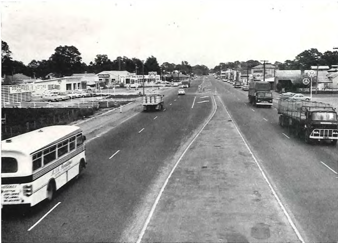
Hume Highway—Four lane dual carriageways in Seymour township.
