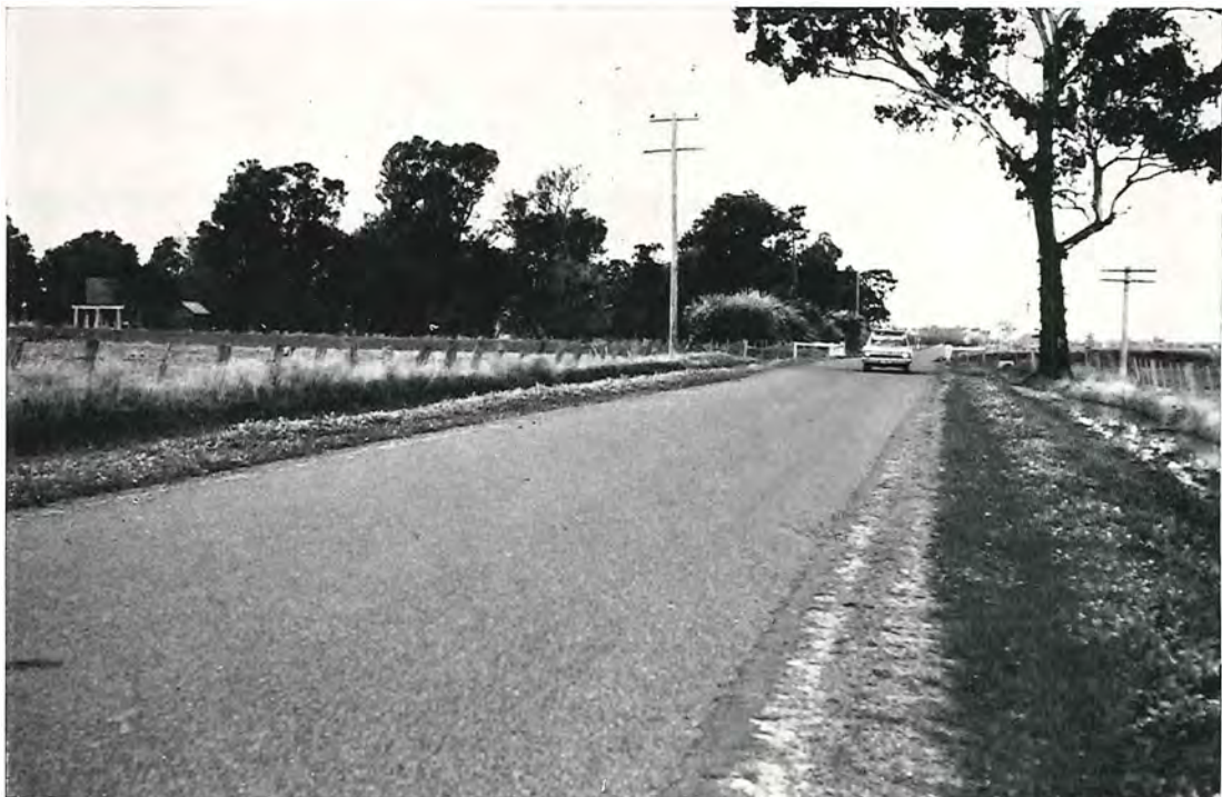
Baulkamaugh Hall Road—Strengthened and sealed to a width of 18 feet.
