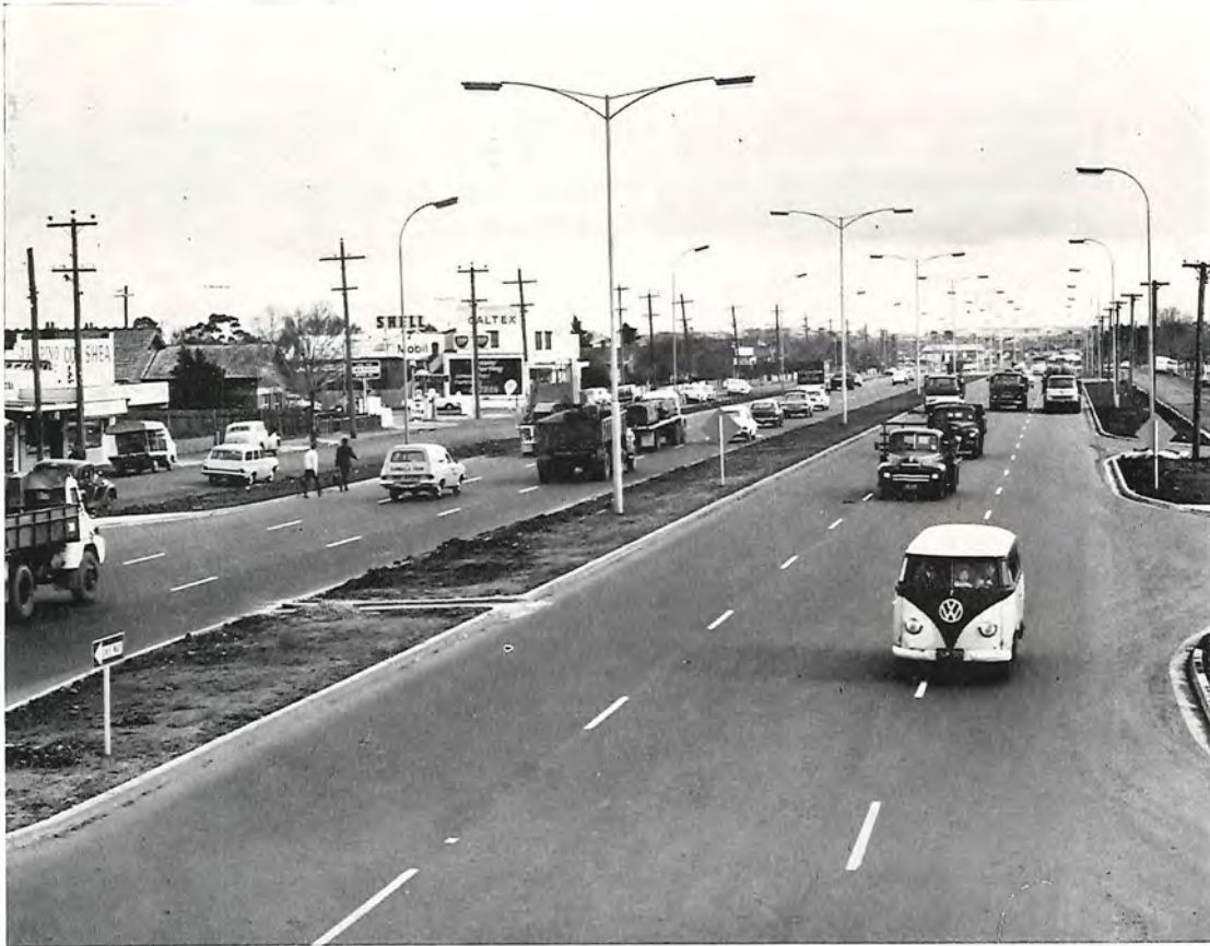
Princes Highway West—Dual carriageways between Robbs Road and Somerville Road—Footscray City.
