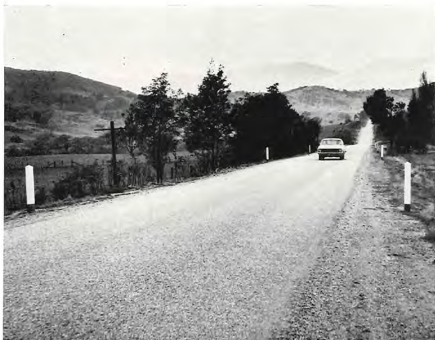
Dederang Road—Yackandandah Shire—Reconstructed section.
