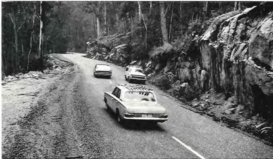
Mount Buffalo Road—A "freeze-thaw" resistant pavement at road level 4000 feet.
