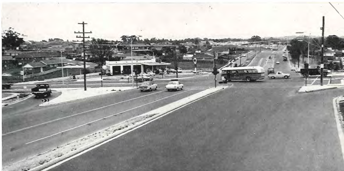
Dual carriageways and intersection treatment at the junction of Canterbury Road and Springvale Road —Nunawading City.
