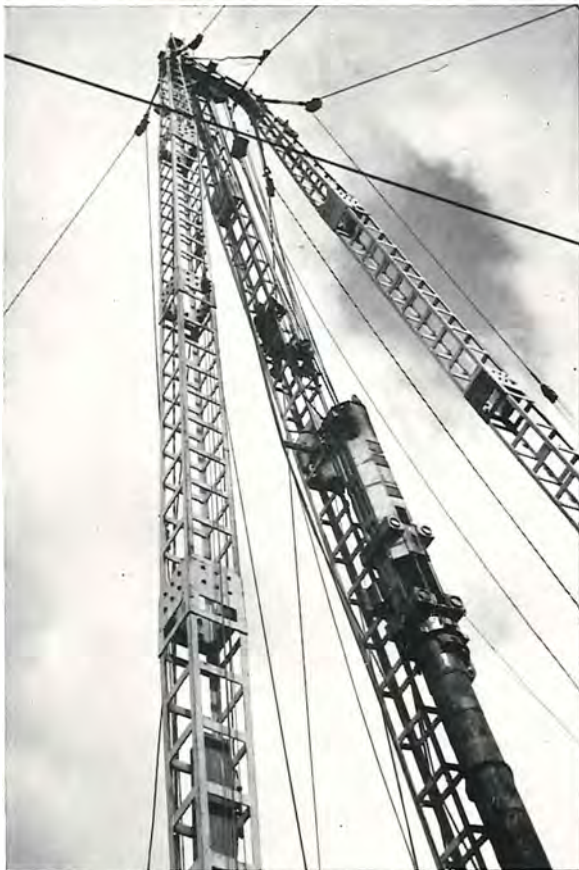
Plate 2—Maribyrnong River Bridge, Raleigh's Road. Pile driving in progress.
