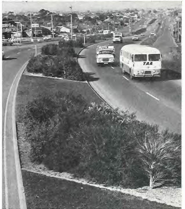
Calder Highway—Shrubs planted in the narrow median reduce headlamp glare and risk of cross median accident.
