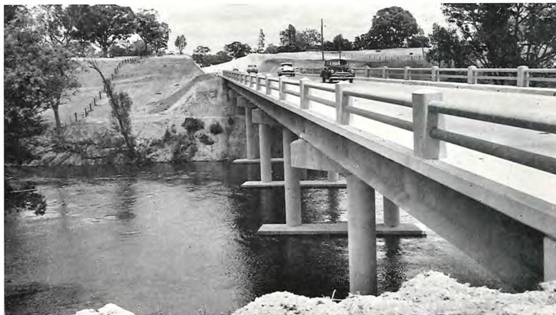
Hume Highway—New Bridge over the Goulburn River on the approach to Seymour.
