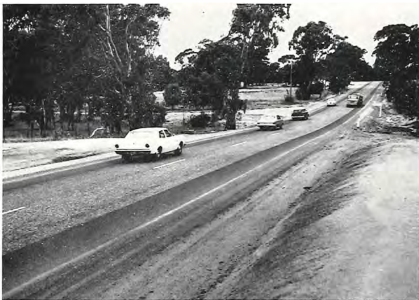
Calder Highway, Marong Shire—Widening to 24 feet sealed width on strengthened shoulders.
