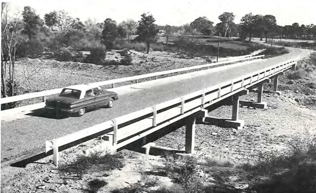
Delta Bridge over Valencia Creek, Briagalong Road—Shire of Maffra.
