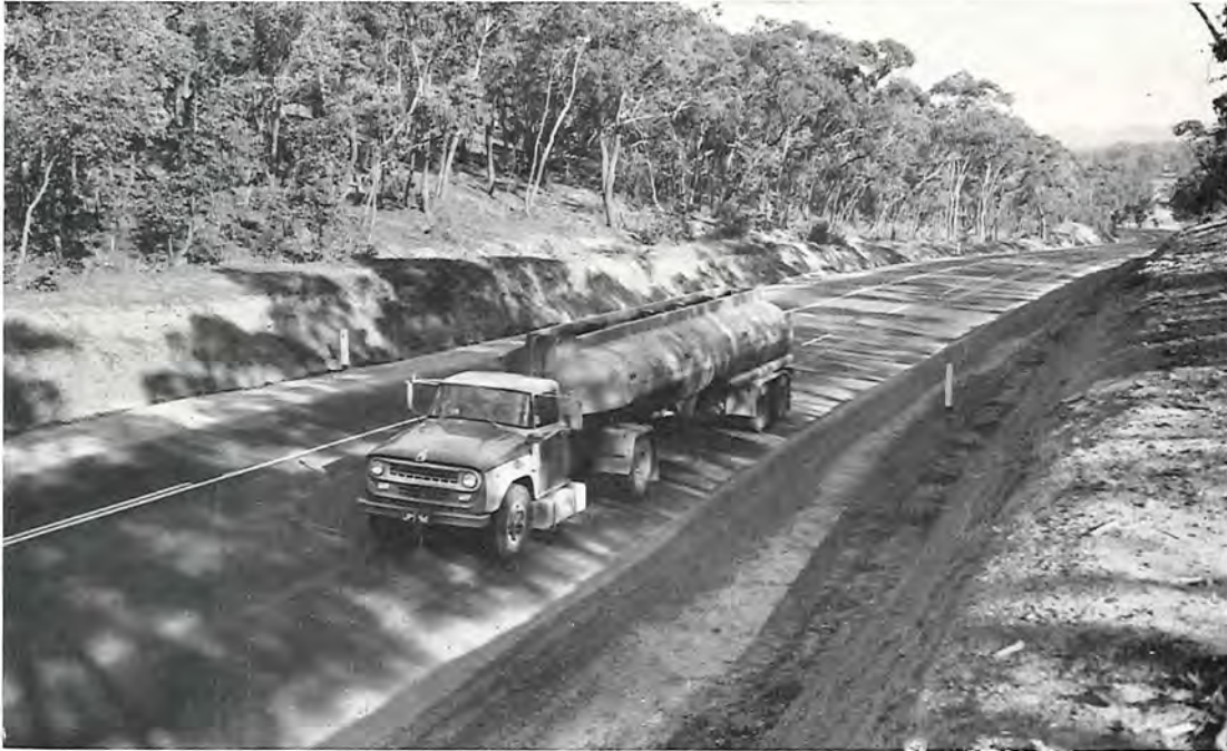
Calder Highway—Reconstruction with an additional climbing lane at Taradale.
