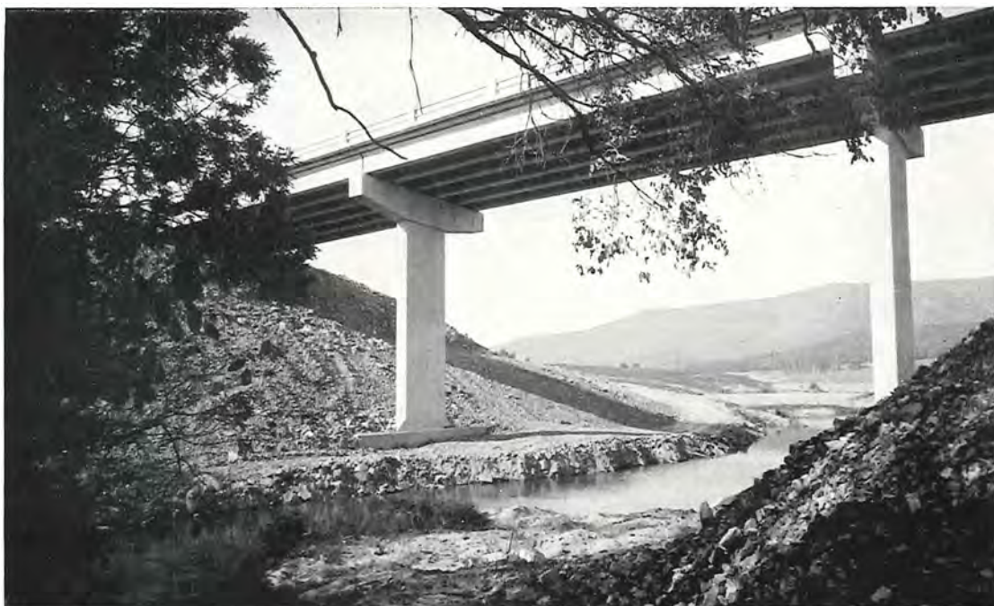
Three span reinforced concrete bridge over Sandy Creek on the Nillahcootie deviation.
