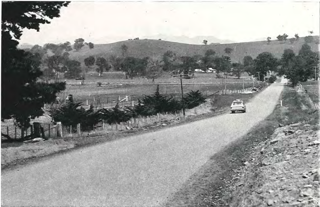
Olivers Lane—Mansfield Shire—Reconstructed section.
