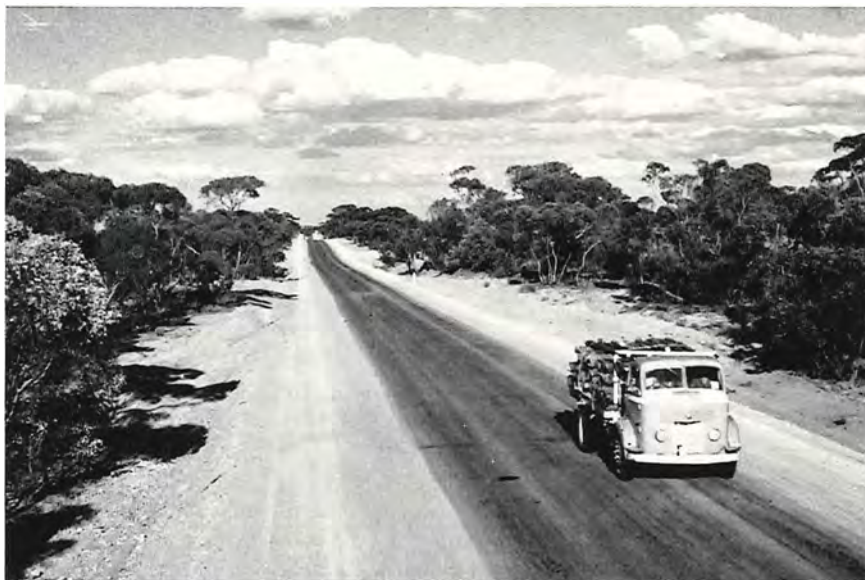
Robinvale Road—Reconstructed section 20 feet wide—Shire of Swan Hill.
