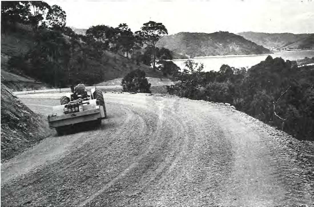
Work is progress on the approach to the Frazer National Park—Lake Eildon in the background.
