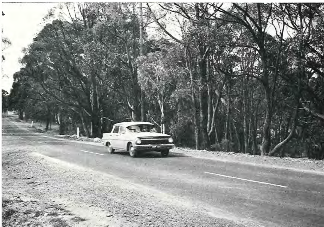
Ballan Road—Daylesford and Glenlyon Shire, reconstructed section.
