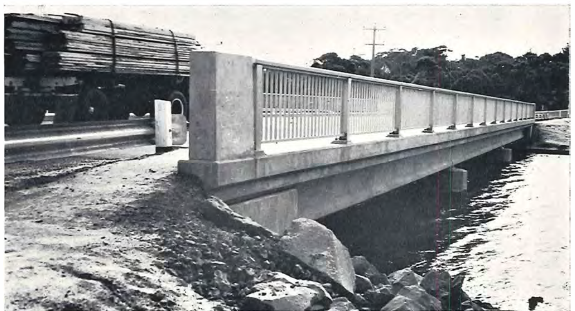
Anglesea River Bridge — Ocean Road, Barrabool.
