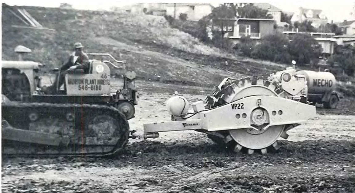
Ten ton Vibrating Tamping Roller in use at Strathmore.
