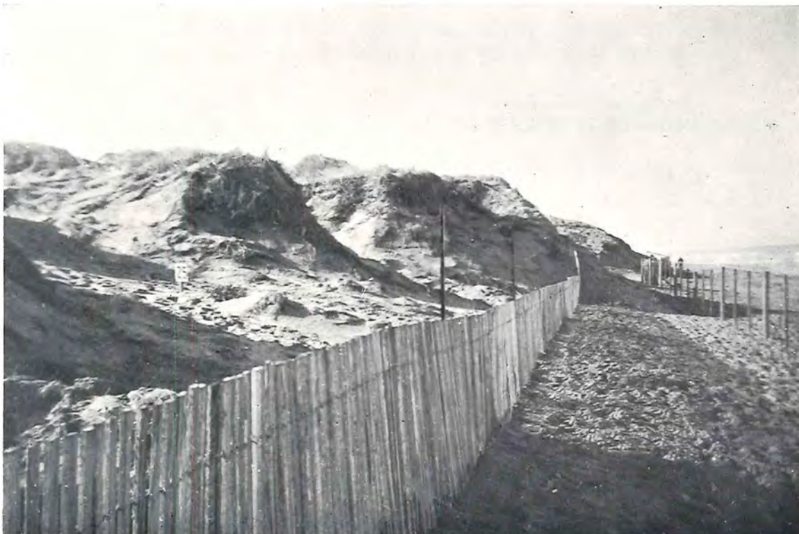
Plate 5 — Sand Drift Control. Slat Fence Erected Across Gully Entrance.
