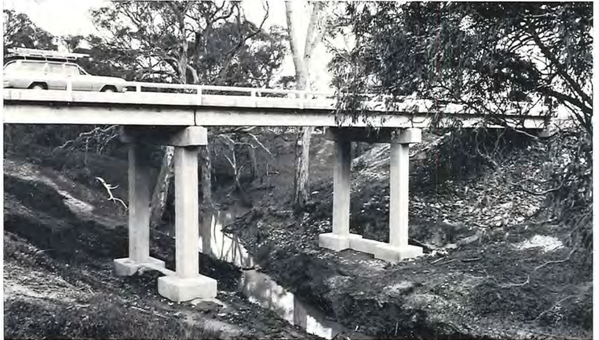
McIntyres Road — Construction of Langdon's Bridge — Kara Kara Shire.
