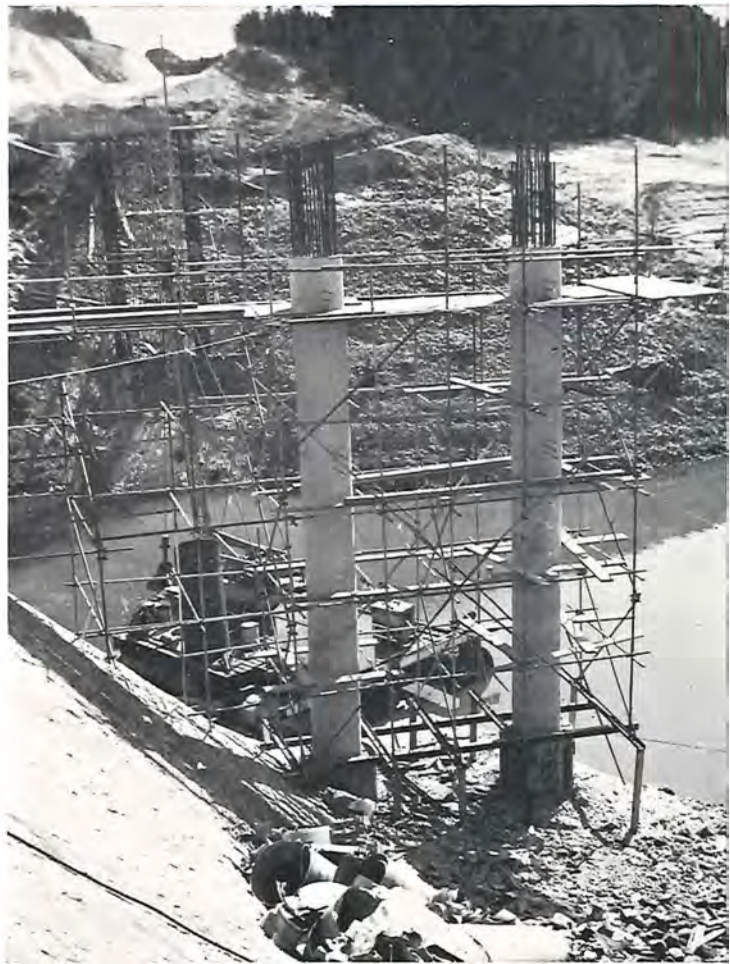
Plate 7 — Pykes Creek Reservoir Bridges Duplication. Outer Main Piers Under Construction.
