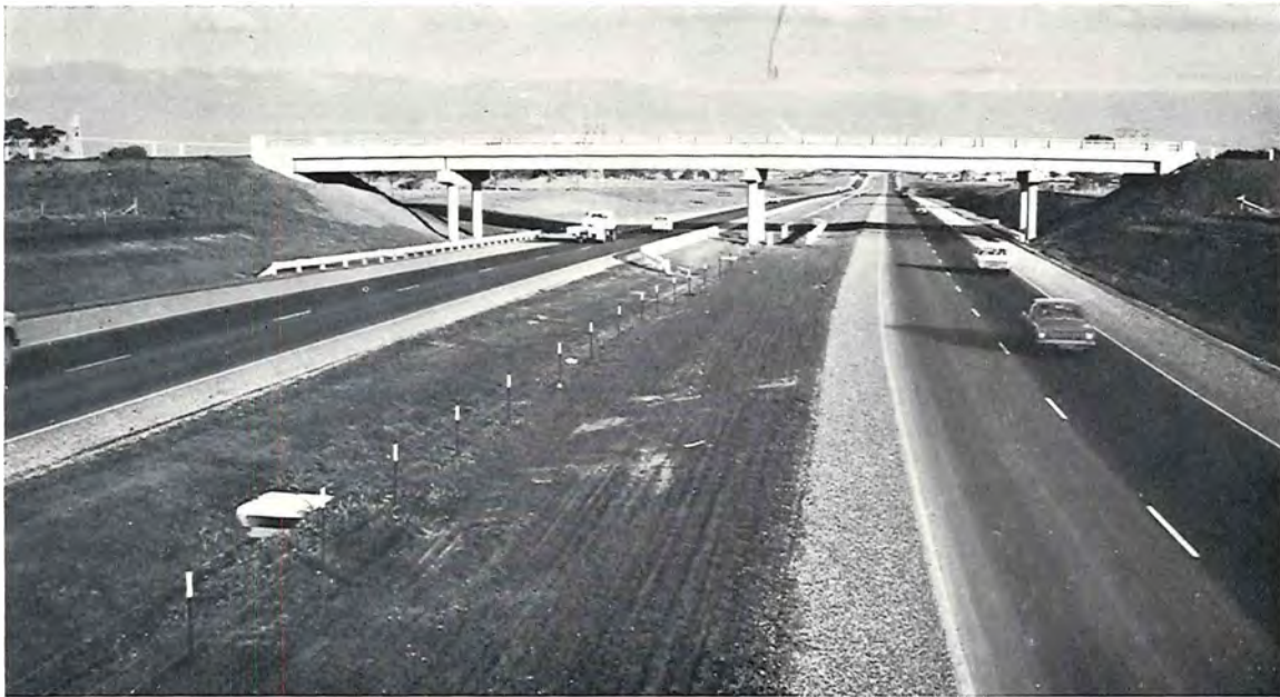
Tullamarine Freeway — View under Carrick Drive Overpass.
