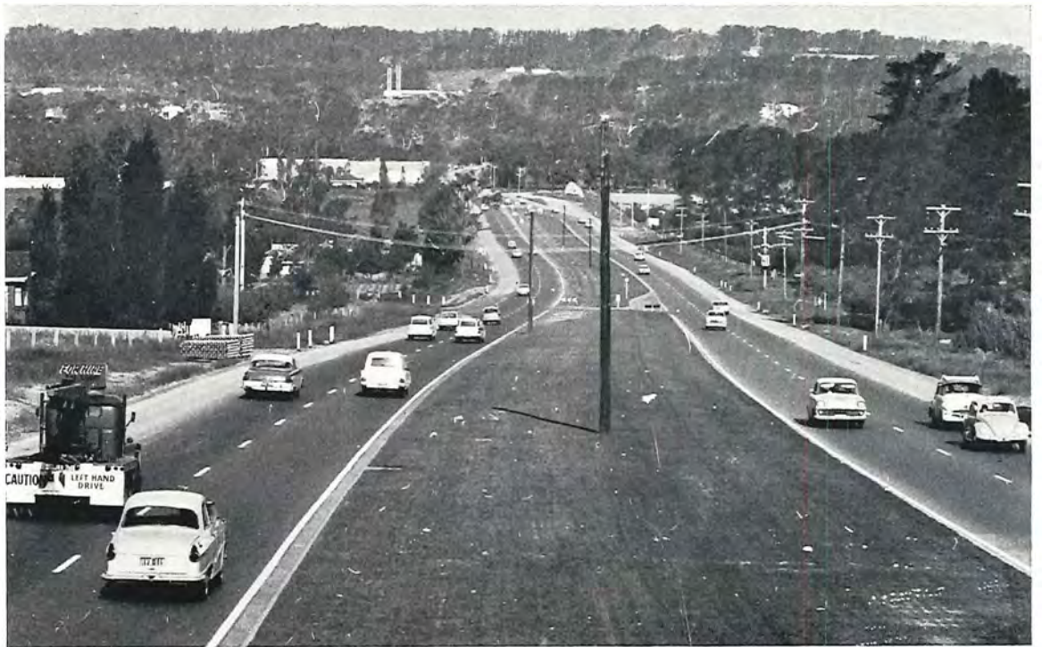
Burwood Highway — Dual carriageways between Springvale Road and Dandenong Creek.
