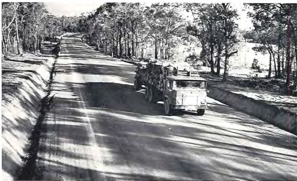
Midland Highway — Reconstructed section south of Yinnar.
