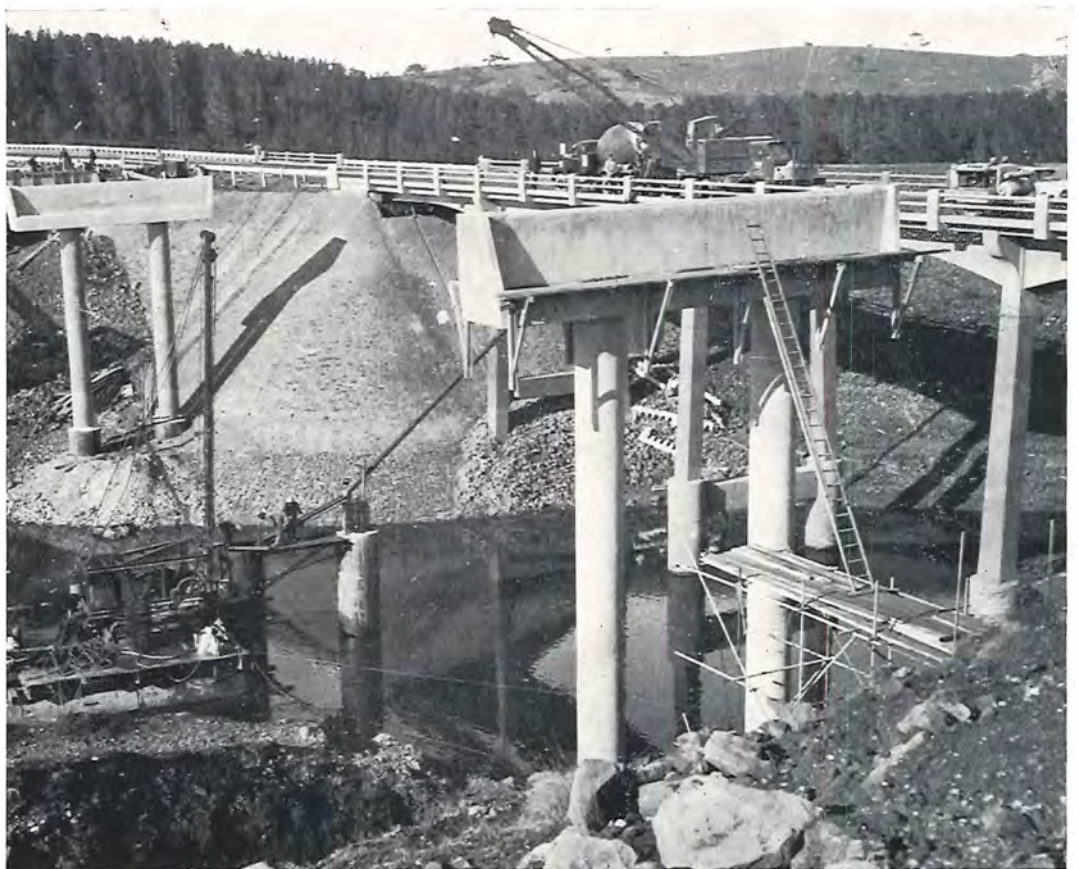
Plate 8 — Pykes Creek Reservoir Bridges Duplication. Central Main Pier Under Construction.
