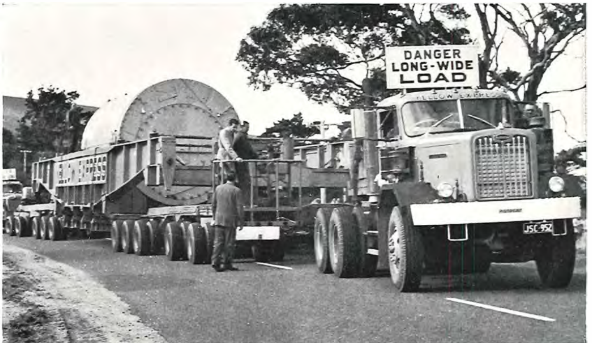
163 ton Stator en route to Anglesea Power Station.
