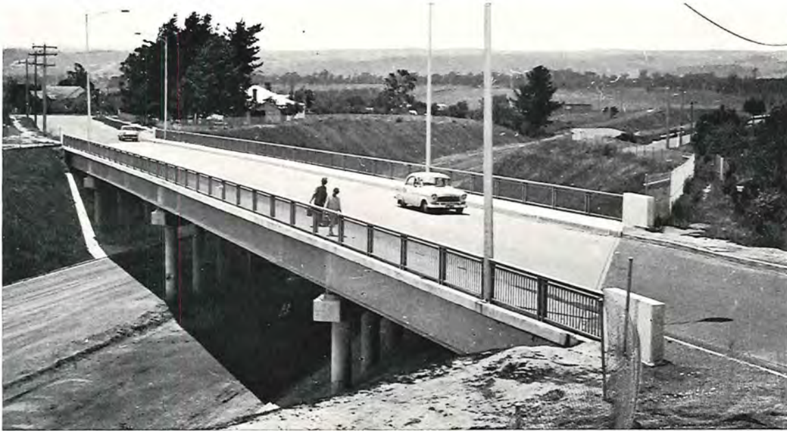
Princes By-pass Road (Moe Section) — Coalville Road Bridge.
