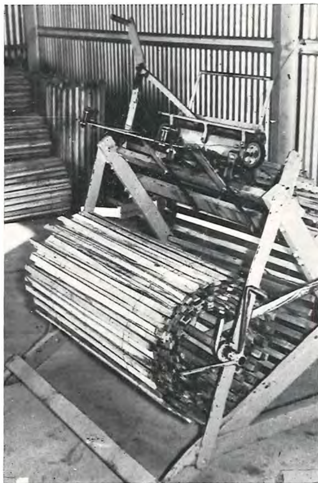
Plate 4 — Sand Drift Control. Machine Designed by Soil Conservation Authority for Production of Slat Fencing.
