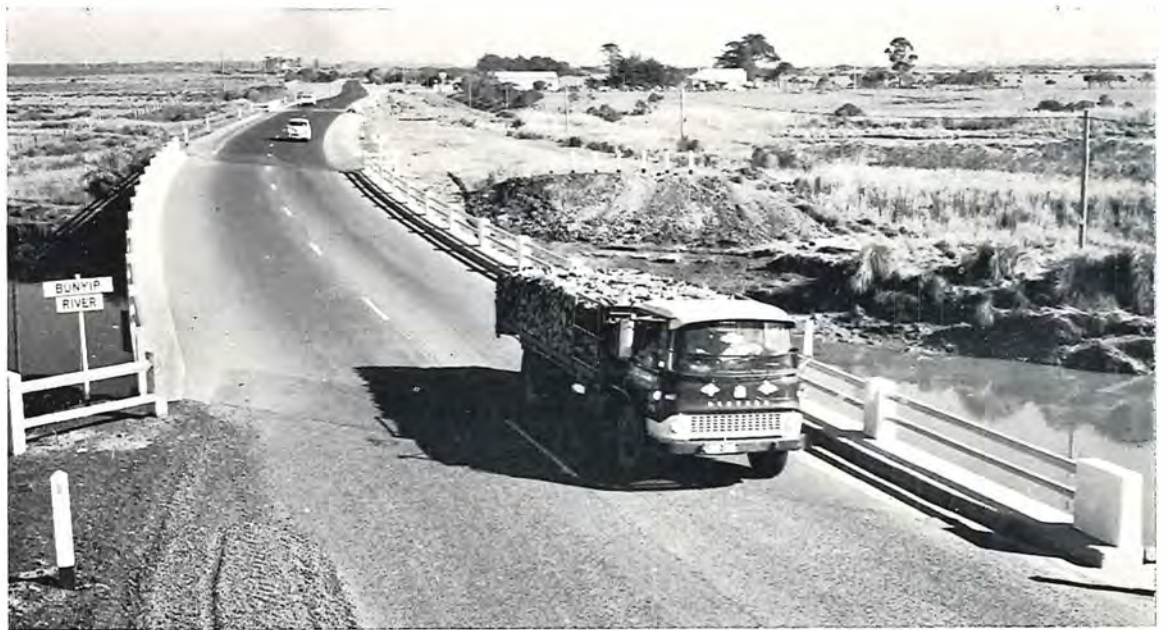
South Gippsland Highway — New bridge over the Bunyip River in Cranbourne Shire.
