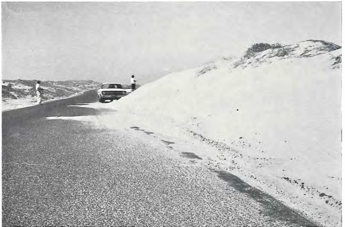
Plate 3 — Sand Drift Control. Sand Drift Across Roads, Before Application of Control Measures.
