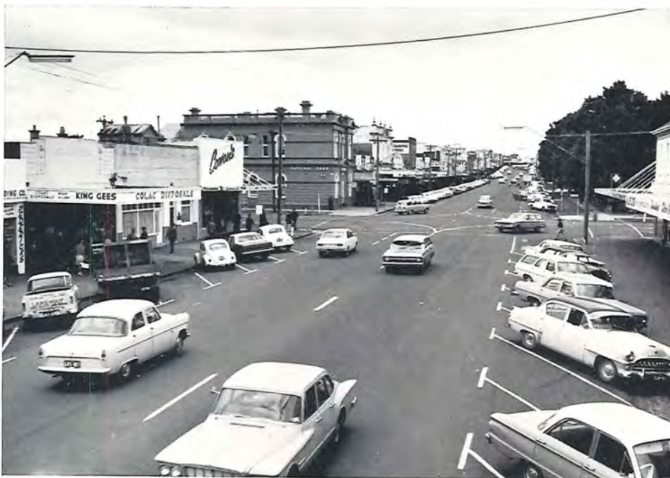
Princes Highway West — Widening of Murray Street, Colac.
