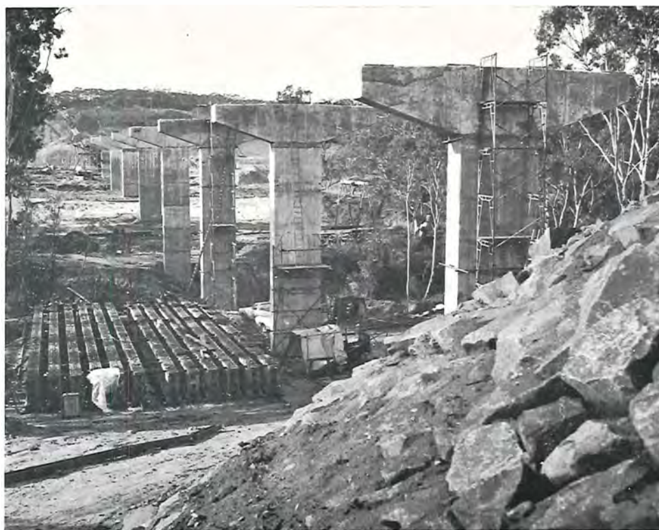
Plate 9 — Construction of the Glenelg River Bridge, Princes Highway West, Dartmoor.
