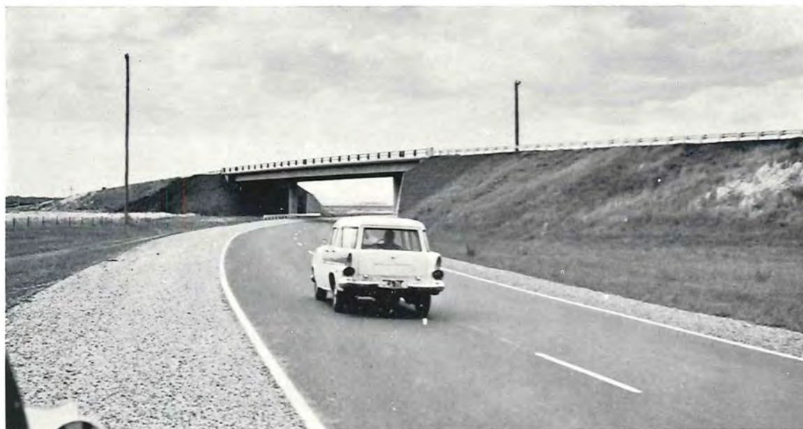
Tullamarine Freeway — Interchange bridge at Airport entrance.
