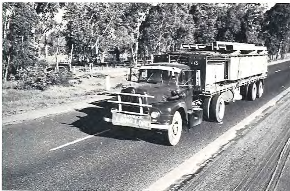
Hume Highway — Dual carriageways south of Tallarook.
