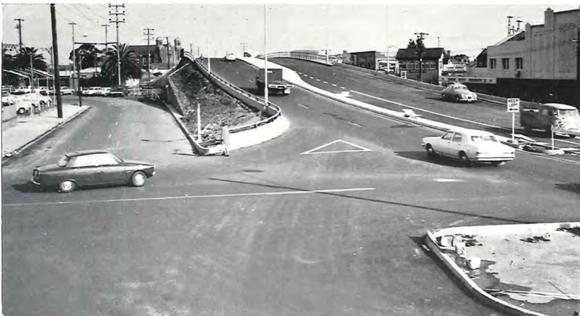
Warrigal Road — Road over rail overpass at Oakleigh.
