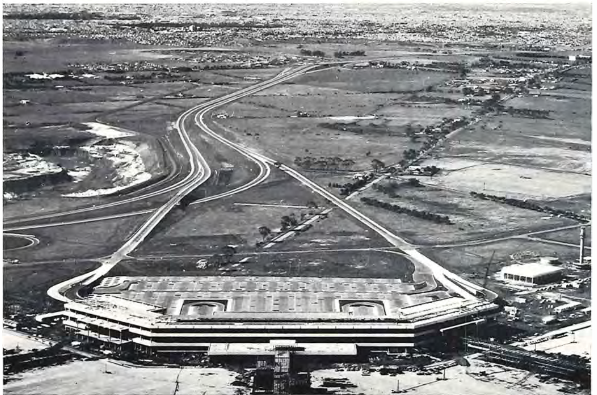
Aerial View of Tullamarine Freeway with Airport Terminal in the foreground.
