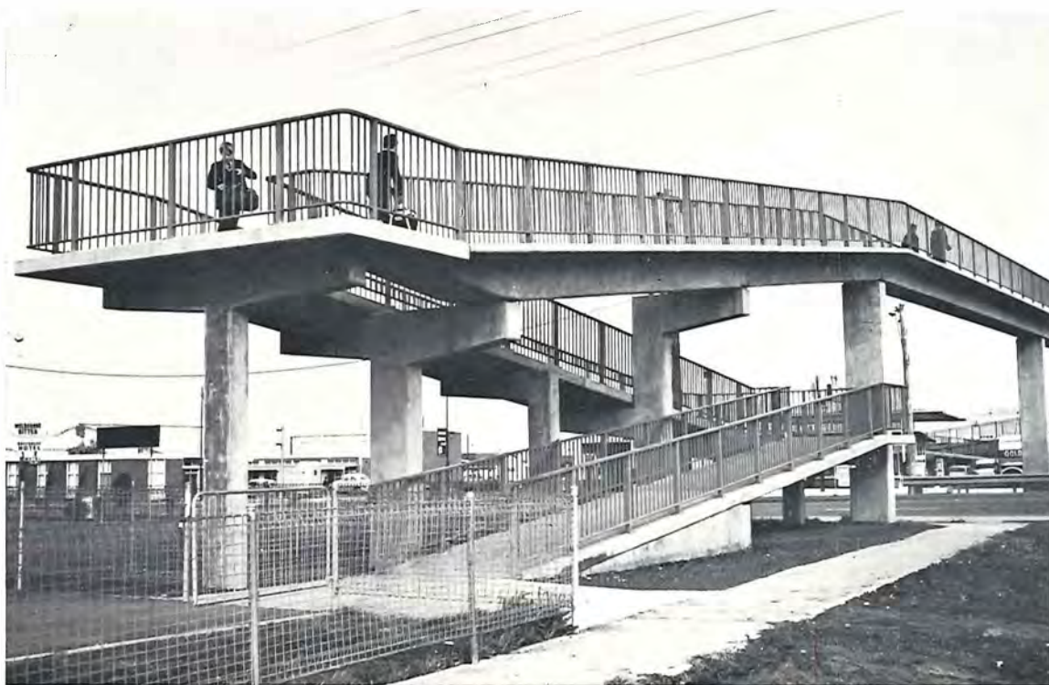
Pedestrian Overpass at Braybrook State School — Western Highway.
