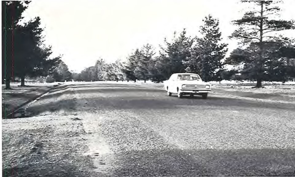
Glenelg Highway — Reconstructed section west of Hamilton.
