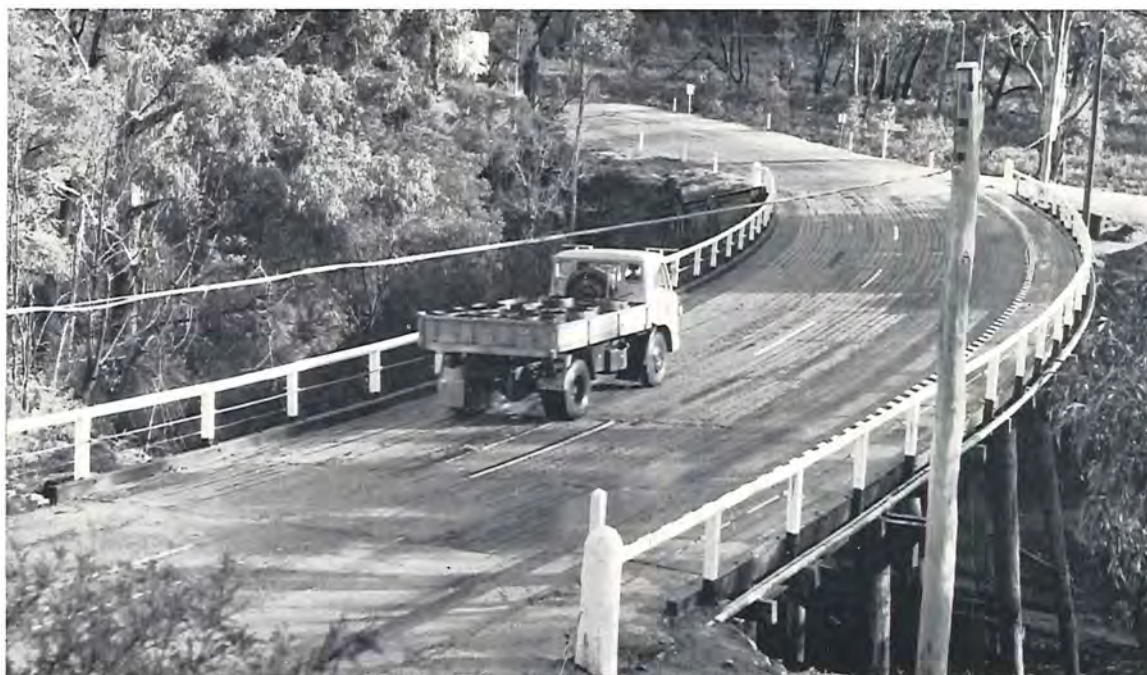
Grampians Tourists' Road — Widening of Delly's Bridge.
