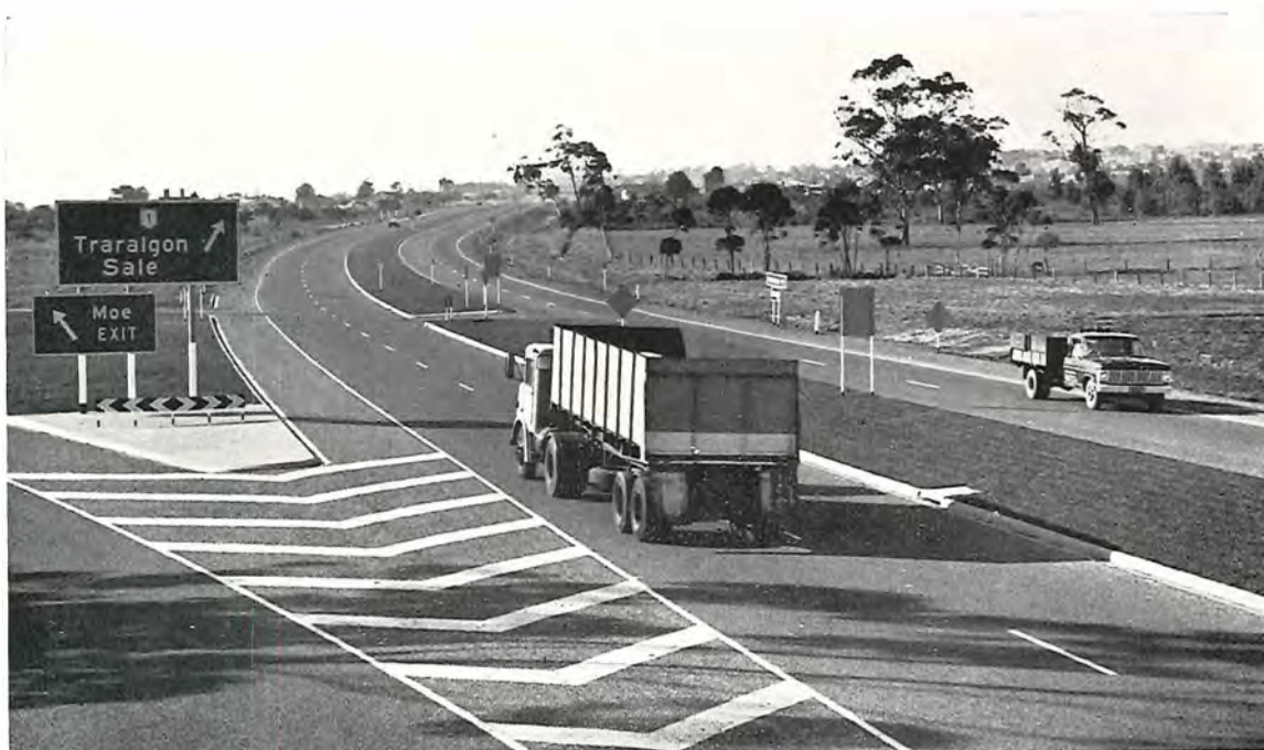
Special Project No. 9—The Princes By-pass Road (Moe Section) west of Moe.
