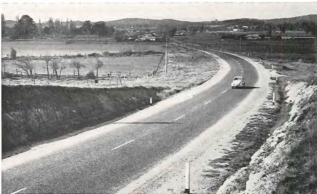
Midland Highway, Shire of Newstead. Widened section at Campbells Creek.
