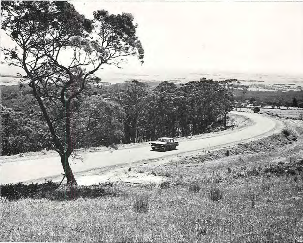
Dean Marsh-Lorne Forest Road, a realigned section north of Dean Marsh, Shire of Winchelsea.
