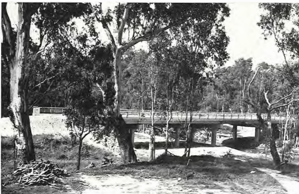
Bright Road, City of Wangaratta. New bridge over the King River.
