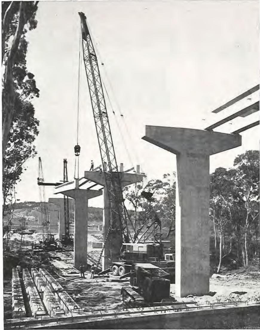
Princes Highway West, Shire of Portland. The Glenelg River Bridge at Dartmoor during construction.
