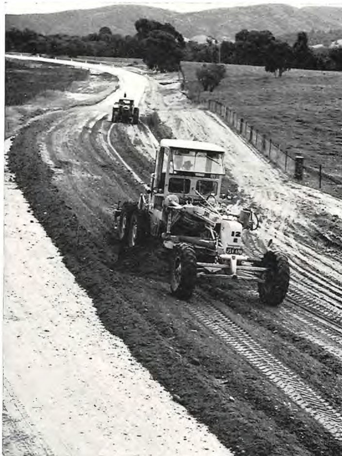
Osbornes Flat Road under reconstruction in the Shire of Yackandandah.
