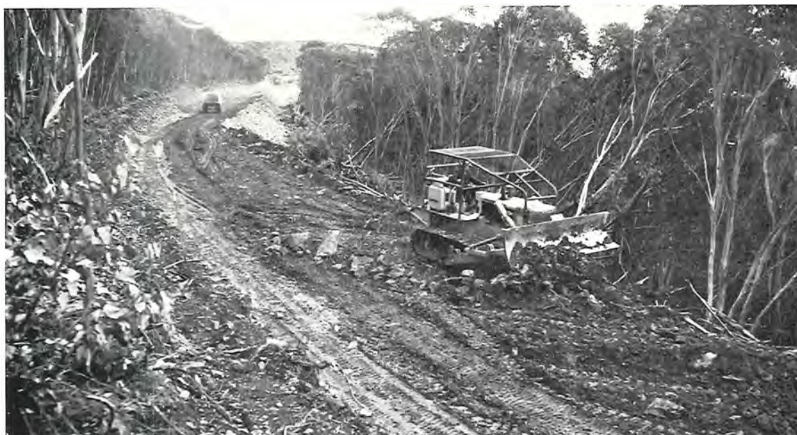
Special Project No. 15. The Jamieson-Licola Road. Construction in progress near Mount Skine.
