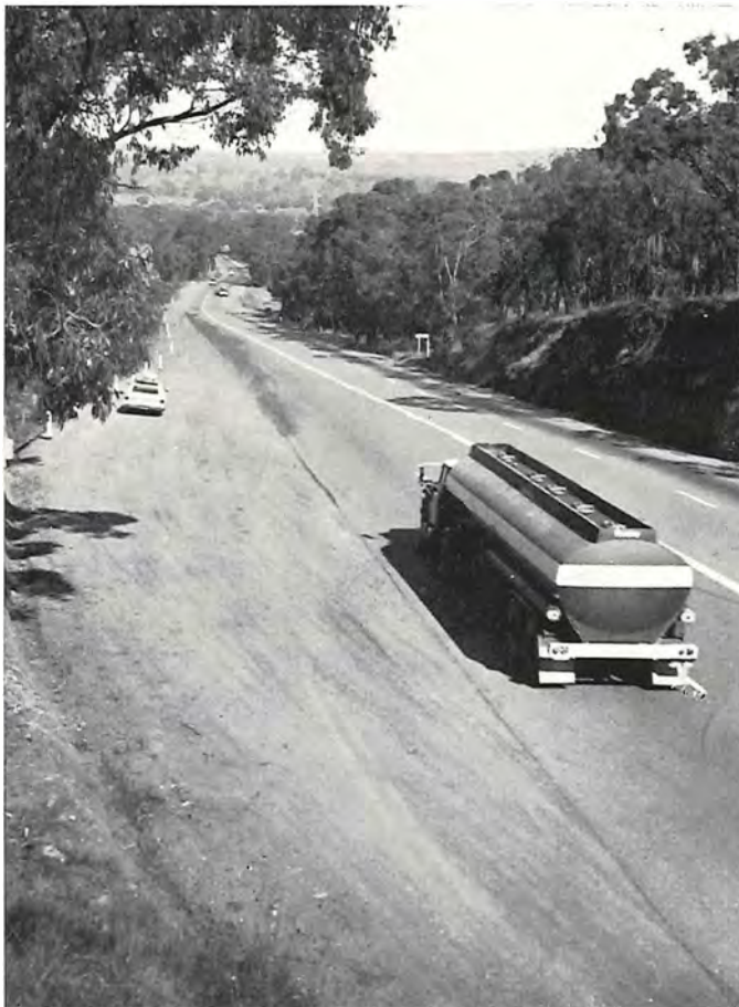
Calder Highway, Shire of Marong—Parking bay at Big Hill.
