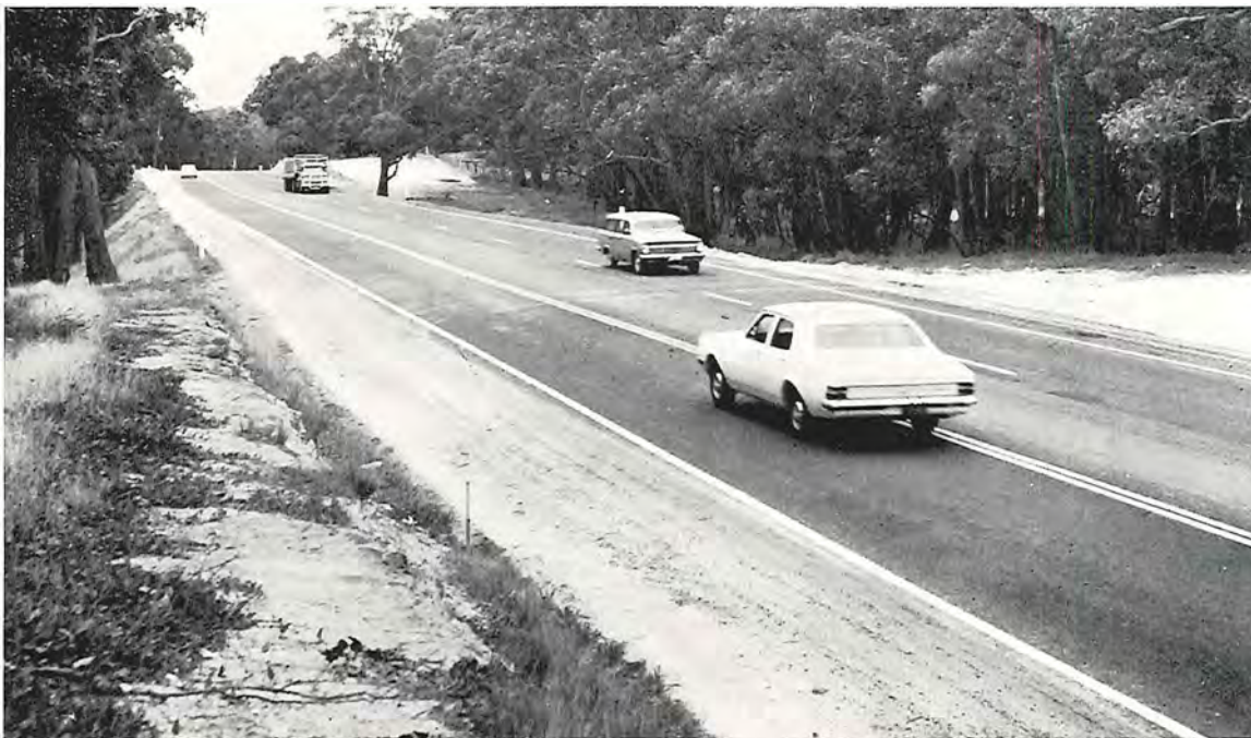
Calder Highway, Shire of Gisborne and Newham and Woodend. A climbing lane through the Black Forest.
