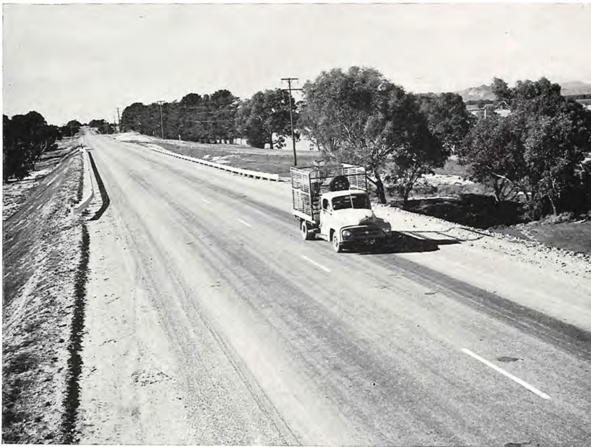
Western Highway, Shire of Wimmera. Reconstruction and realignment at Green Lakes.
