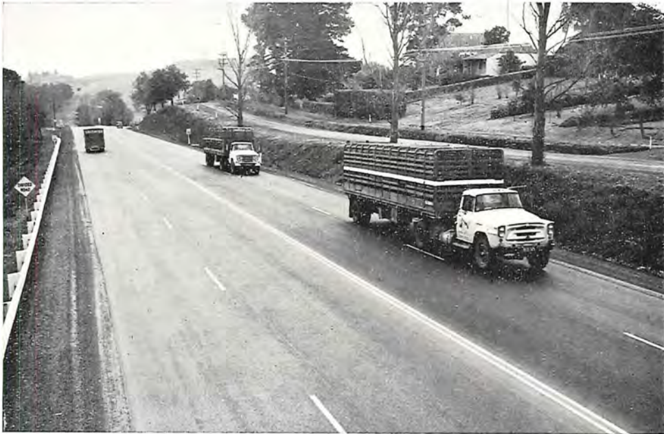
Princes Highway East, Shire of Berwick. Reconstruction to provide climbing lanes on Berwick Hill.
