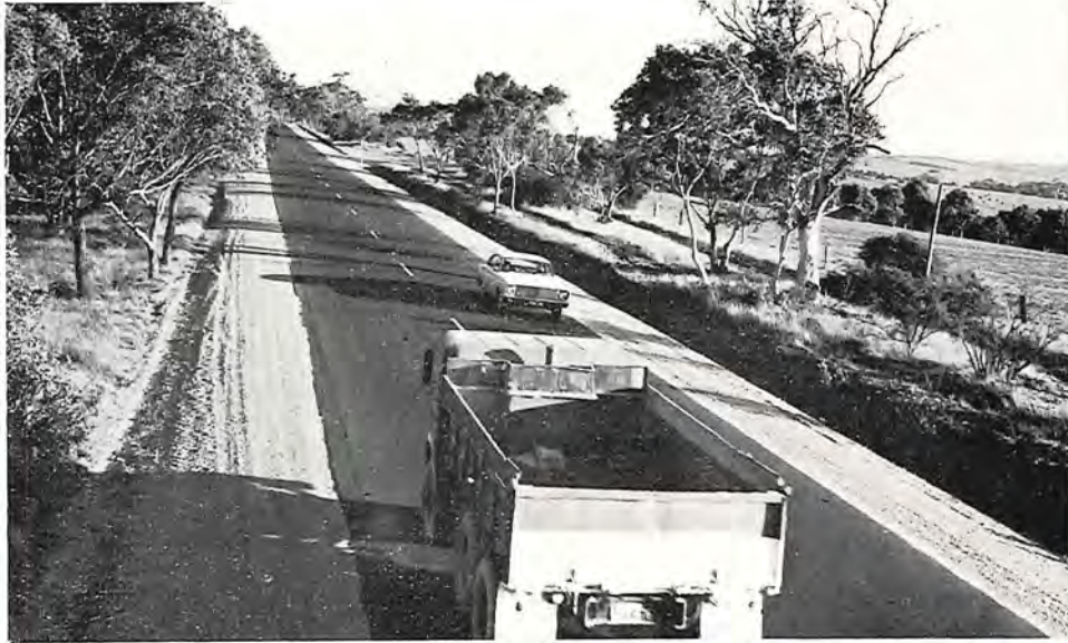
Moorooduc Road, Shire of Mornington. Reconstructed section south of Tyabb Road.
