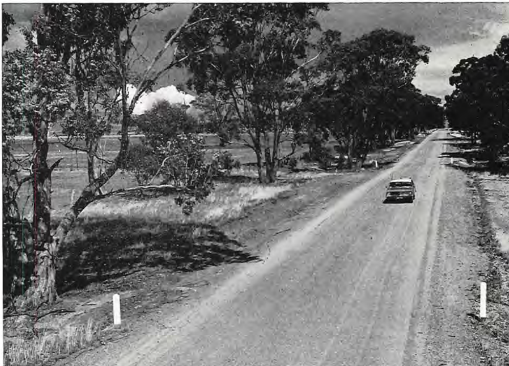
Benalla-Yarrowonga Road, Shire of Benalla. Widened section near Bungeet.
