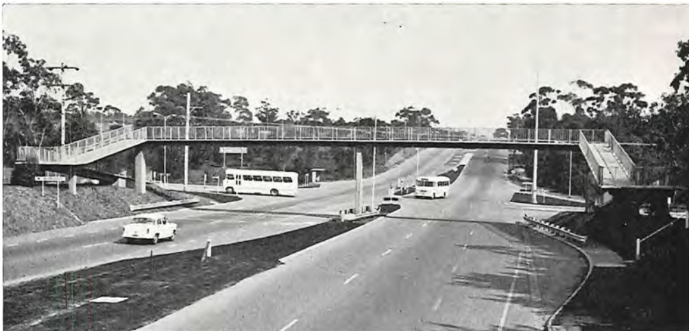
Nepean Highway, Shire of Mornington. Pedestrian overpass at Mount Eliza.
