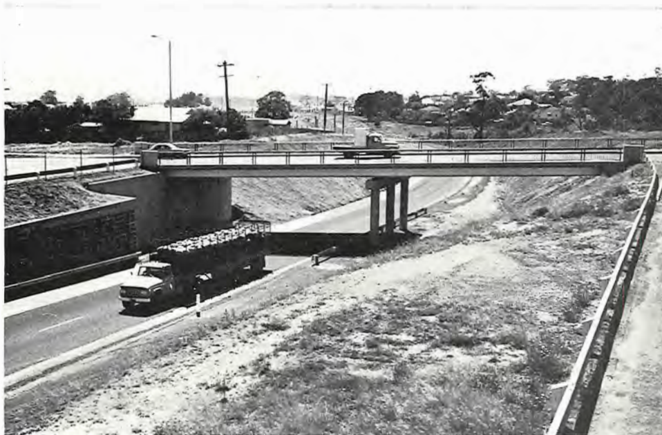
Princes Bypass Road (Moe Section) A reinforced concrete bridge providing grade separation.
