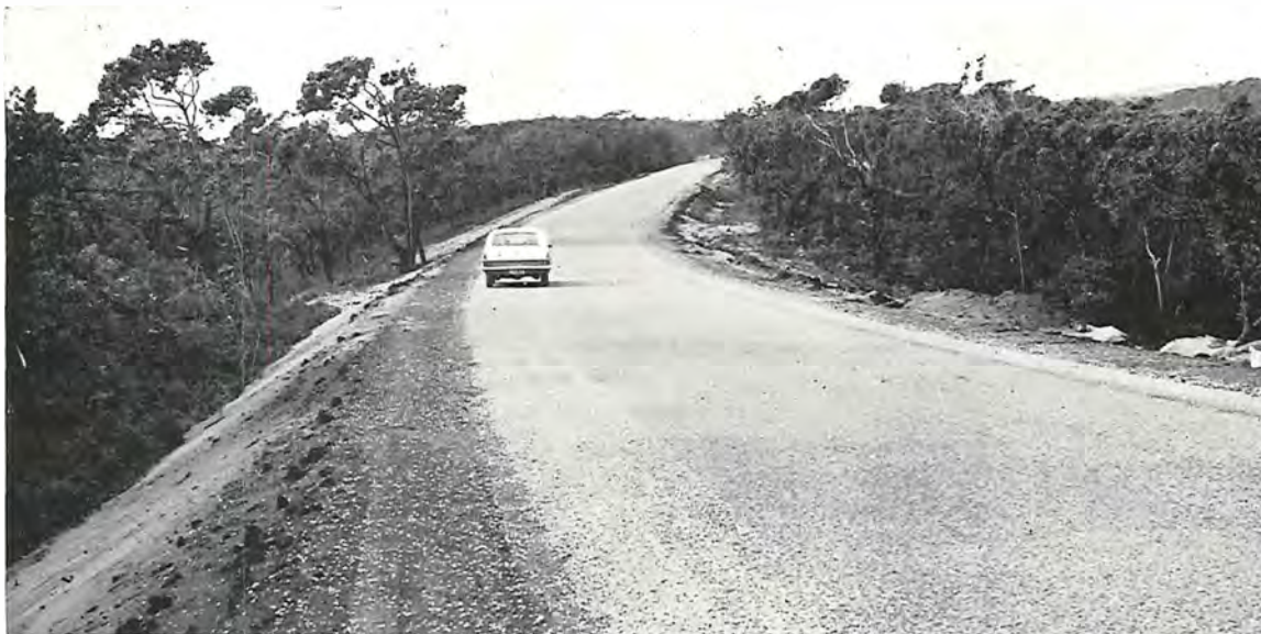
Special Project No. 14—Marlo—Cape Conran Road.
