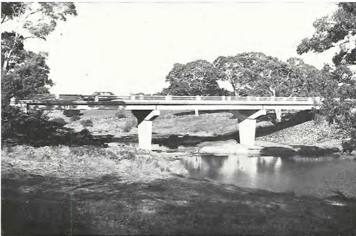
Glenelg Highway, Shire of Dundas. New Concrete Bridge over the Wannan River near Wannan.
