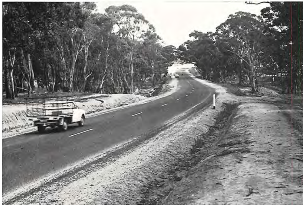
Pyrenees Highway, Shire of Ararat. Reconstructed section west of Elmhurst.
