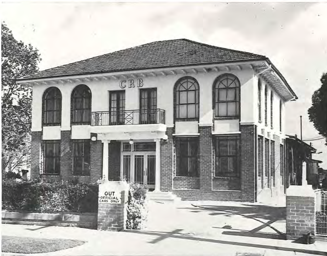
The Dandenong Divisional office at Nunawading.
