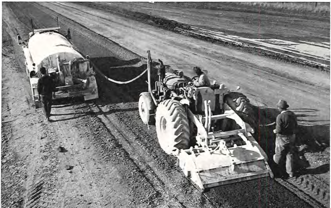
Plate 1—Lime Stabilization by Incorporating Lime Slurry into the Subgrade.
