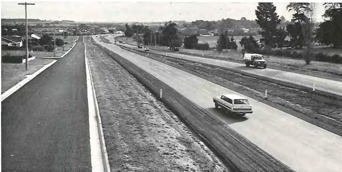
Princes Highway East, Shire of Berwick—Dual Carriageways east of Narre Warren.
