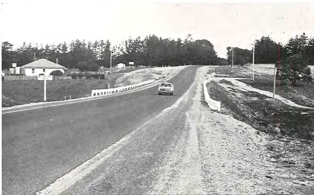
Midland Highway, Shire of Buninyong. Realignment and new culverts at Clarendon.
