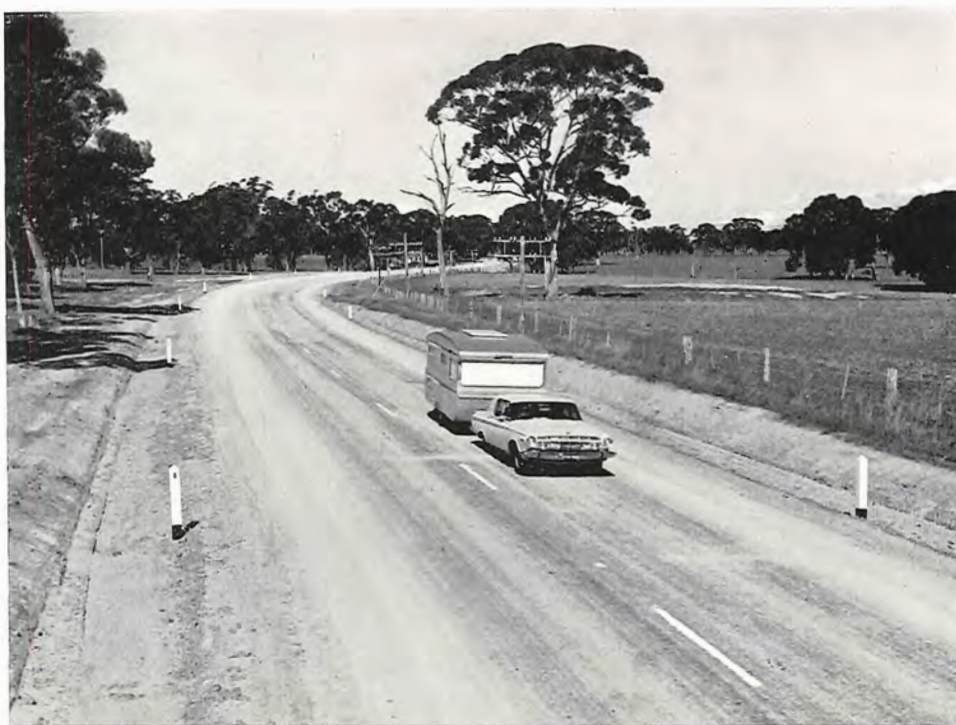
Henty Highway, Shire of Arapiles. Widened section between Mockinya and Wonwondah North.
