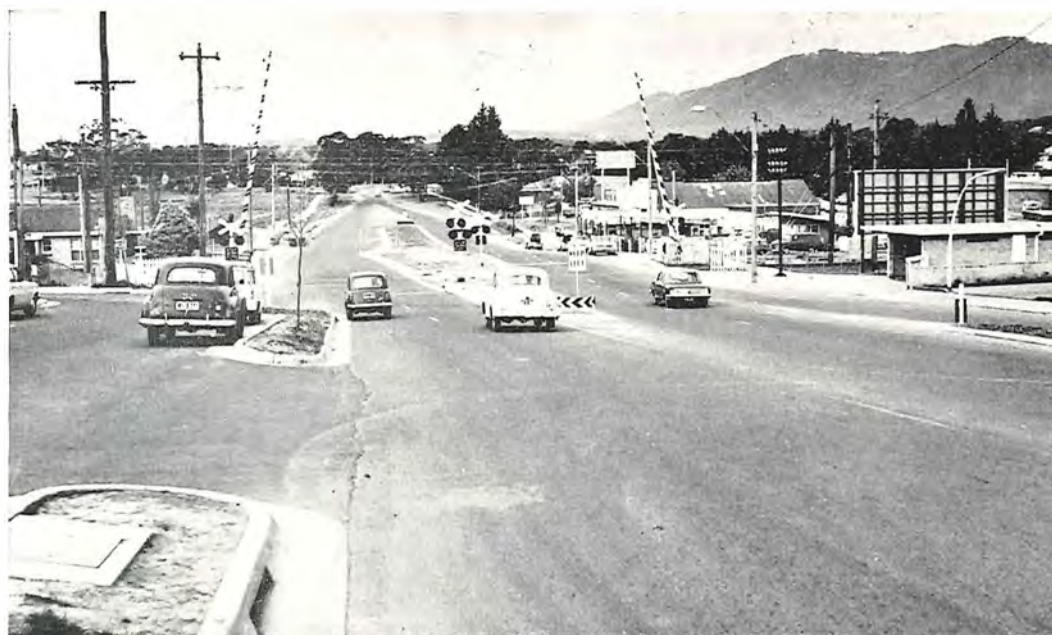
Wantirna-Sassafras Road, Knox City. Dual carriageways constructed at Bayswater.
