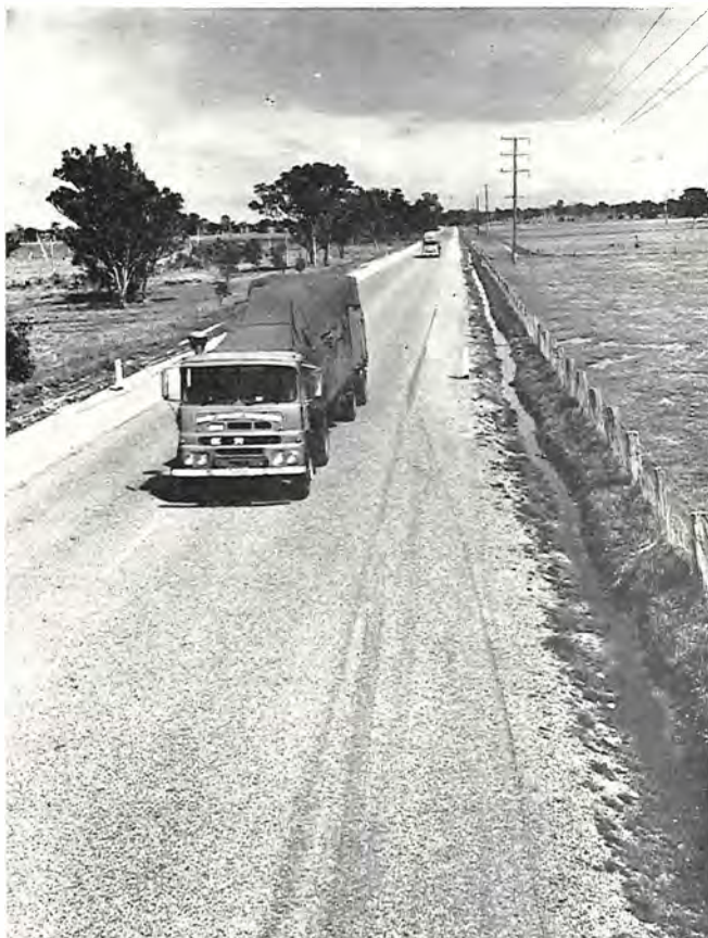
Widened section of the Princes Highway East to the west of Bairnsdale.
