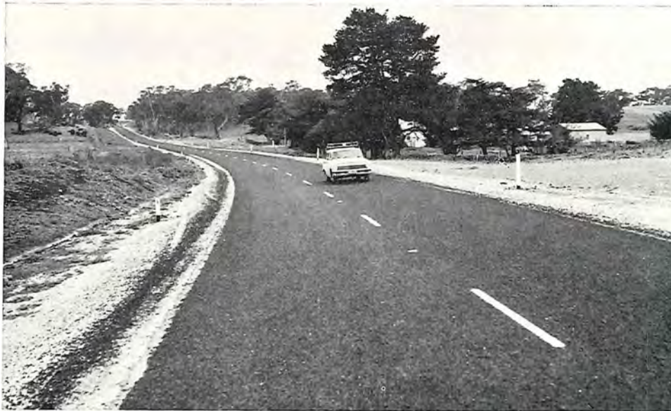
Reconstructed section of the Midland Highway north of Mount Franklin.
