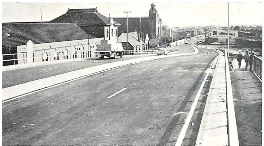
Four lane road over rail overpass at Somerville Road, Yarraville.
