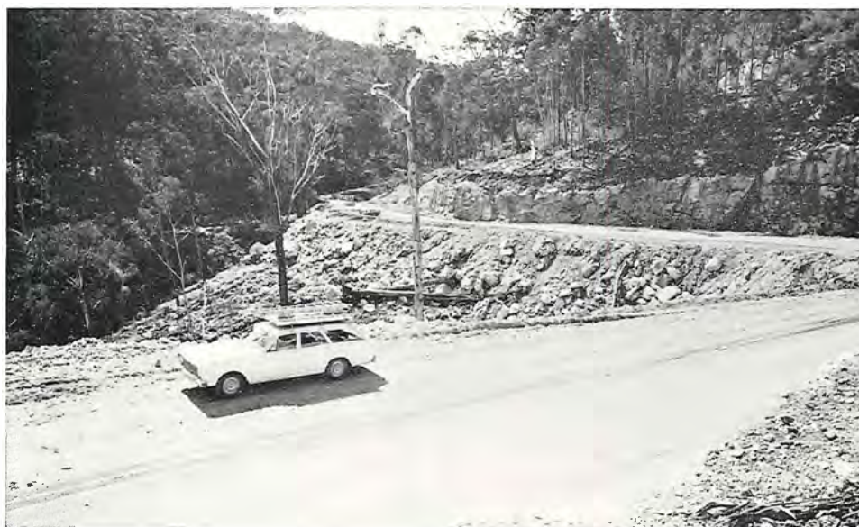
Gelantipy Road, Tambo Shire. Widened section at Murrindal.
