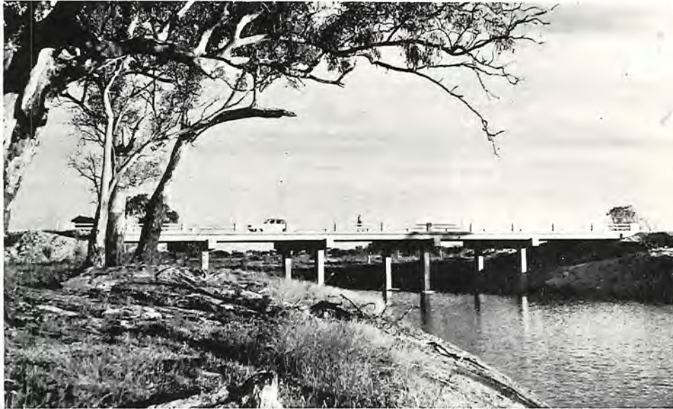
Nhill-Jeparit Road, Dimboola Shire. New bridge over the Wimmera River.
