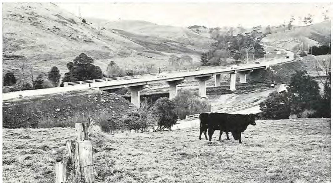
Overpass structure spanning Alsops Creek and the railway line on the South Gippsland Highway east of Loch.
