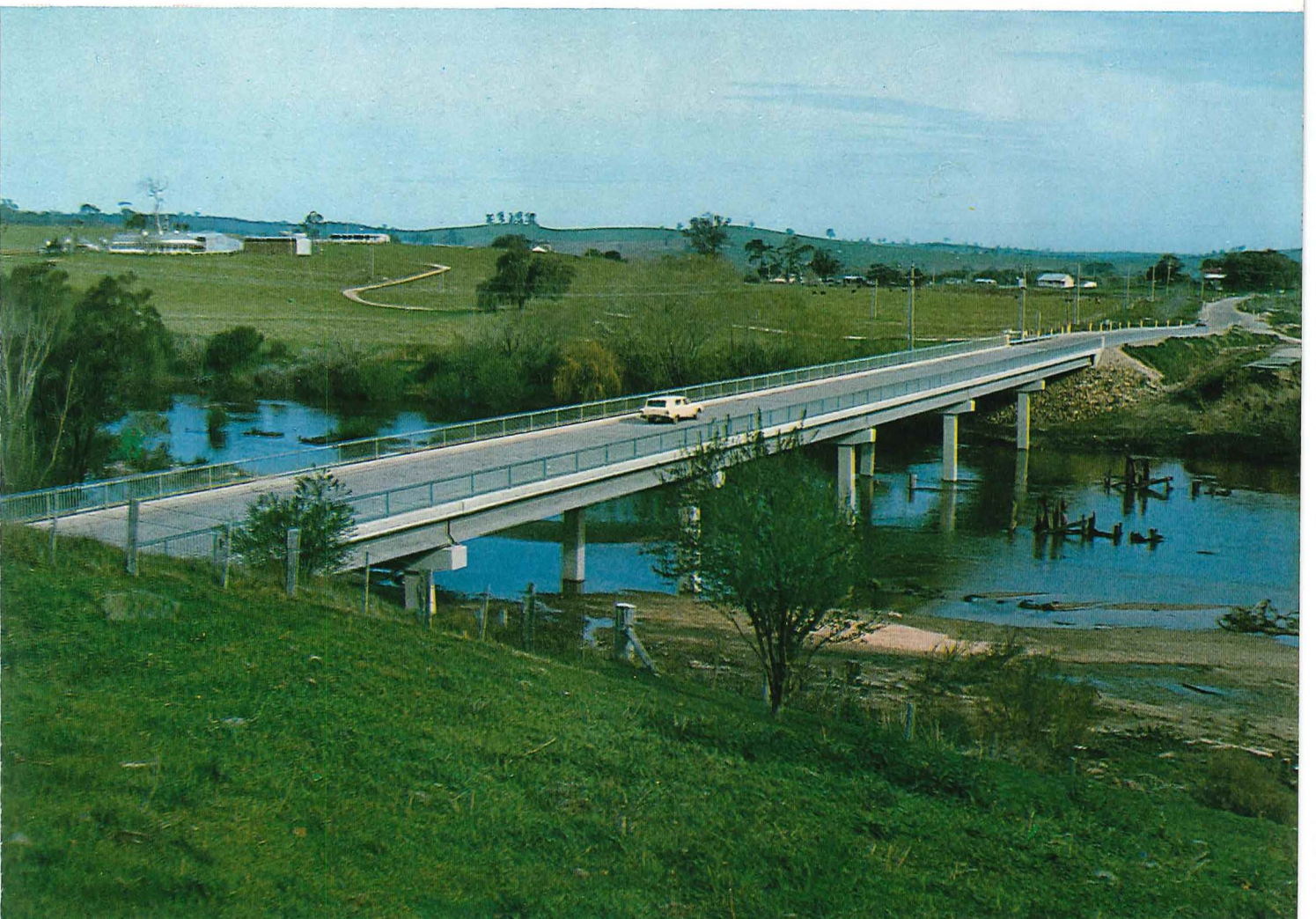
Tambo Upper-Road, Shire of Tambo. New bridge over Tambo River near Bruthen.
