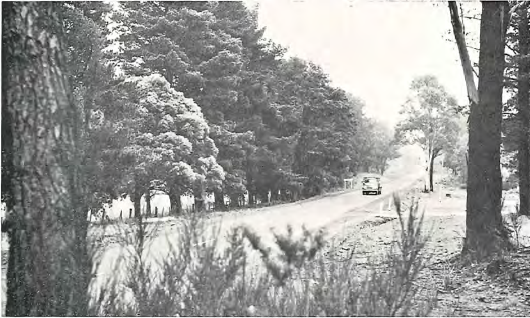
Whittlesea-Kinglake Main Road, Eltham Shire. Reconstructed section near Pheasant's Creek.
