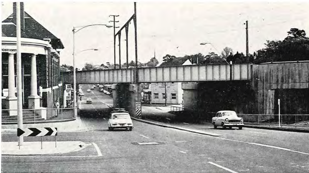
Road under rail grade separation which replaces the level crossing at Canterbury.
