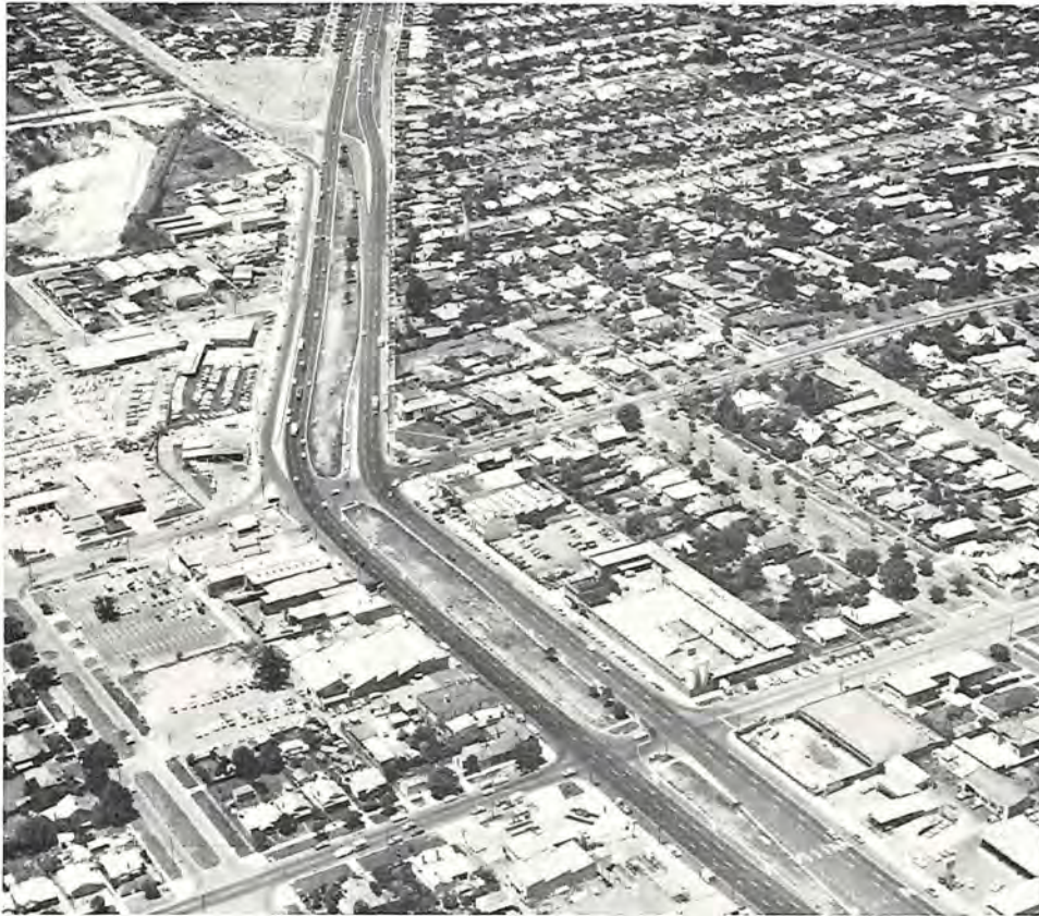
Princes Highway East—widened section between Warrigal Road and Ferntree Gully Road.
