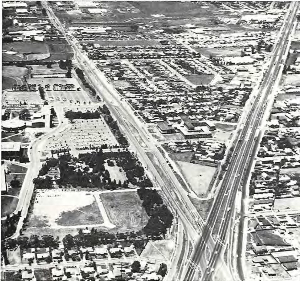
Wellington Road—dual carriageways constructed east of the Princes Highway.
