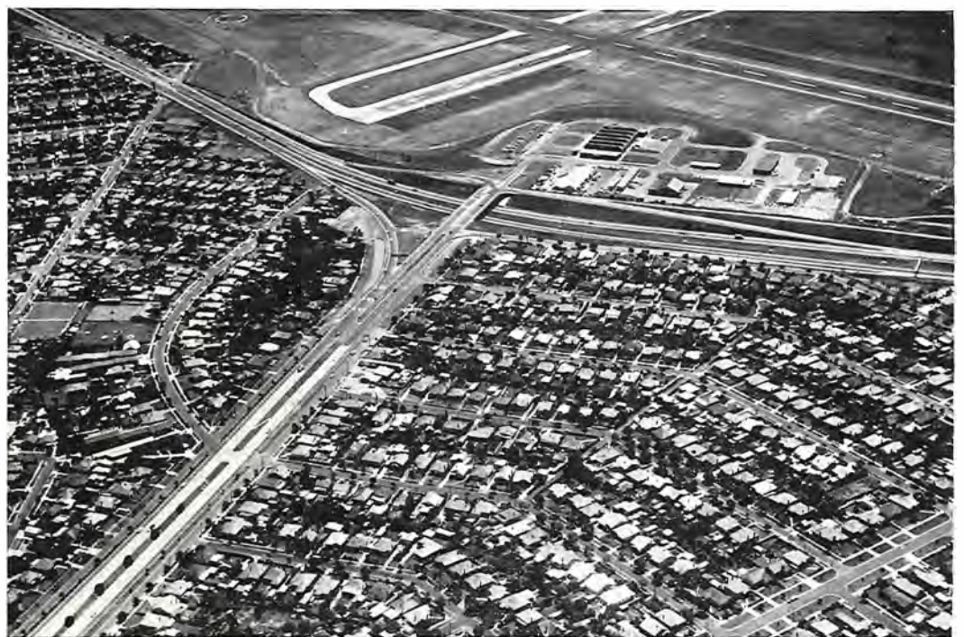
The Tullamarine Freeway, Bulla Road interchange.
