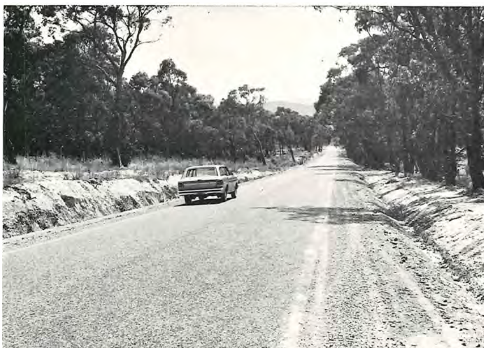
Reconstruction and widening of Donna Buang Road east of Healesville.
