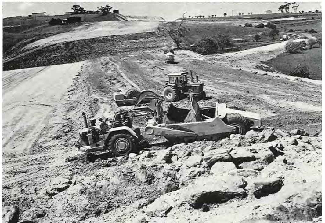
Earthworks in progress on the Western Freeway (Bacchus Marsh Section).
