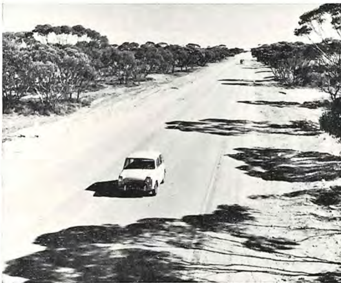
Reconstructed section of the Sturt Highway east of Cullulleraine.
