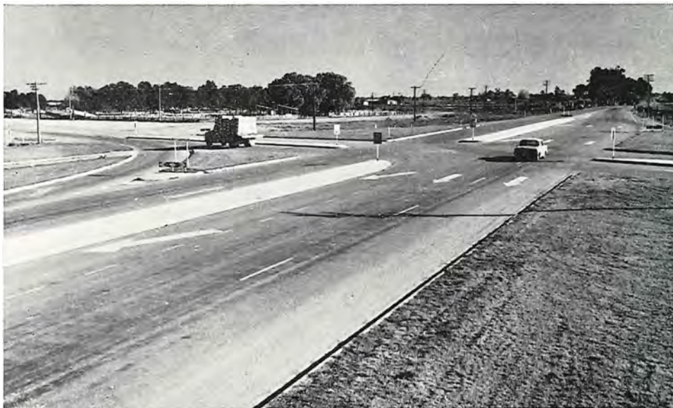
Dual carriageways and intersection treatment on the Murray Valley Highway at Swan Hill.
