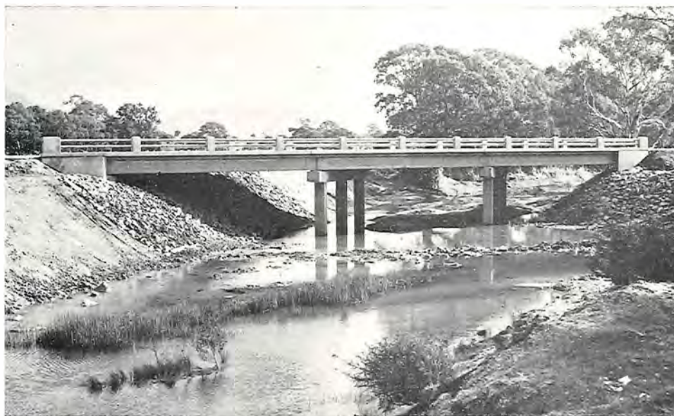
Ararat-Halls Gap Road, Ararat Shire. New bridge over Salt Creek.
