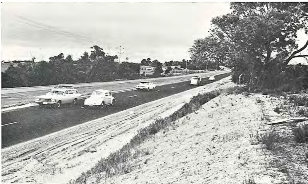
Dandenong-Frankston Road, Frankston City. Dual carriageways constructed south of O'Grady's Road.
