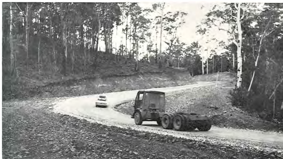
Widened section of the Bonang Highway north of Orbost.
