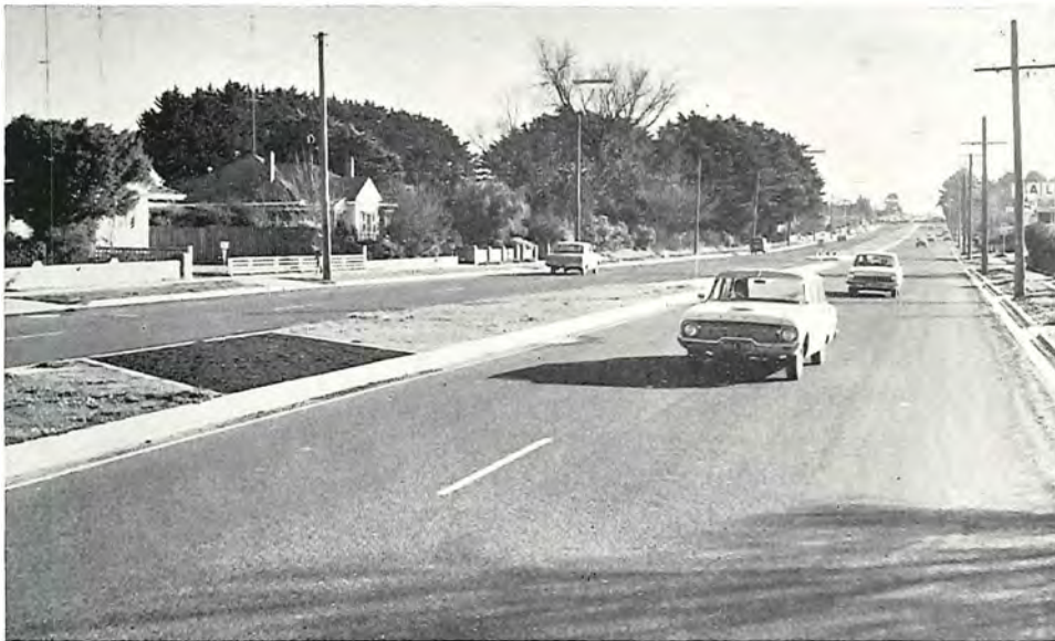
Dual carriageways constructed on the North Western Highway (Howitt Street), Wendouree.
