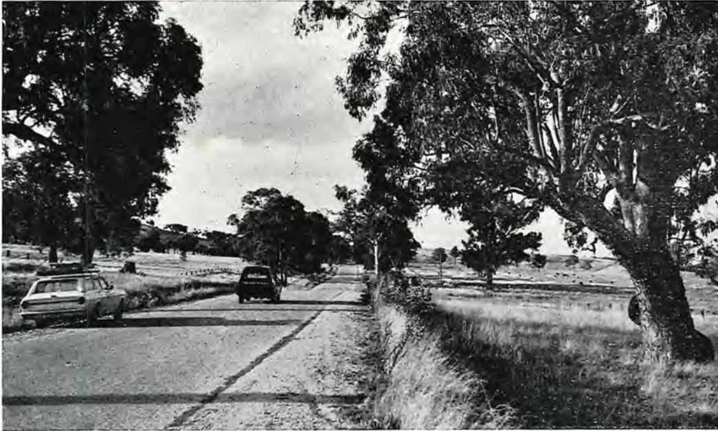
Yackandandah-Wodonga Road, Yackandandah Shire. One mile of this main road was reconstructed, realigned, and sealed.
