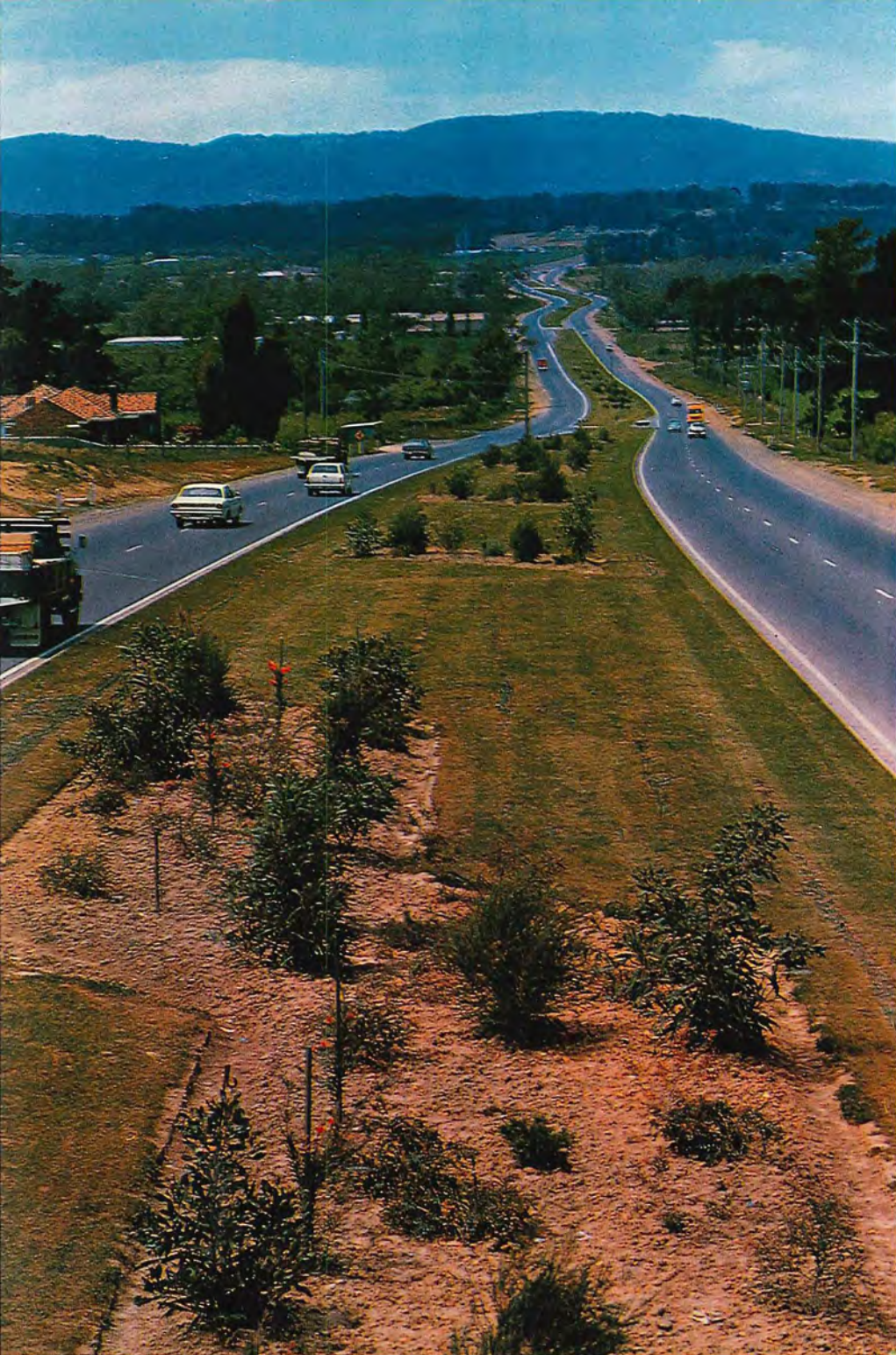
The Burwood Highway looking east towards Dandenong Creek showing recent planting of shrubs in the median.
