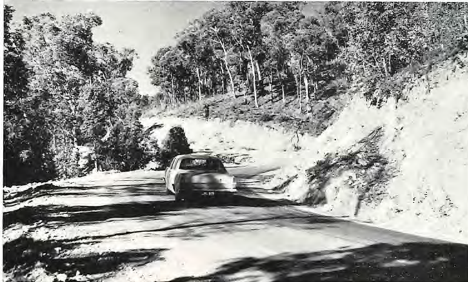
Bright-Tawonga Road, Bright Shire. Section resheeted and sealed.
