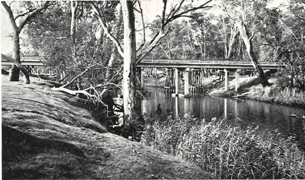
Goornong-Barnadown Road, Waranga and Huntly Shires. Five span bridge built over the Campaspe River.
