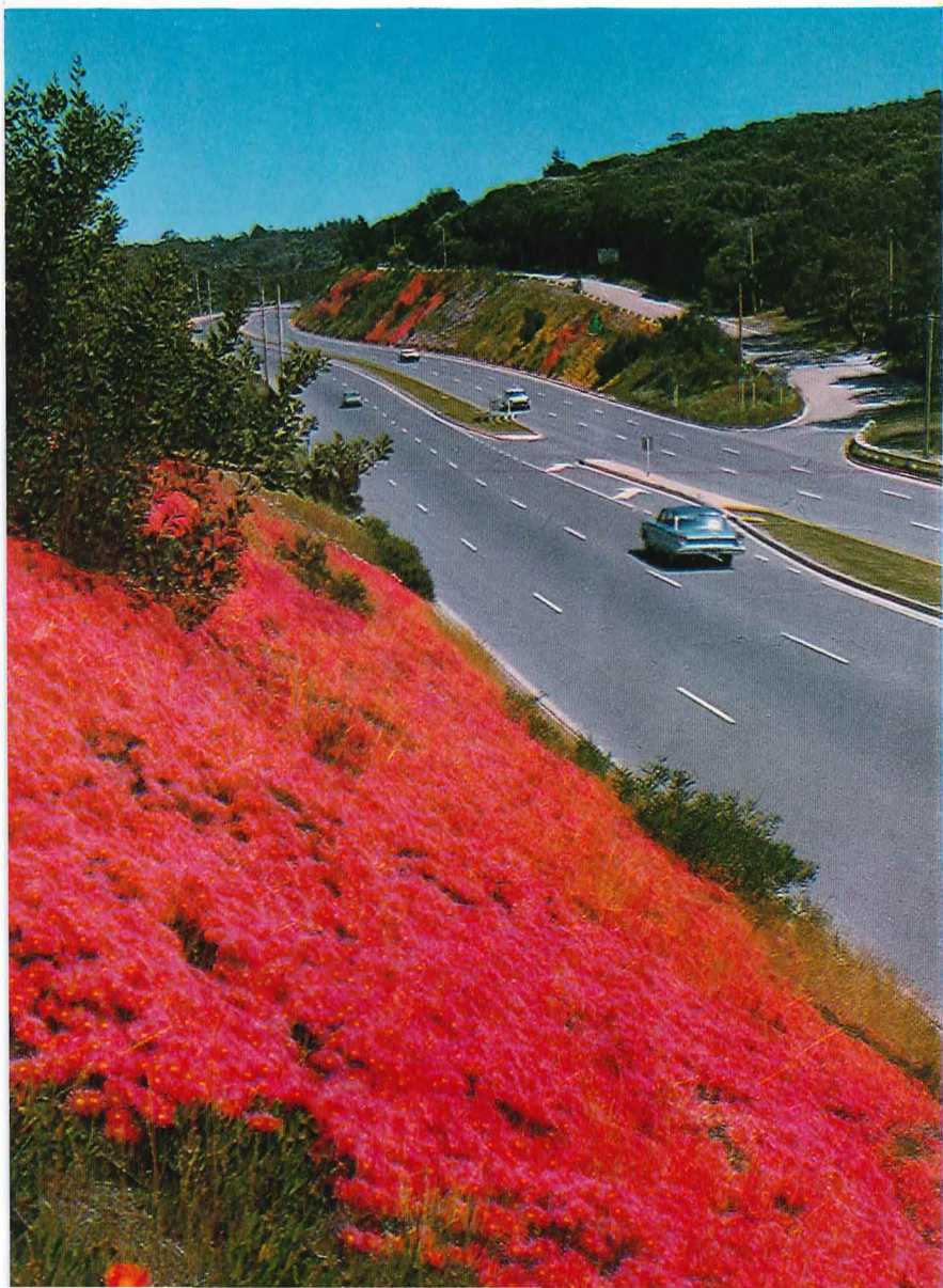
Batter treatment on the Nepean Highway at Mount Eliza.
