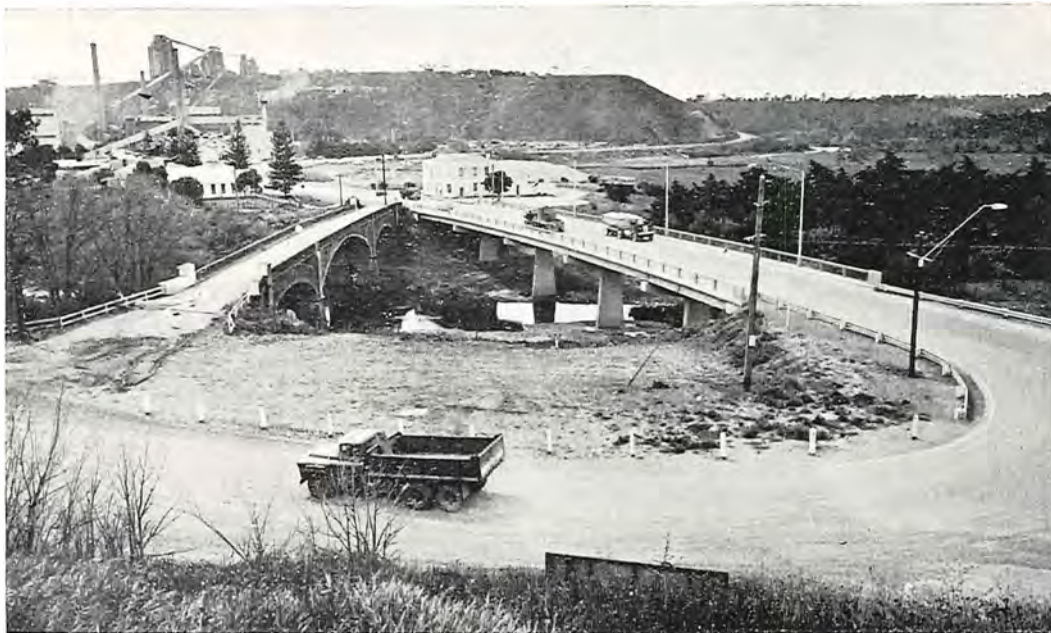
New five span bridge on the Hamilton Highway over the Moorabool River at Fyansford.
