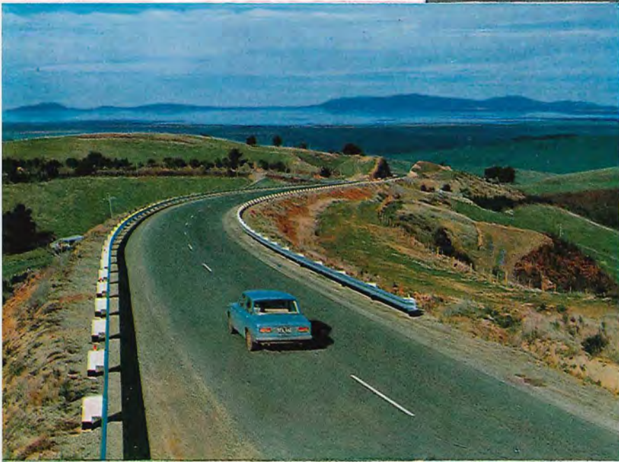
Realigned section of the South Gippsland Highway north of Foster.
