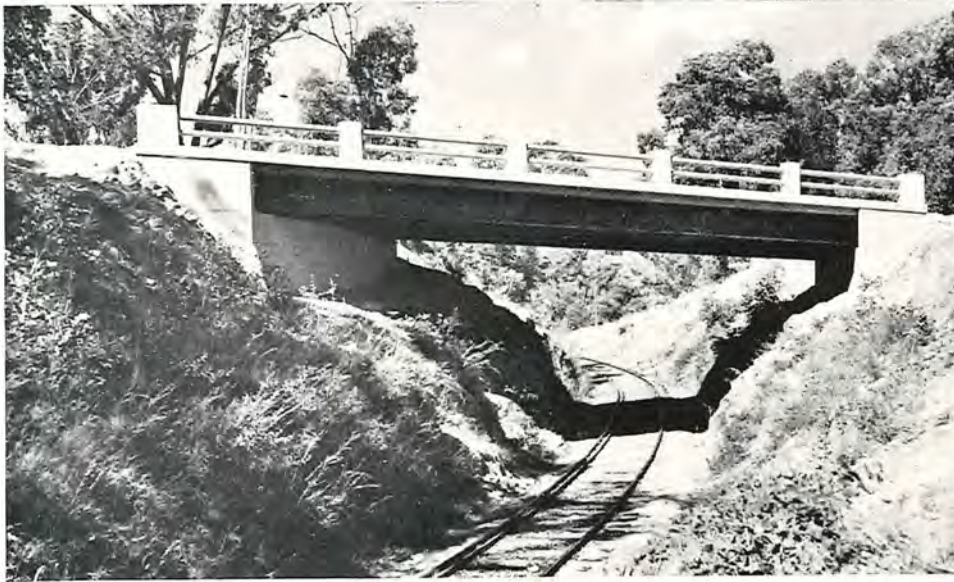
Tallangatta-Corryong Road, Towong Shire. New bridge over the railway at Darbyshire.
