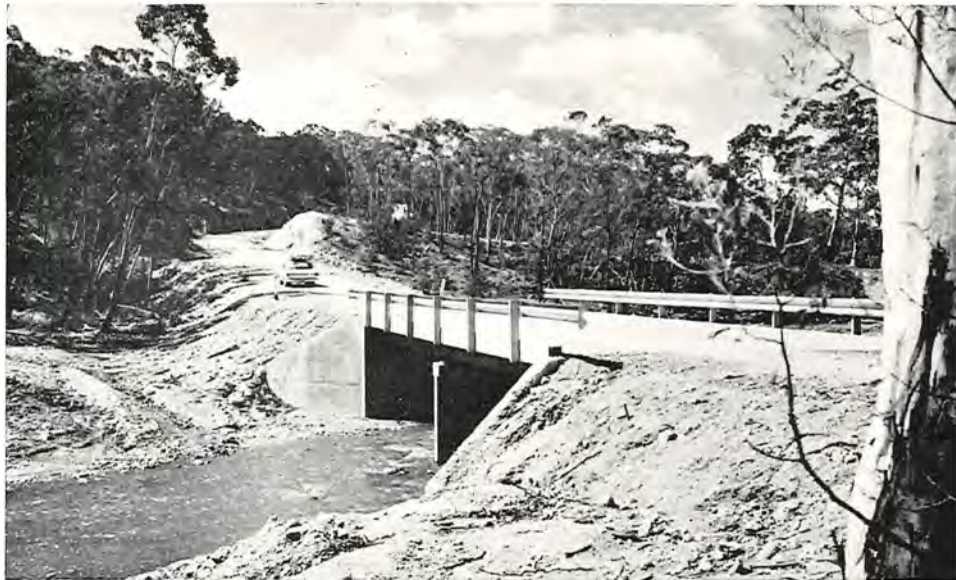
Snowy River Road, Tambo Shire. New bridge over Goodwin Creek.
