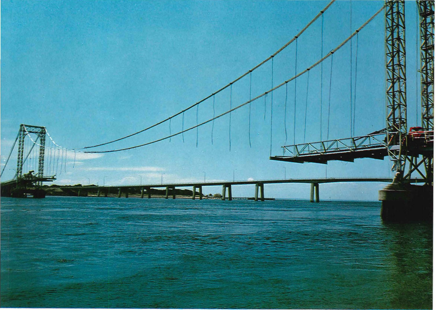
Dismantling the old suspension bridge built in 1938.
