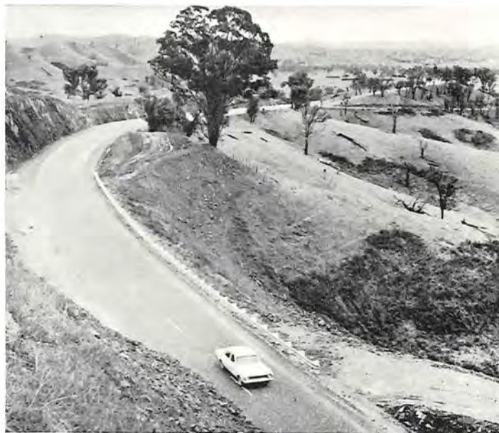
The Maroondah Highway reconstructed at Acheron Cutting.
