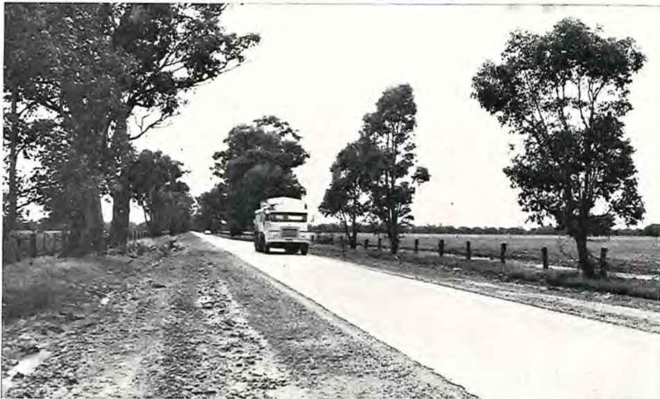
Reconstructed section of the Nagambie-Locksley Road, Goulburn Shire.
