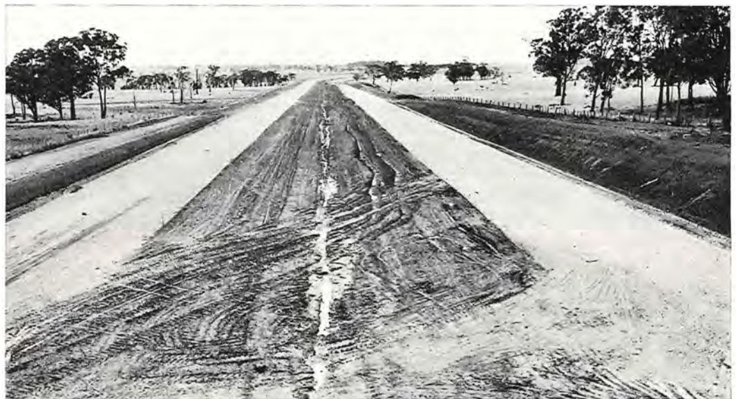
The Western Freeway (Gordon Section) under construction.
