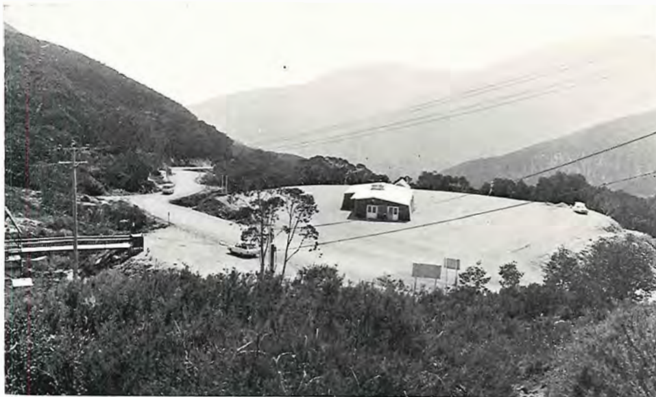
The Bogong High Plains Road reconstructed and sealed at Falls Creek.
