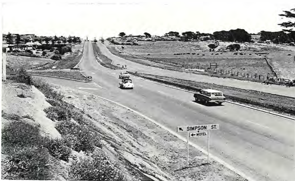
Dual carriageways constructed on the Princes Highway West at Warrnambool.
