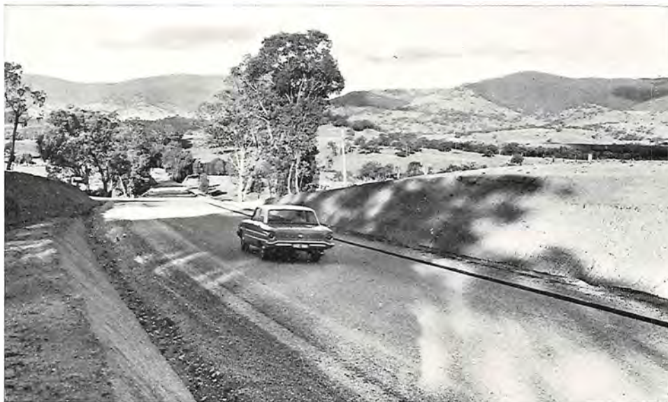
Reconstructed section of the Yackandandah-Wodonga Road, Yackandandah Shire.
