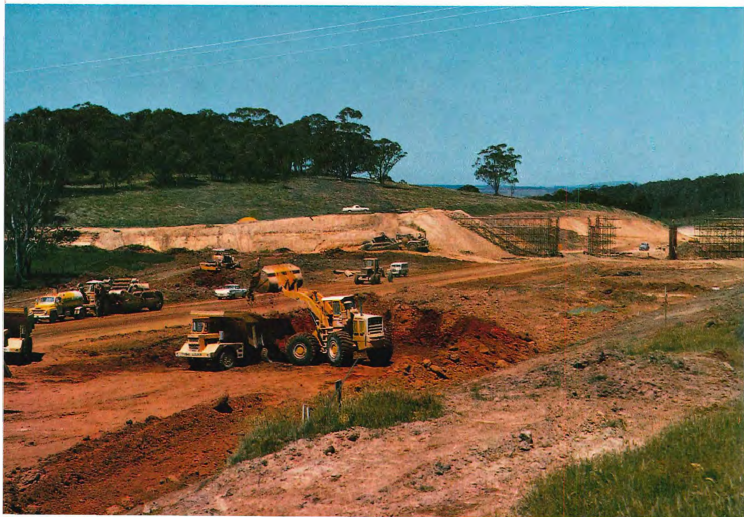
Work in progress on the Western Freeway (Gordon Section)
