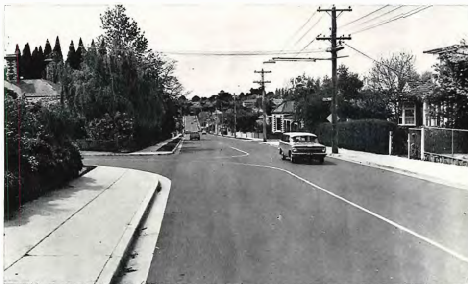
Reconstruction of Wellington Street, Kew City.
