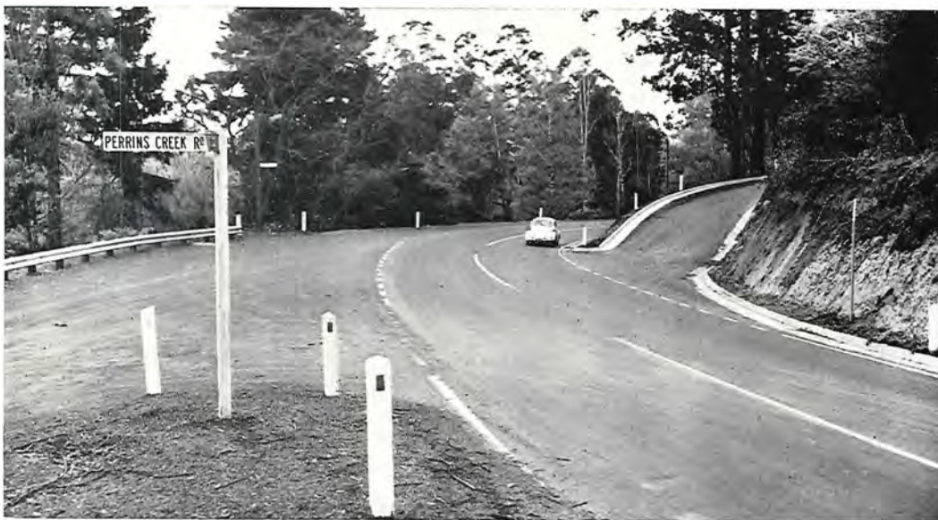
Widened section of the Mount Dandenong Tourists' Road near Sassafras.
