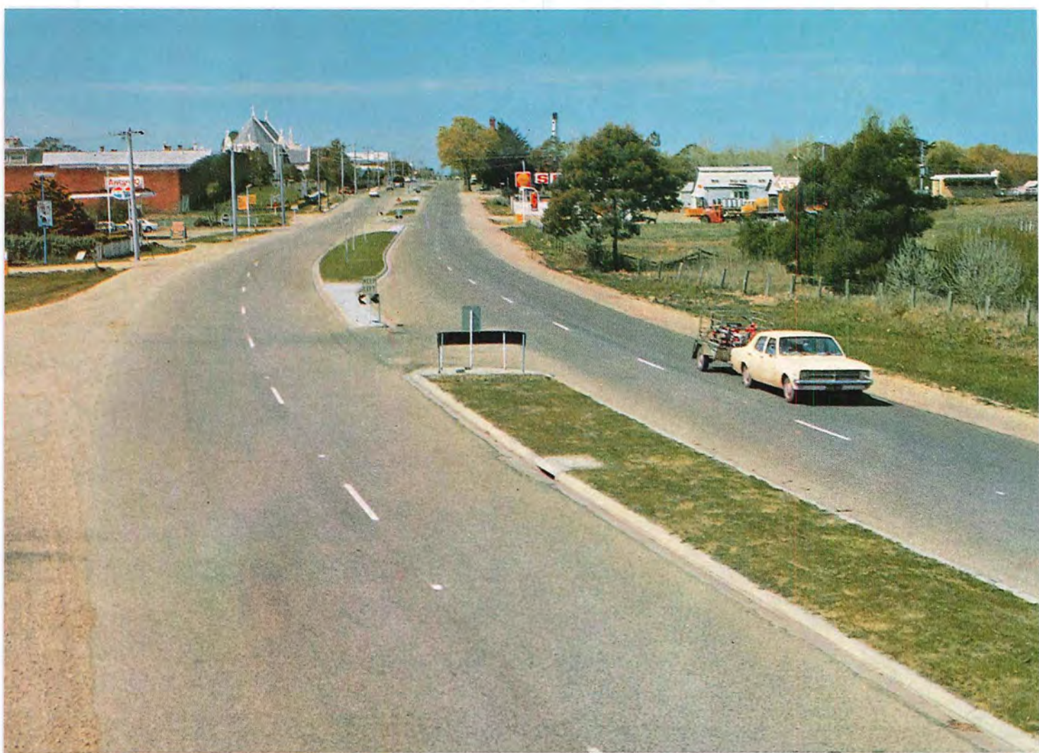
Dual carriageways constructed on the Princes Highway at Sale
