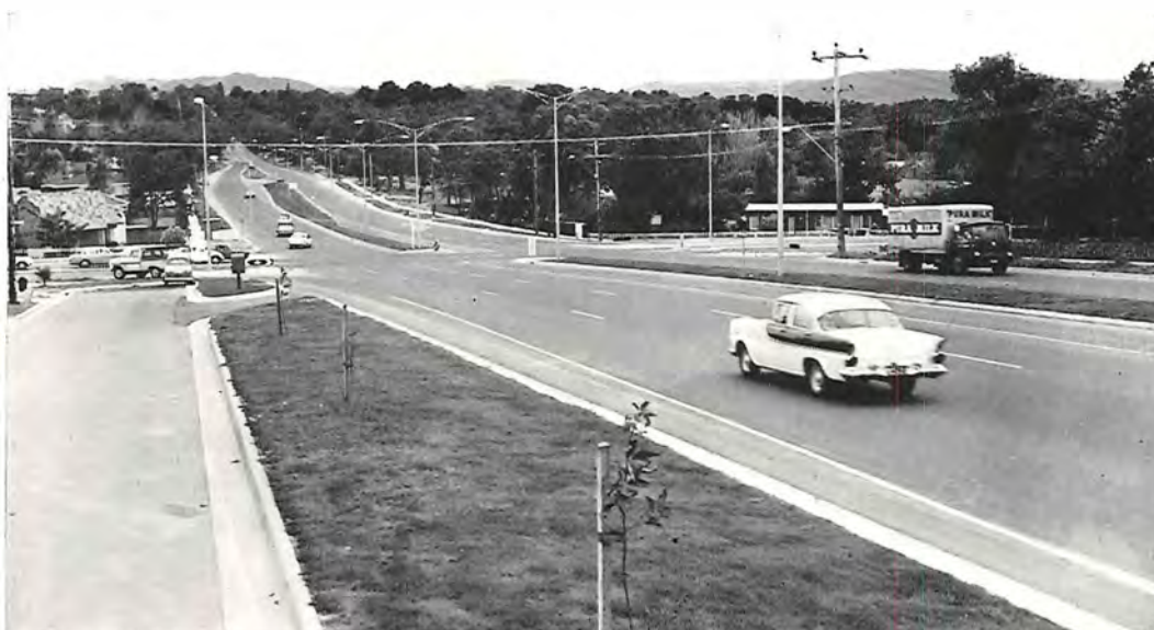
Reconstruction of the intersection of Canterbury Road and Wantirna Road.
