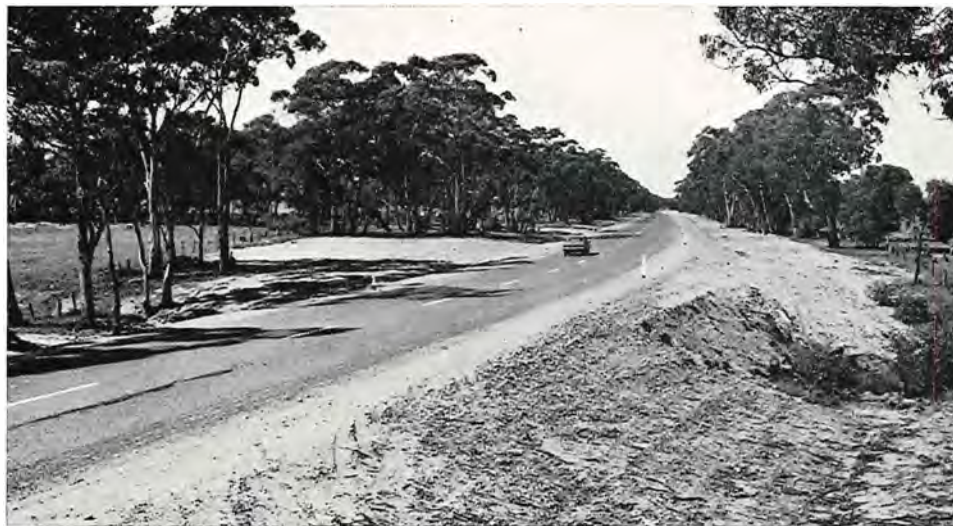
North Western Highway reconstructed between Lamplough and Avoca.
