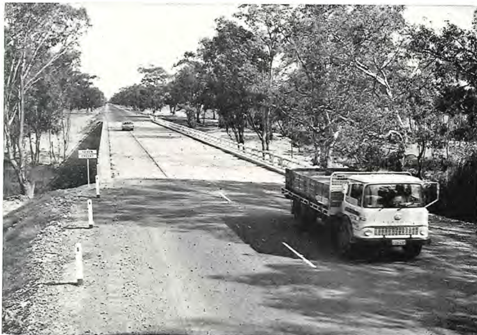
Bridge over Seven Creeks on the Goulburn Valley Highway which was widened to 28 feet between kerbs.
