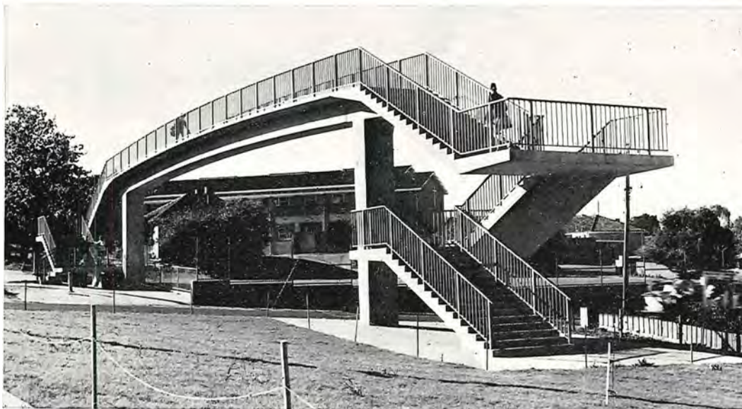
Pedestrian overpass over Heidelberg Road at Silk Street, Rosanna.
