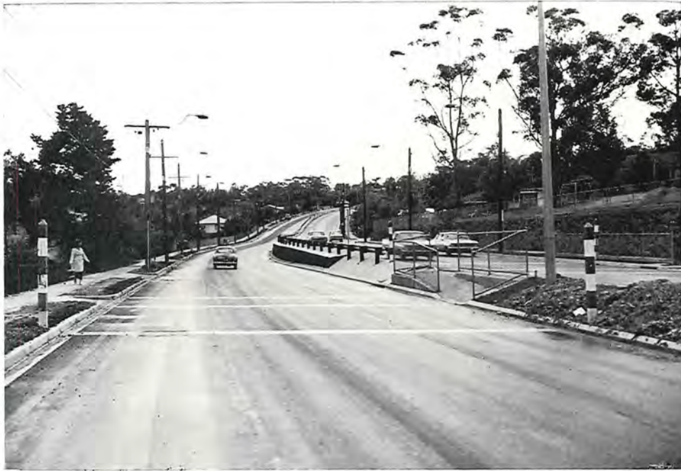
Dual carriageways constructed on the Eltham-Yarra Glen Road, Eltham Shire.
