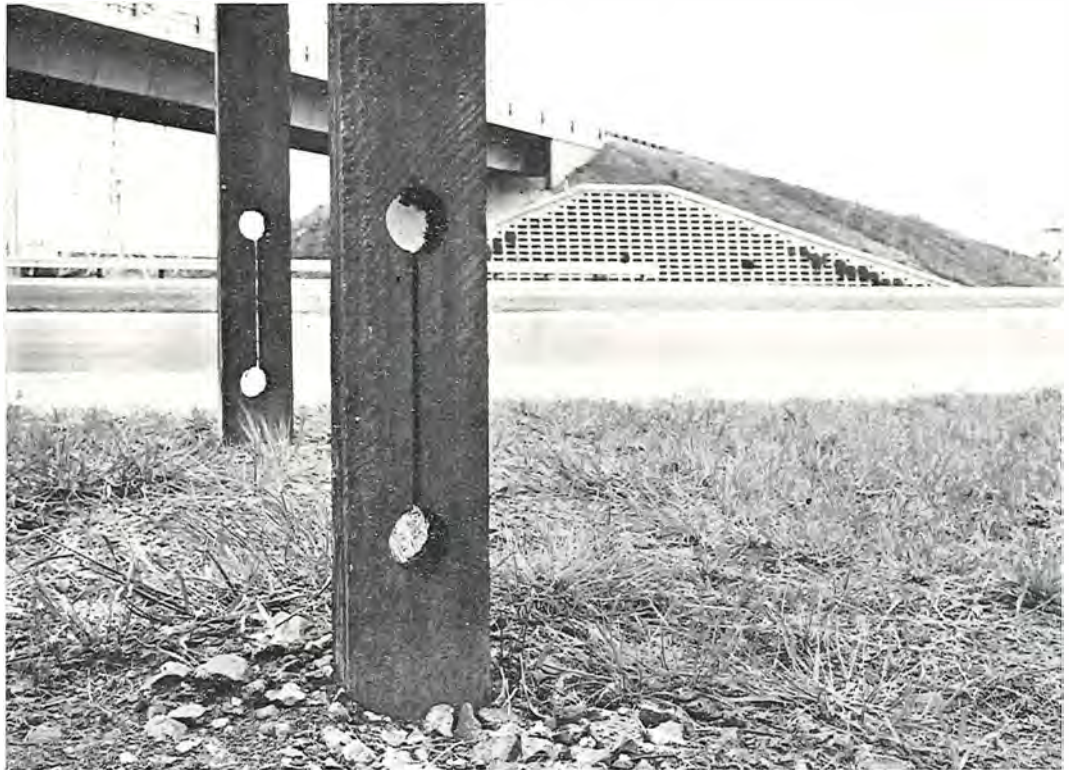
Plate 10—Frangible timber posts.
