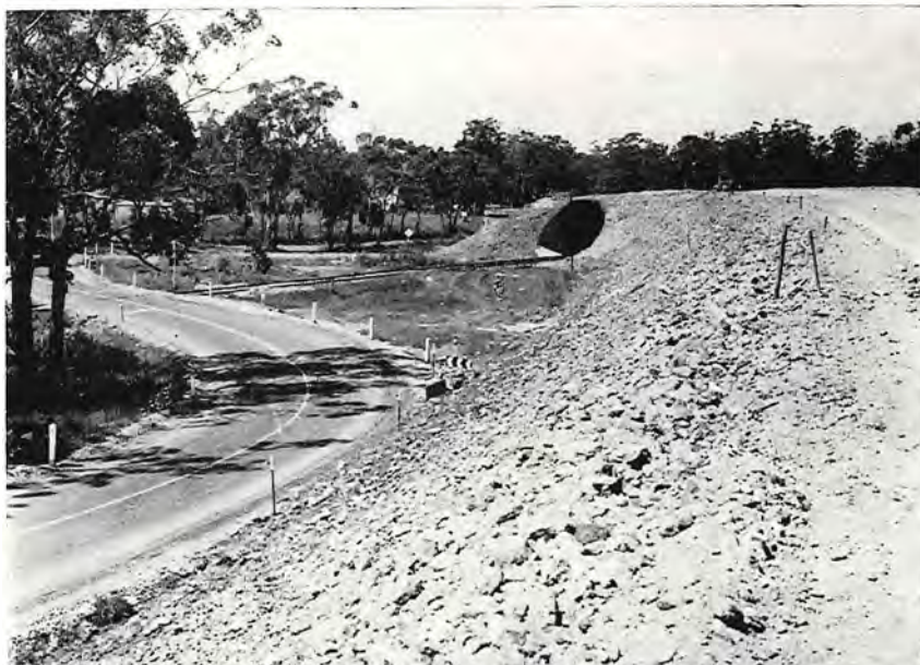
Plate 1—View of Lyons grade separation structure (before completion of the roadworks) showing the sharp approach curves to the rail level crossing.
