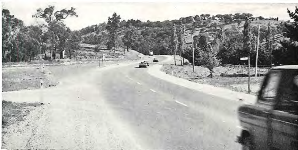
Reconstructed section of the Maroondah Highway east of the Warburton Highway.
