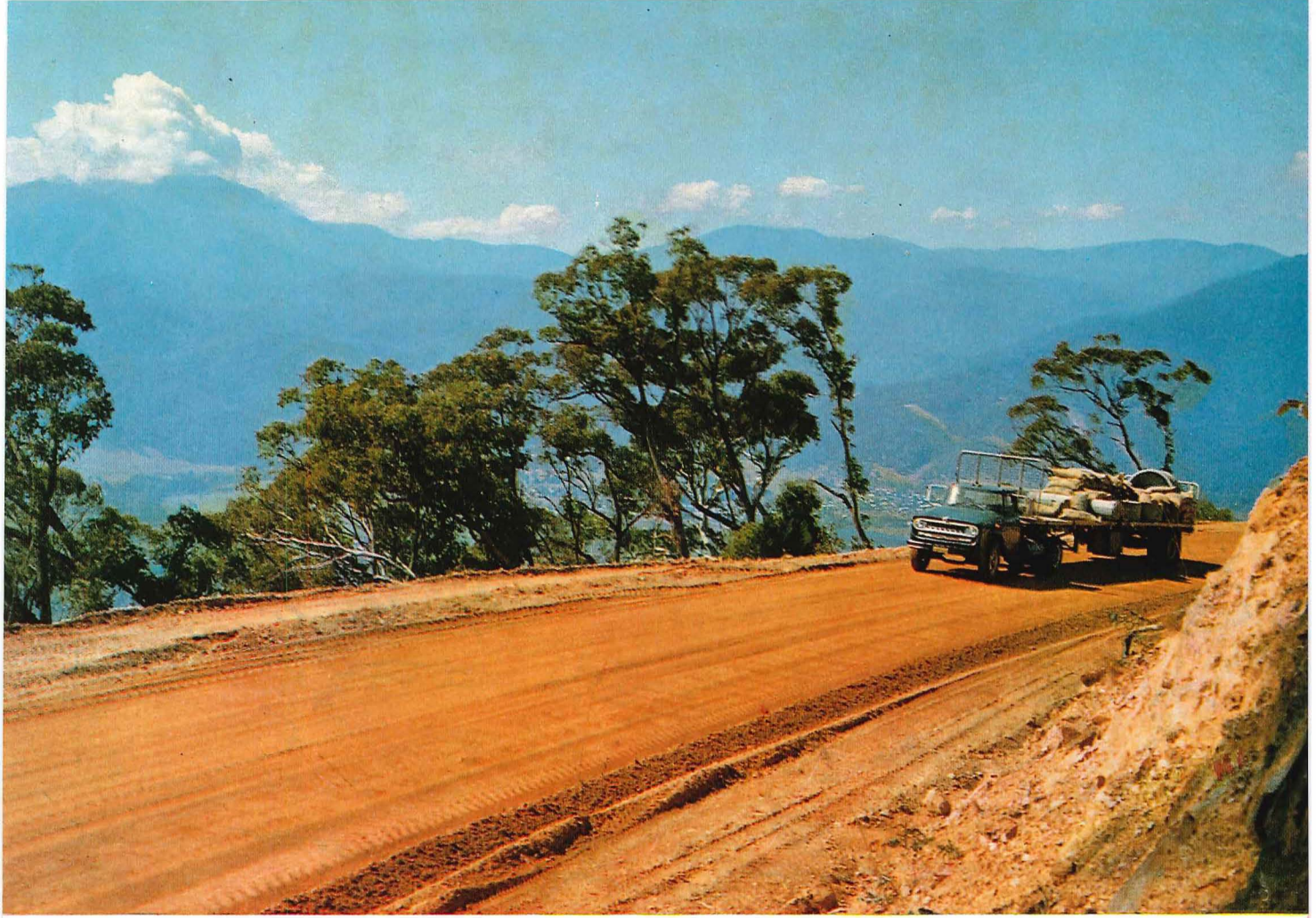
Widening in progress on the Bright - Tawonga Road, Shire of Bright
