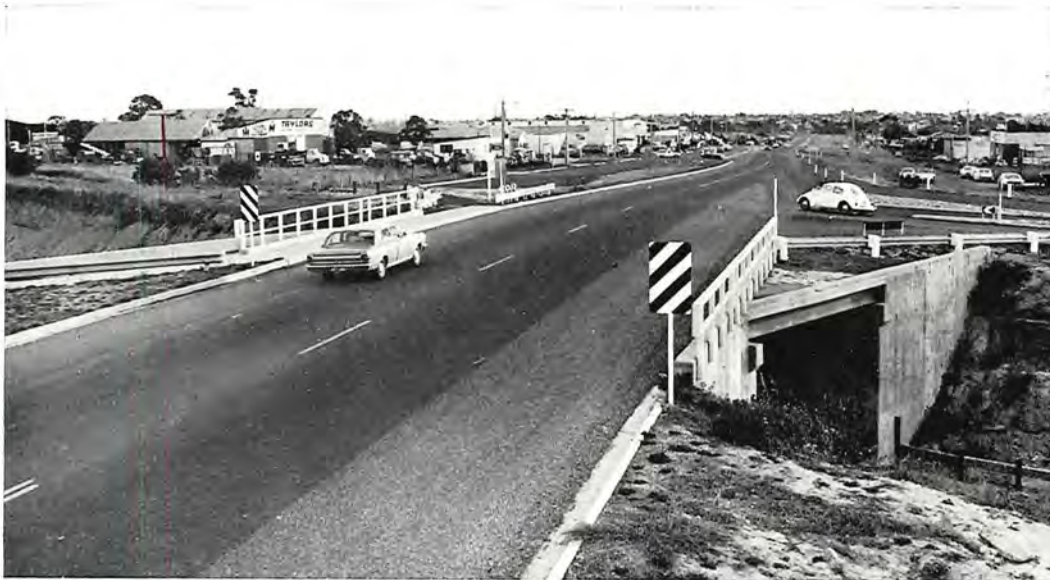
Road over rail bridge replacing the level crossing on the Princes Highway at Traralgon.
