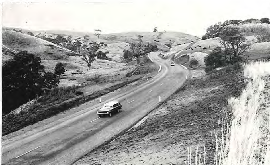
Reconstructed section of the South Gippsland Highway between Bena and Loch.
