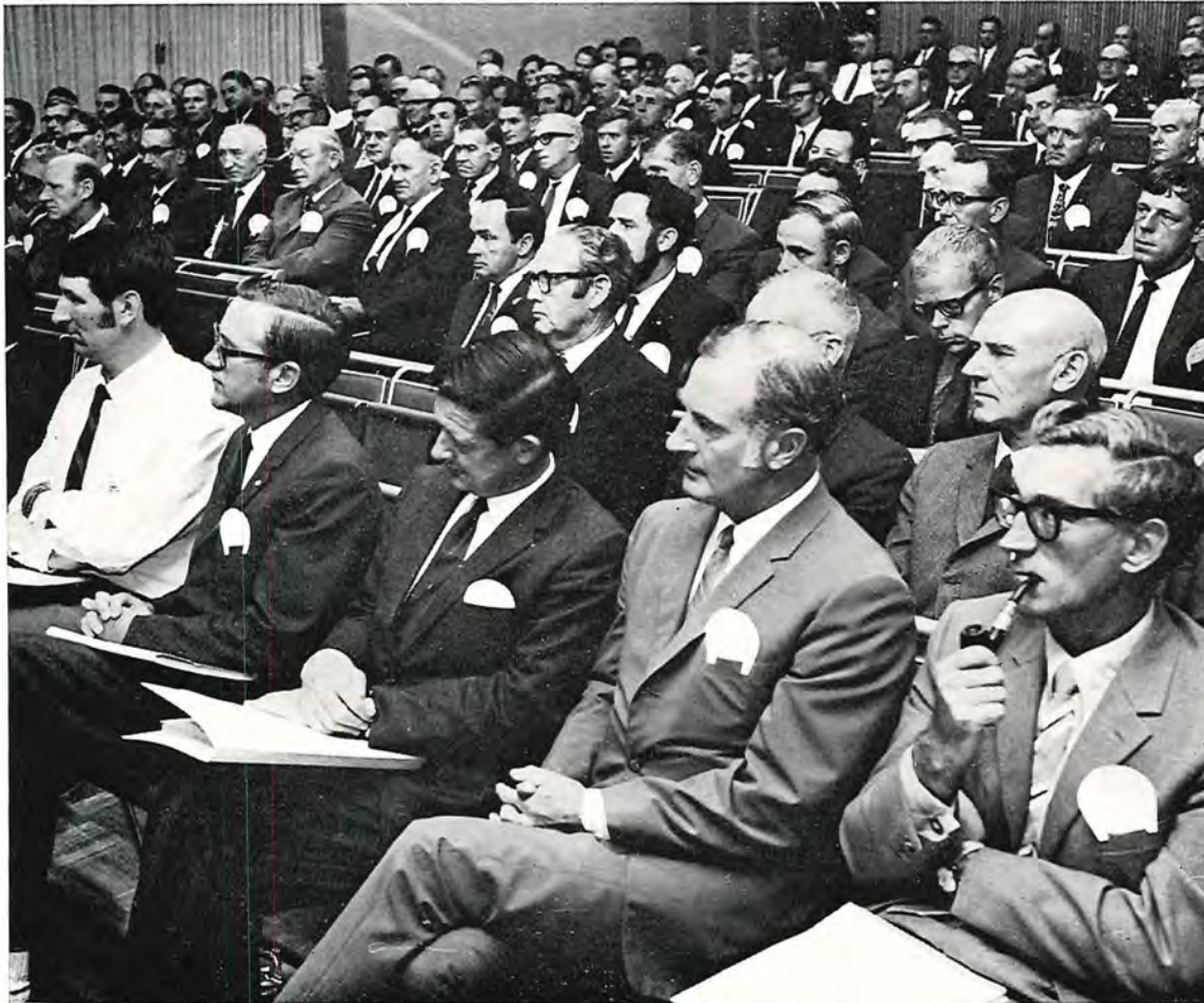
The 27th Conference of Municipal Engineers held at the Board's Head Office in February, 1971.
