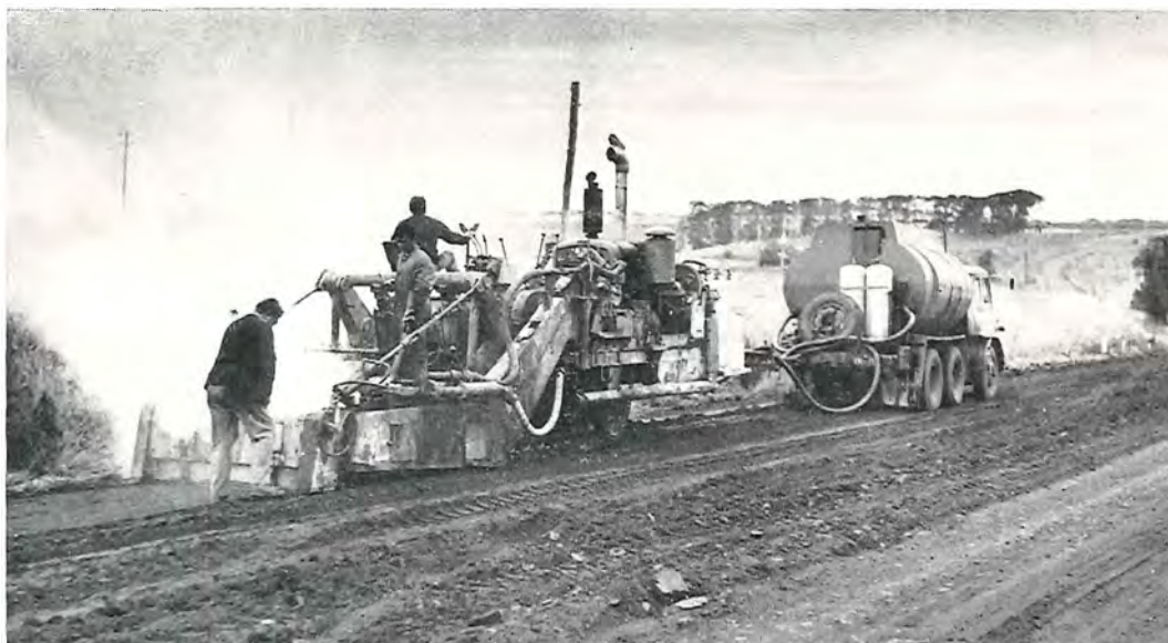
Plate 18—Bitumen stabilization of scoria tuff, Princes Highway West, Warrnambool Division.
