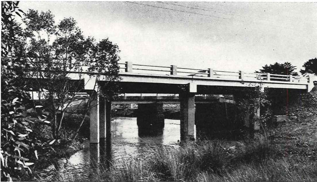
Glenelg Highway — new bridge over Fiery Creek at Streatham.
