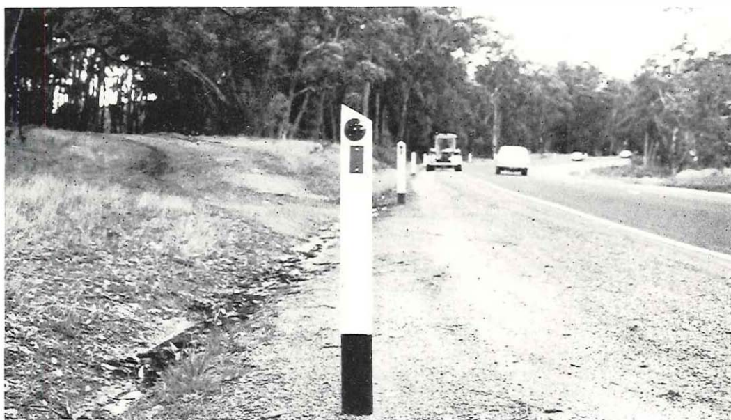
Plate 4—Red corner-cube delineator and red reflective sheeting strip delineator.
