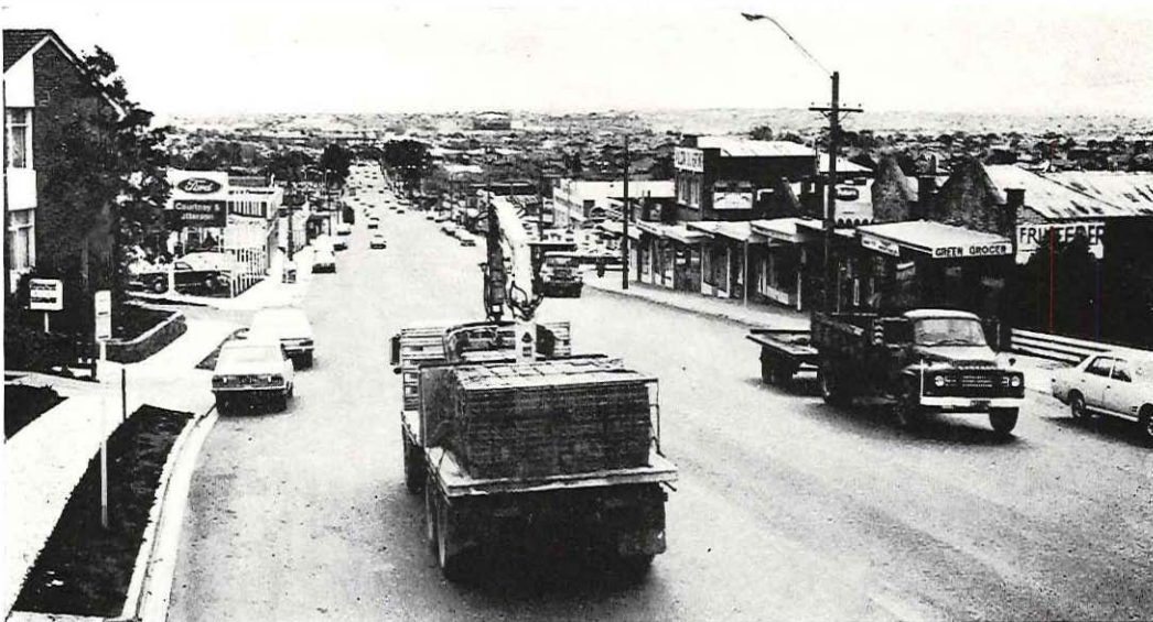
Reconstructed section of Bell Street between Waterdale Road and Upper Heidelberg Road, City of Heidelberg.
