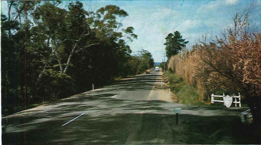
Tyabb-Mornington Road — reconstructed section in Hastings Shire.
