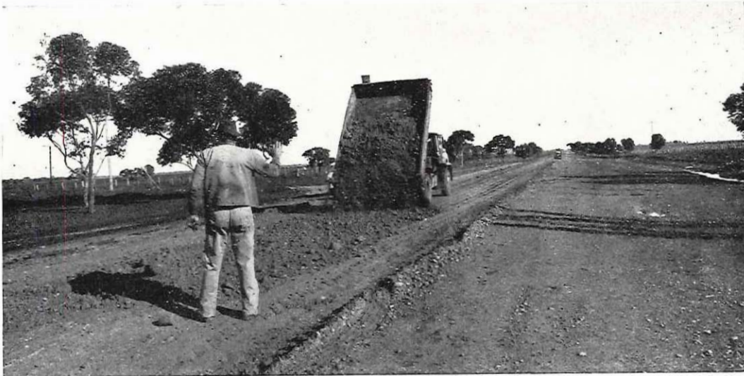
Birchip-Wycheproof Road, Wycheproof Shire — reconstruction in progress west of Wycheproof.
