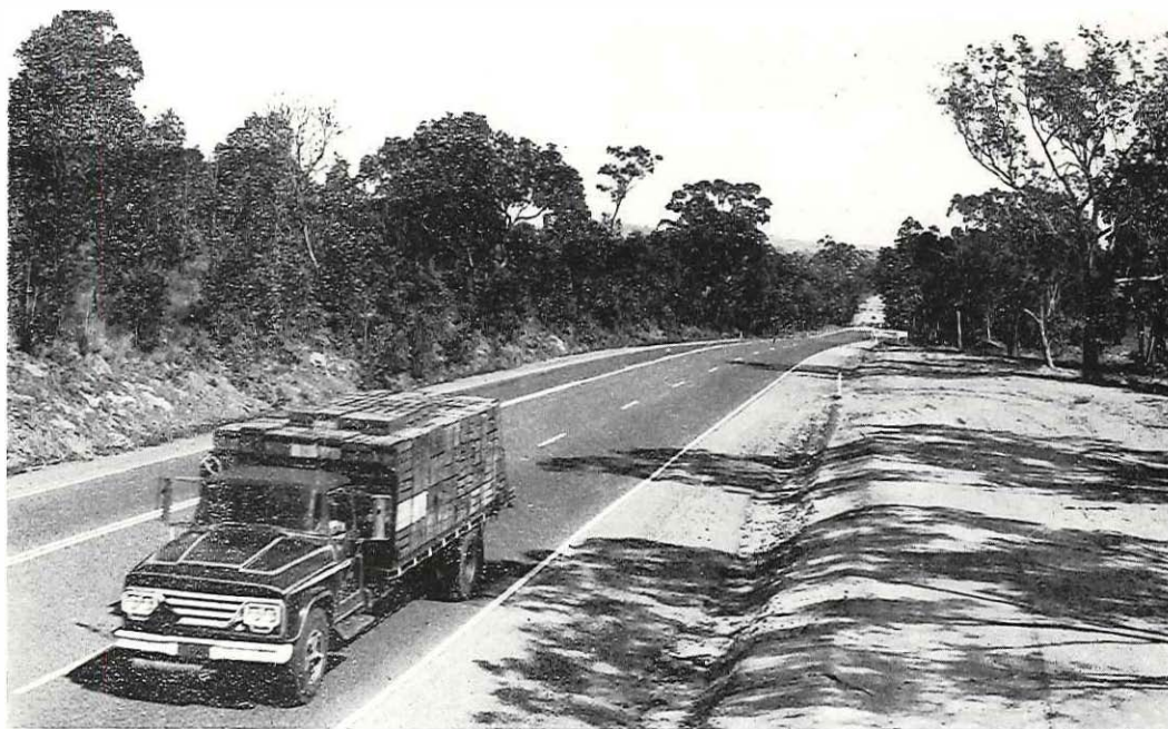
Climbing lane constructed on the Hume Highway at Teneriffe Hill.
