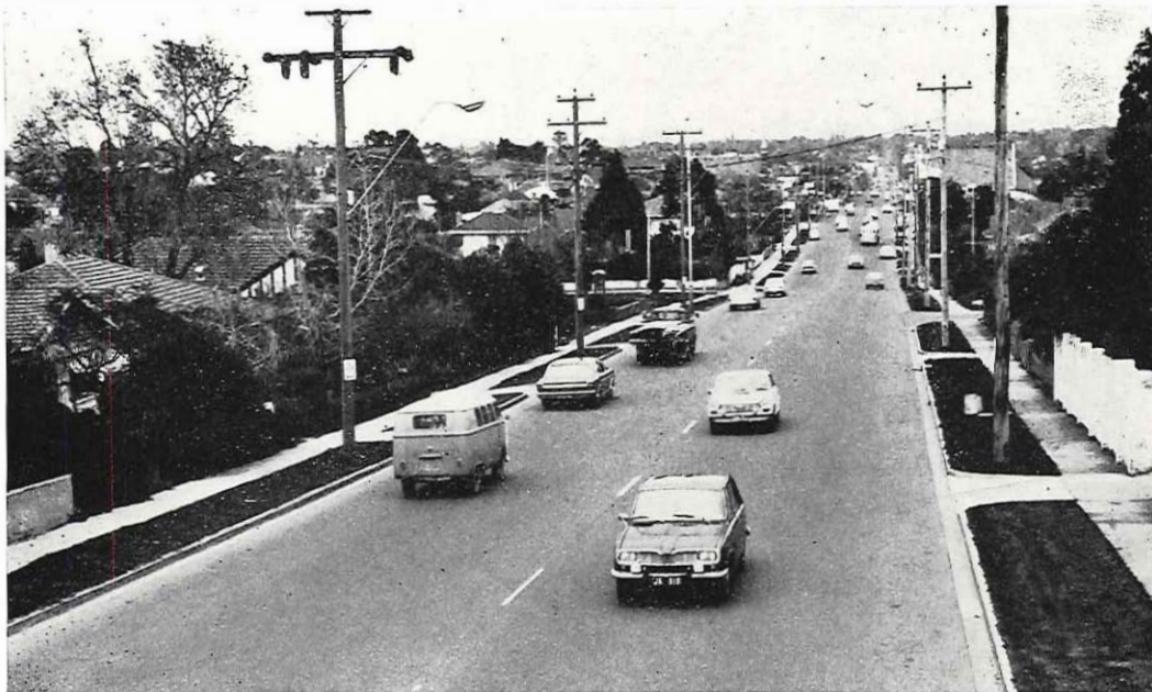
Reconstructed section of Canterbury Road east of Warrigal Road, Box Hill City.
