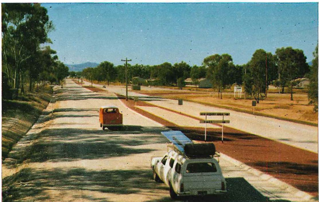
Dual carriageways constructed on the Murray Valley Highway at Bandiana.
