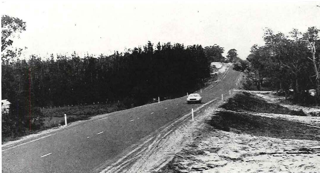
Reconstructed section of the Yarram-Traralgon Road, Alberton Shire.
