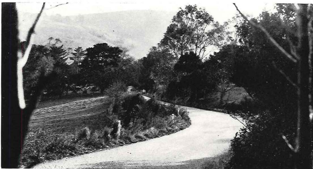
Reconstructed section of Kardella Road, Korumburra Shire.
