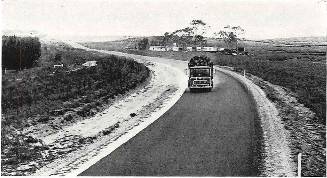
Reconstructed section of the Drik Drik-Nelson Road, Portland Shire.
