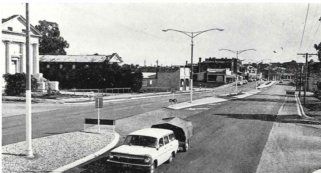
Dual carriageways constructed on the Loddon Valley Highway, Eaglehawk.
