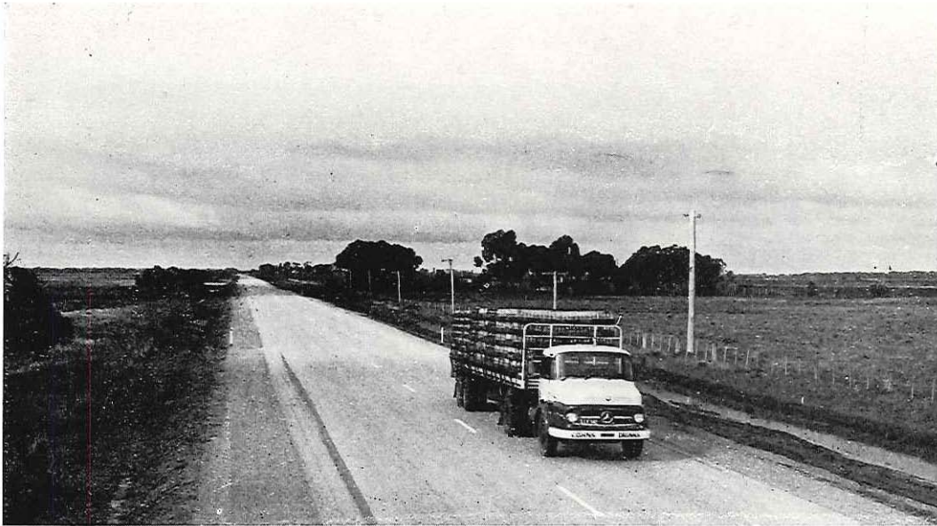
Reconstructed section of the Loddon Valley Highway at Durham Ox.
