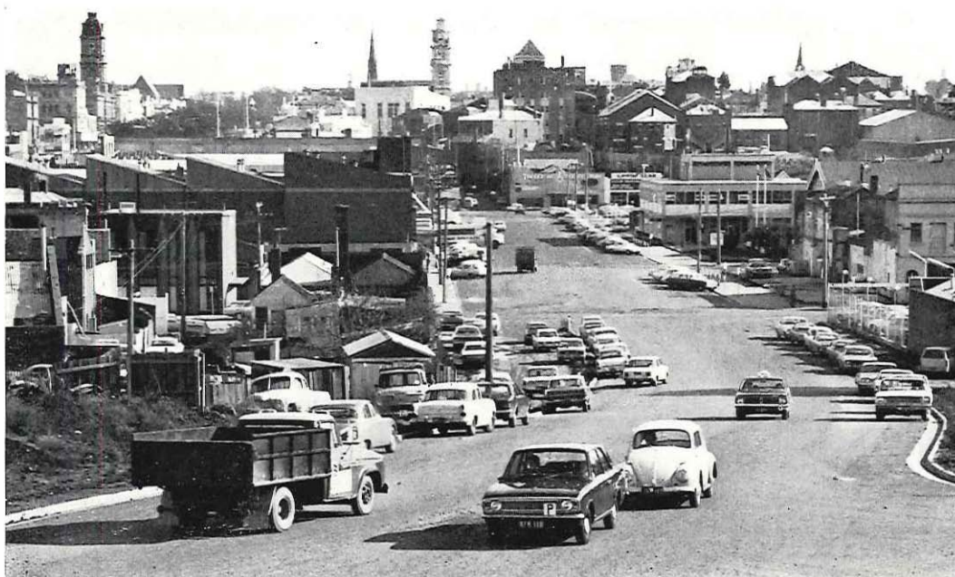
Constructed section of Curtis Street, Ballarat City.
