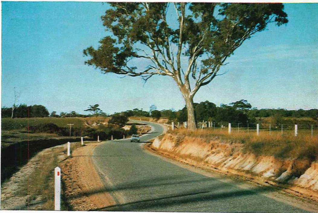
Reconstructed section of the Rosedale-Longford Road (unclassified), Rosedale Shire.
