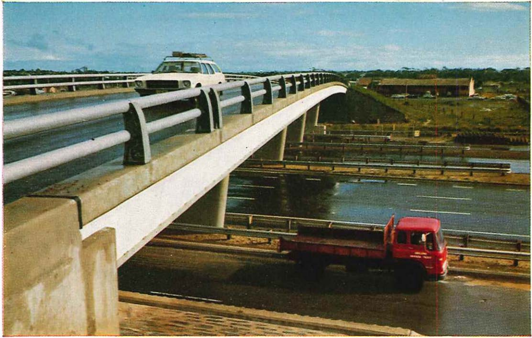
New Margaret Street overpass replacing the level crossing at Victoria Street, Geelong.
