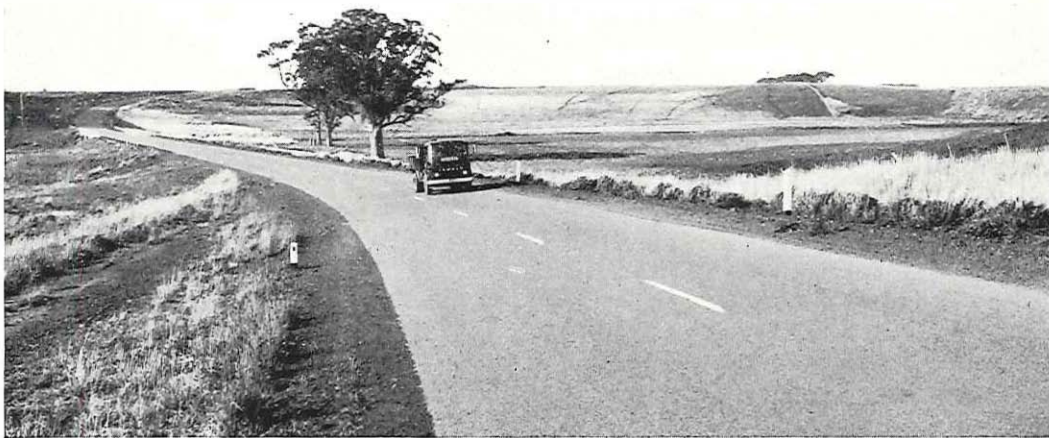
Hamilton Highway — reconstructed section east of Duverney.
