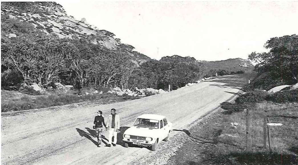
Reconstructed section of Mount Buffalo Road.
