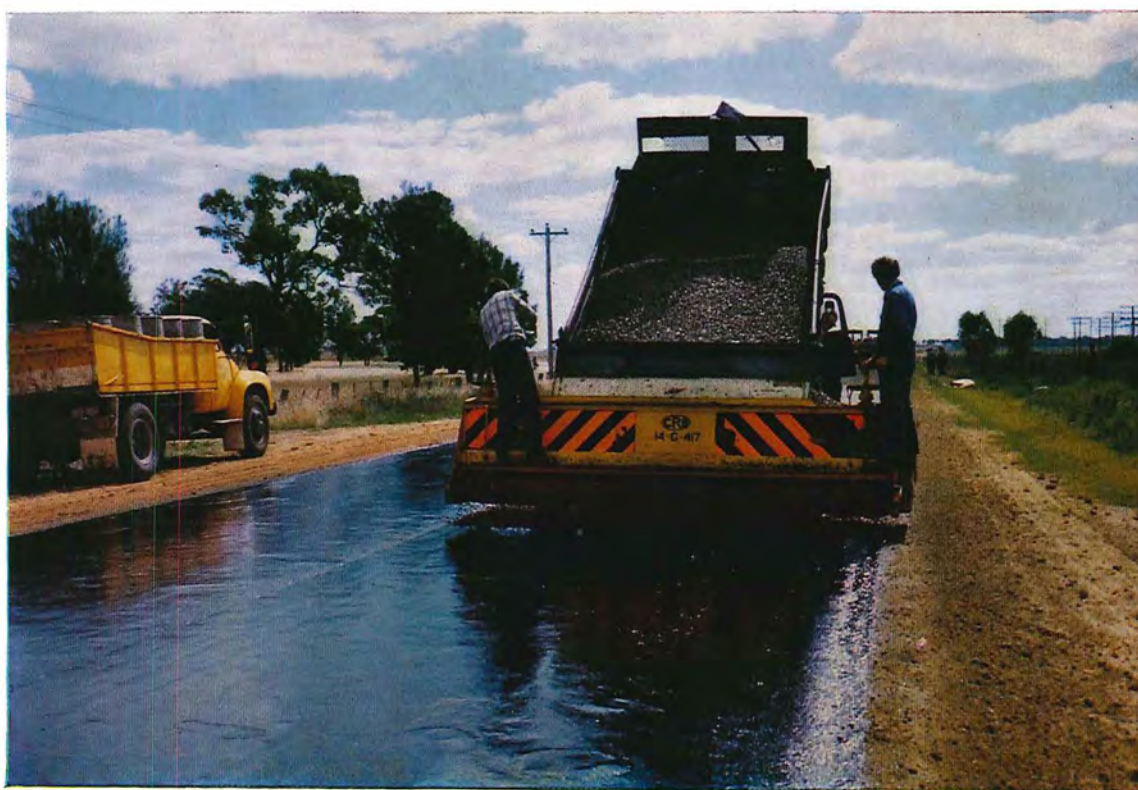
Spreading aggregate on a sprayed bitumen binder.
