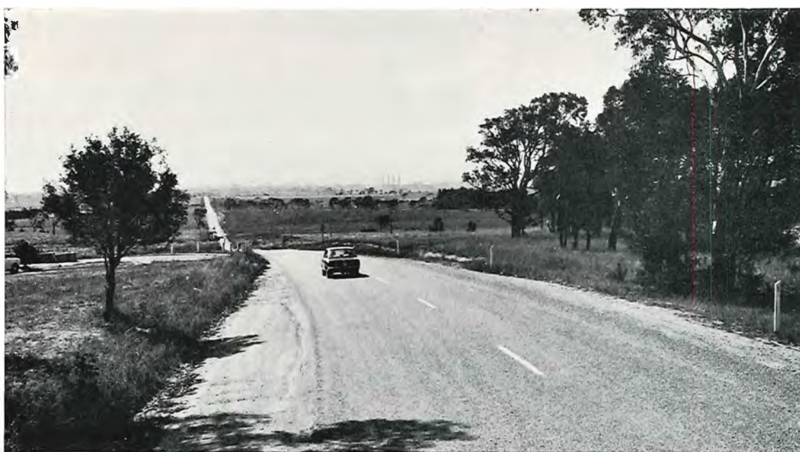
New construction on the Midland Highway deviation south of Morwell.
