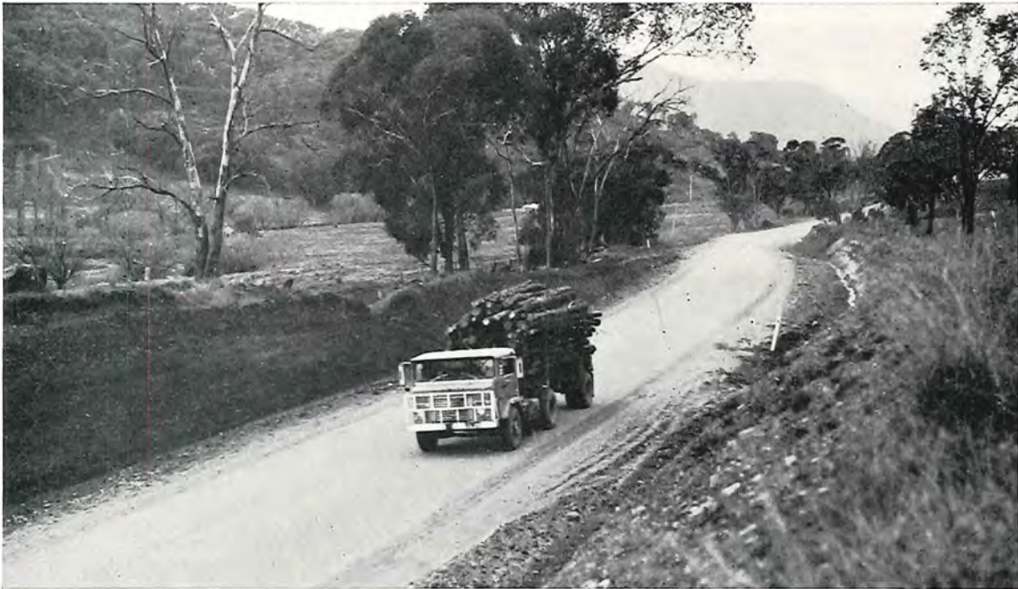
Reconstructed section of Happy Valley Road, Shire of Myrtleford.
