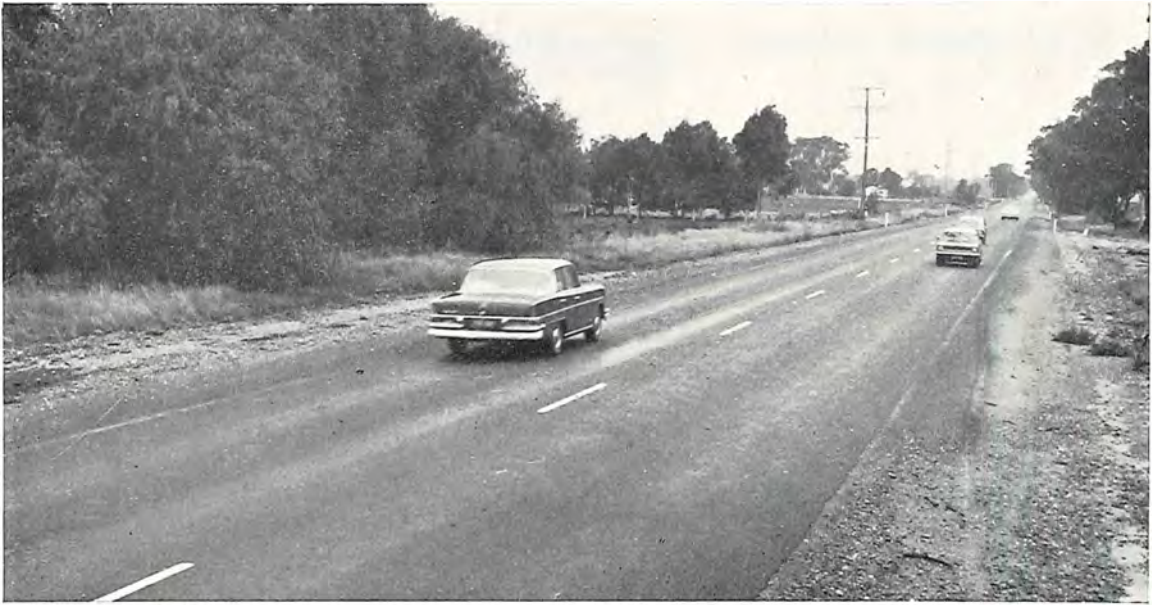
Reconstructed section of Boort-Kerang Road, Shire of Gordon.
