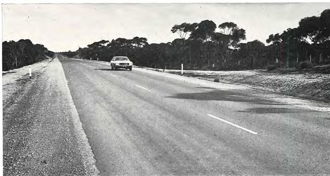
Reconstructed section of the Calder Highway north of Ouyen.
