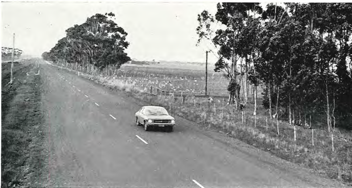
Hamilton Highway—reconstructed east of Lismore.
