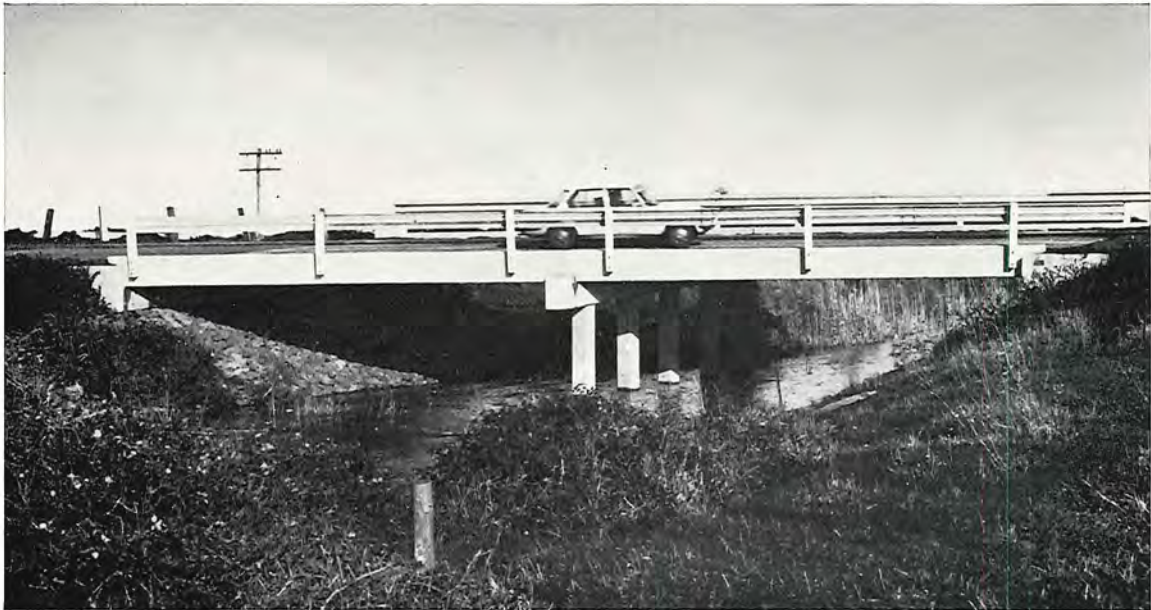
St. Helens Road bridge over Shaw River, Shire of Belfast.
