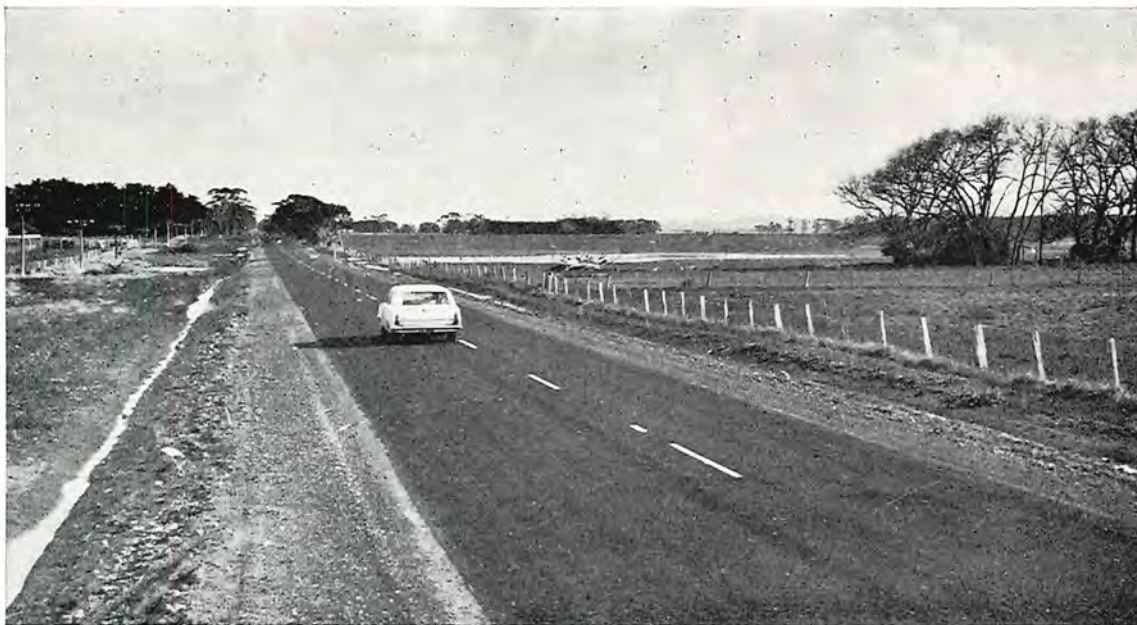
Reconstructed section of Woolsthorpe-Heywood Road, Shire of Portland.
