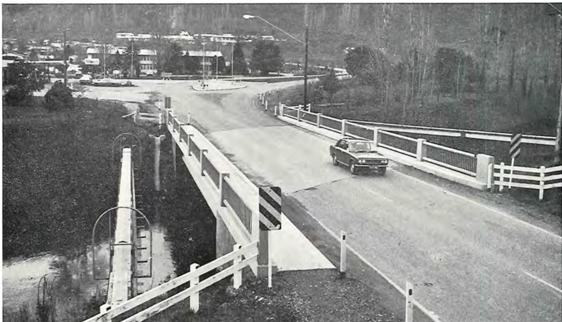
Bogong High Plains Road—bridge over Tail Race Channel, Mt. Beauty.
