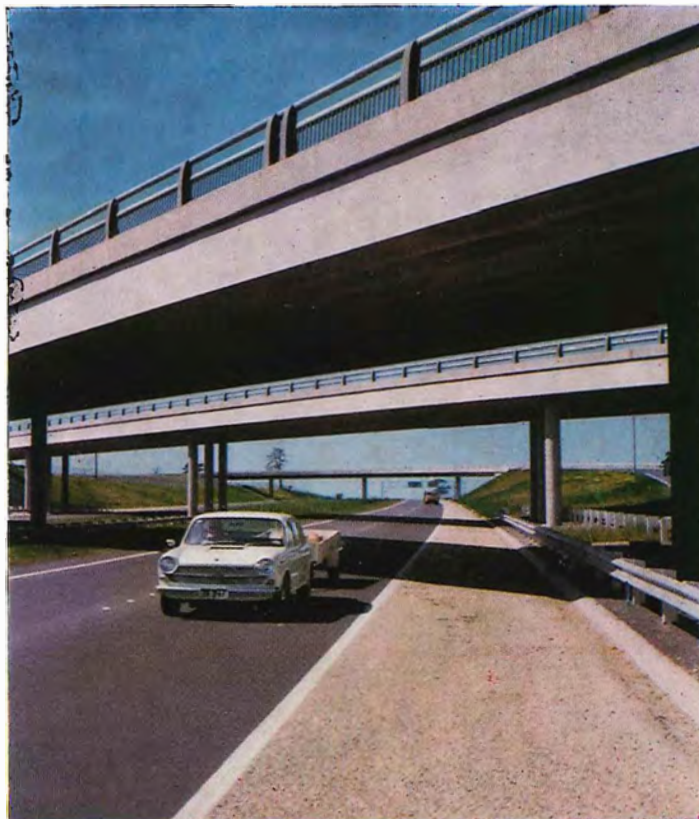
The Mulgrave Freeway at the Wellington Road interchange.
