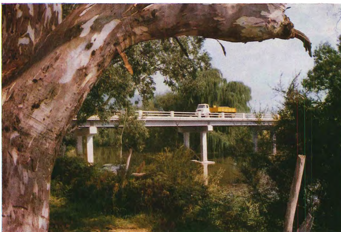
Bridge over the Mitta Mitta River, Dartmouth Road, Shire of Tallangatta.
