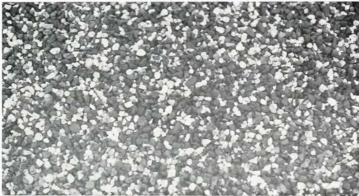
Plate 6—Close up view of scoria/calcined pyrophyllite mix surface seal.
