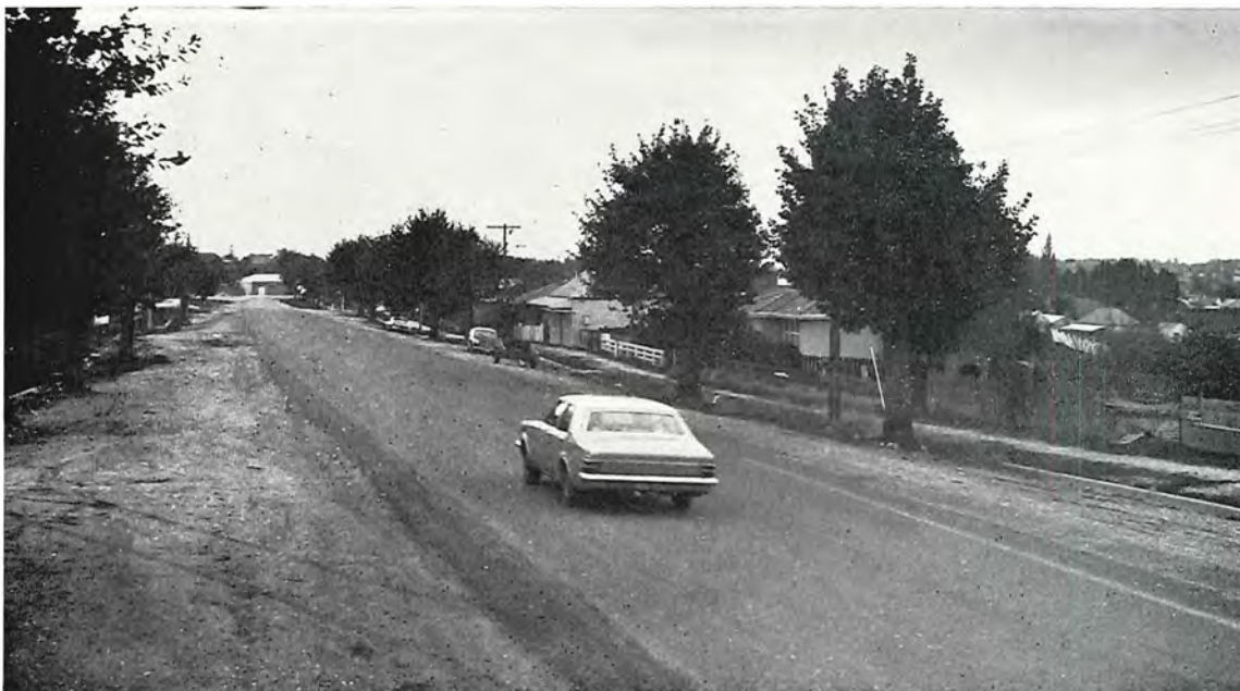
Reconstructed section of Creswick-Dean Road, Shire of Creswick.
