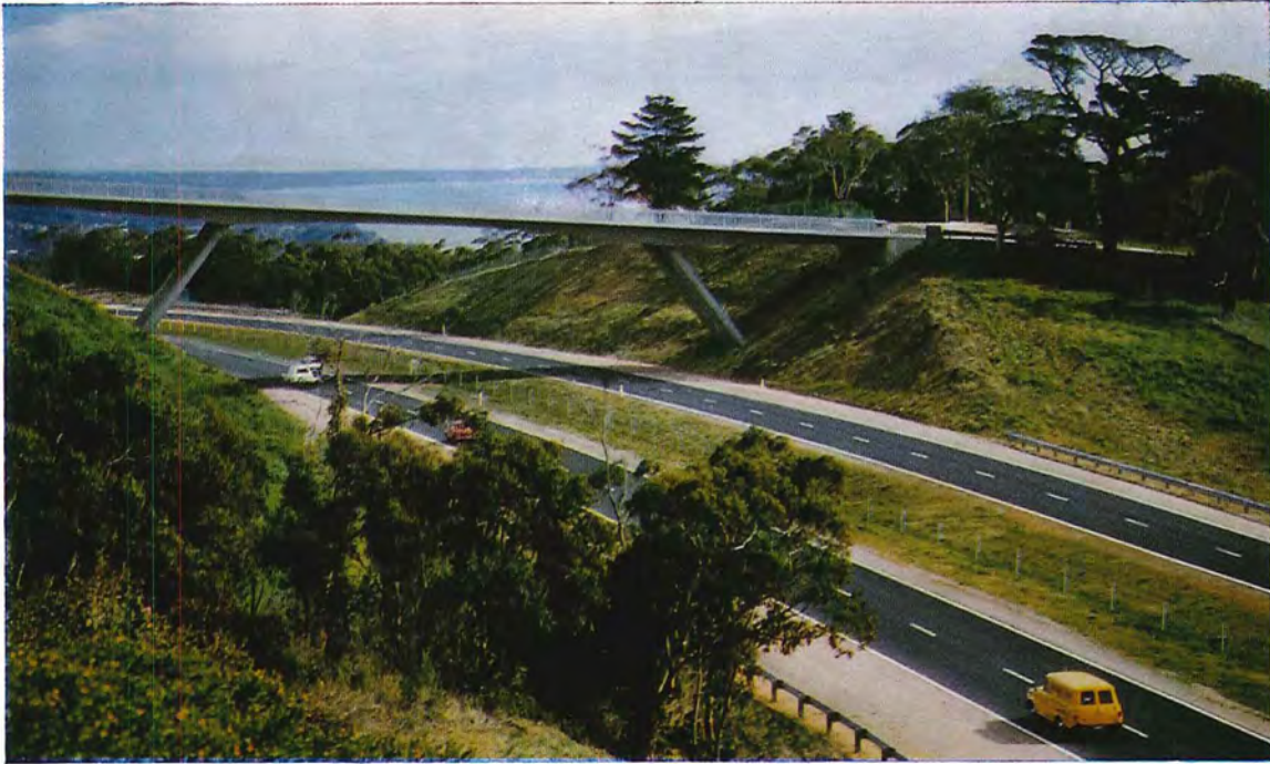
The Burrell Road bridge, Mornington Peninsula Freeway.
