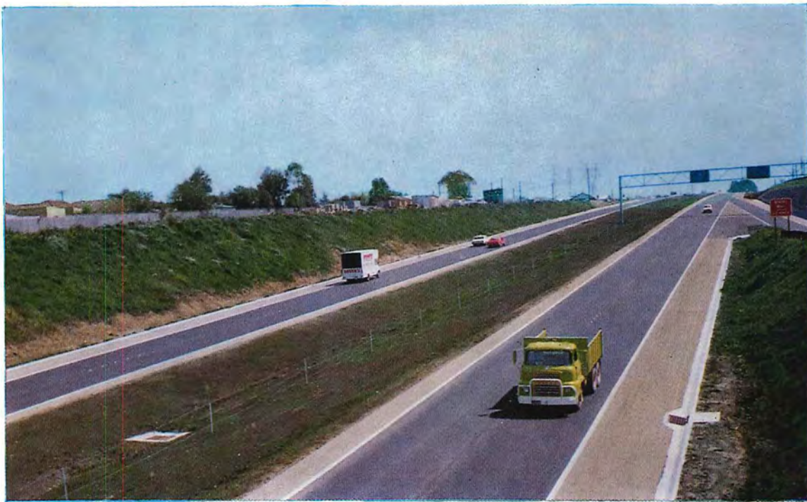
New section of the Calder Freeway at Keilor East.
