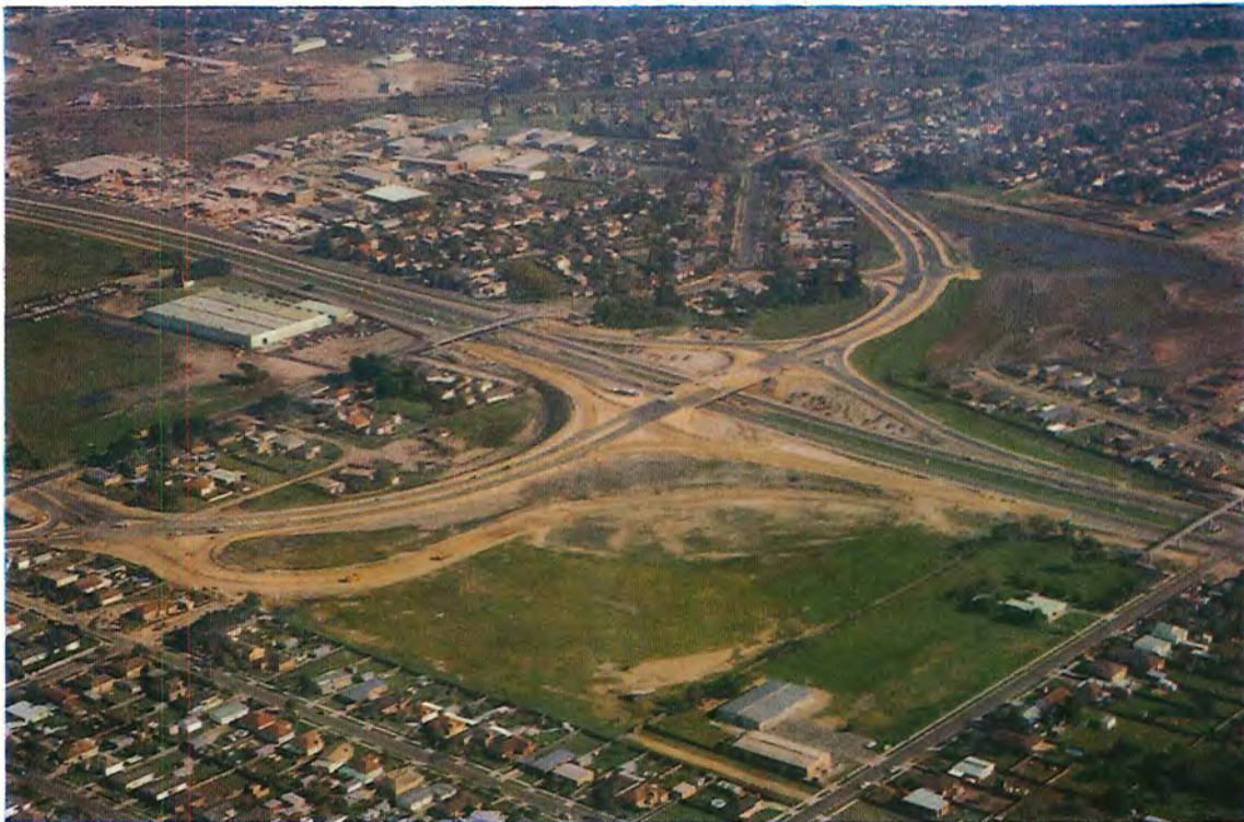
Seaford Road overpass of the Frankston Freeway during construction.
