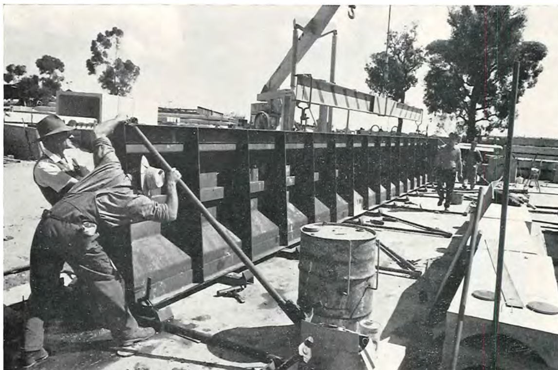
Plate 1—Setting up I-beam form.
