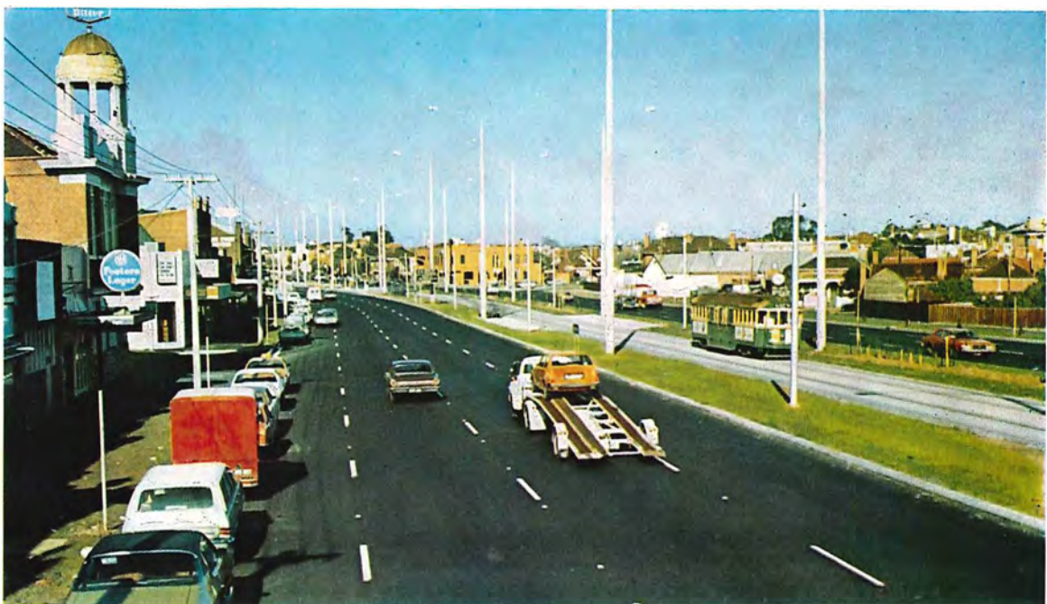
Widened and reconstructed section of High Street, St Kilda.
