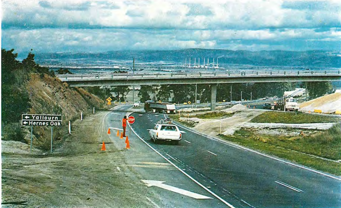
The Hernes Oak interchange bridge over the Princes Freeway (Haunted Hills Section).
