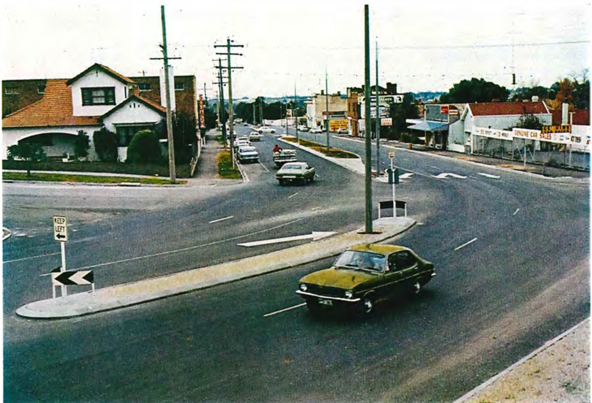
Reconstructed section of the Calder Highway providing dual carriageways in Bendigo City.
