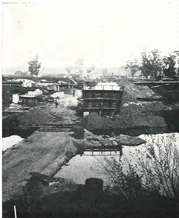
Plate 2—Construction of land piers for the main river bridge.
