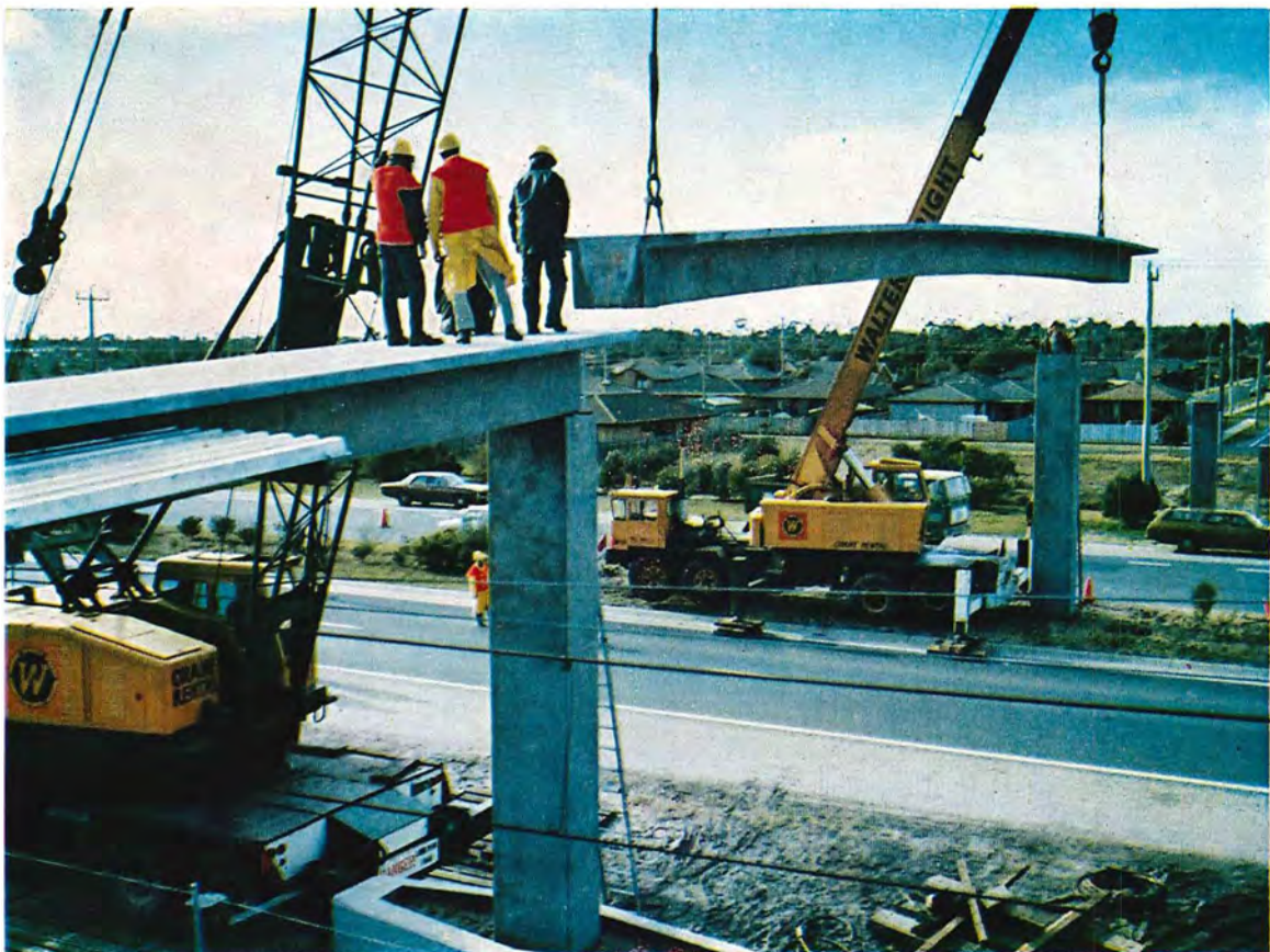
Pedestrian overpass, Frankston Freeway, during construction.
