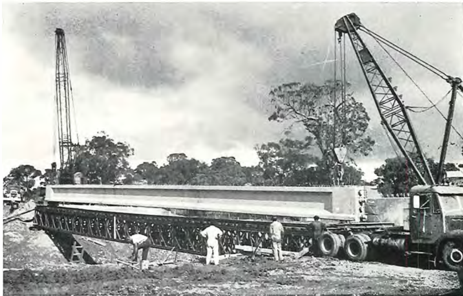
Plate 1—Launching a beam across the temporary Bailey bridge.
