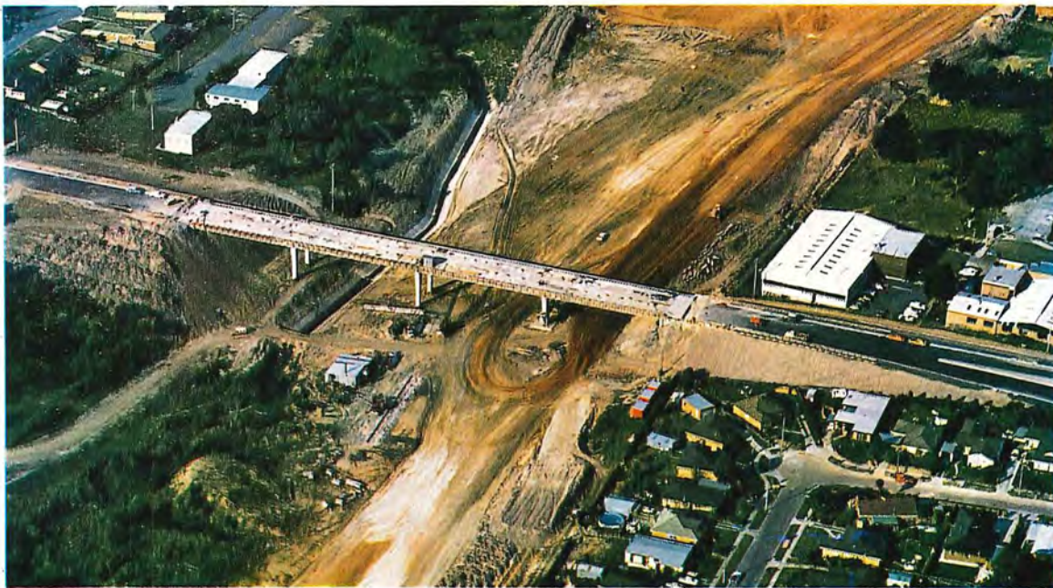
Bridge over the Mulgrave Freeway at Stephenson's Road.
