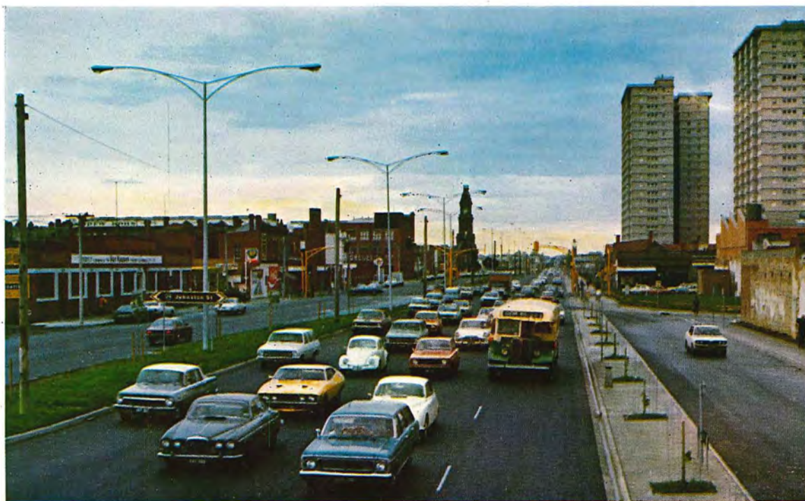
Dual carriageways provided on Hoddle Street, Collingwood.
