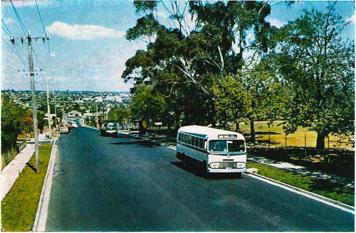
Station Street, Box Hill South, reconstructed by the Box Hill City Council with financial assistance from the Board.
