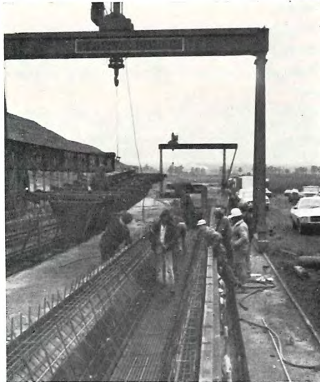
Plate 5—Beam formed with tendons and reinforcing placed ready for casting.
