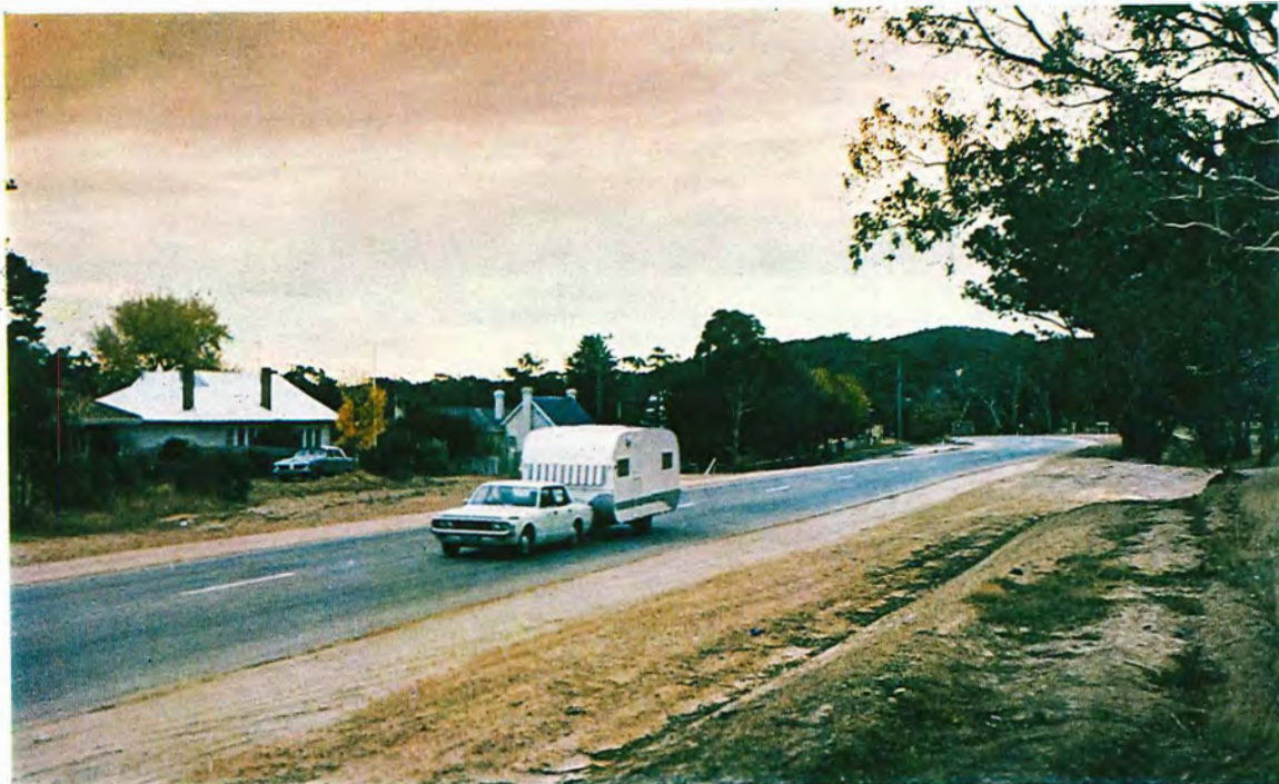
Reconstructed and realigned section of the Goulburn Valley Highway between Trawool and Kerrisdale.
