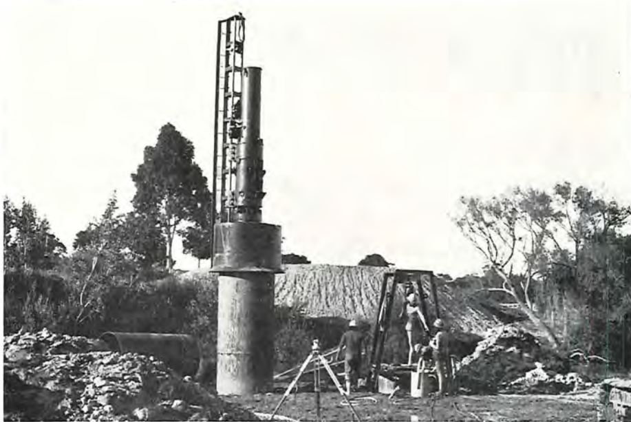
Plate 4—Kobe K32 diesel hammer with steel driving plate bellmouth and mast leaders attached.
