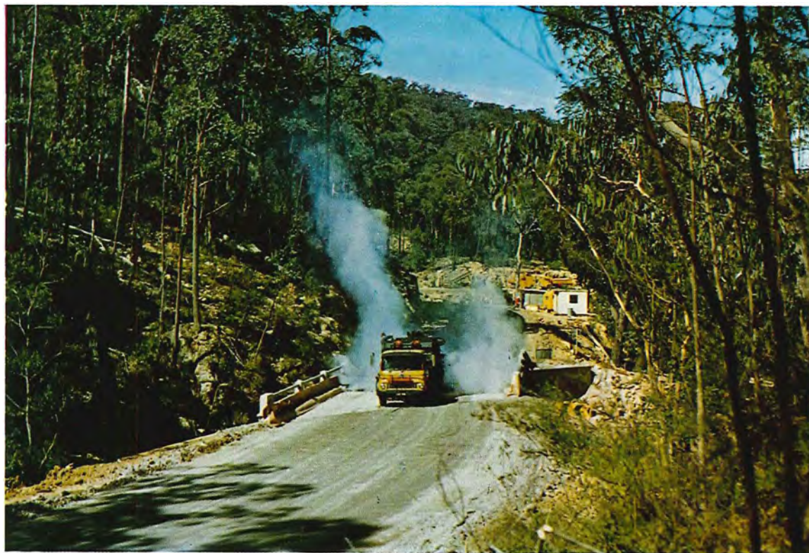
Sealing the deck of the new bridge over Wattle Tree Creek on the Gelantipy Road, Tambo Shire.
