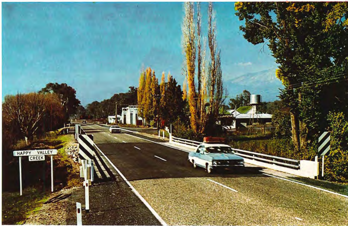
New reinforced concrete bridge on the Ovens Highway at Happy Valley Creek.
