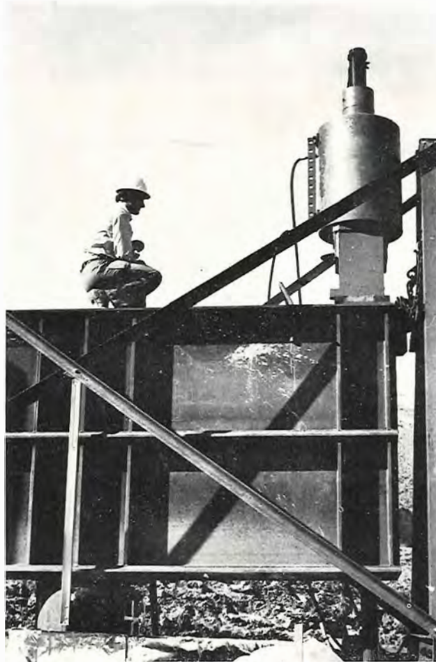
Plate 7—Pile Load Testing in Progress. 5000 kN anchor cables were tensioned against a reaction beam to load the test piles.
