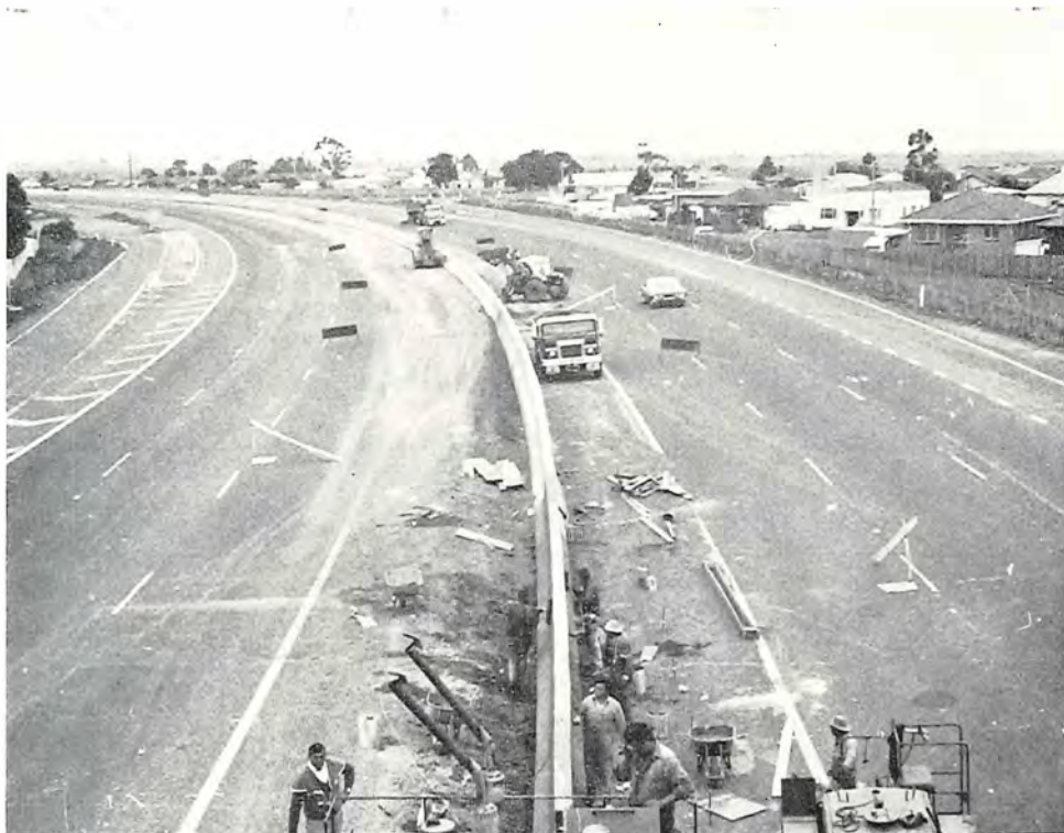
Plate 28—View showing new work in progress on Princes Freeway at Laverton.
