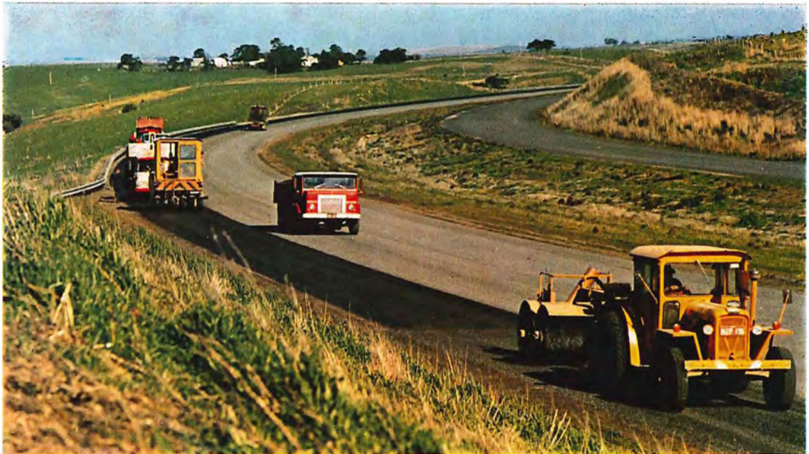
Work in progress on the Western Freeway (Myrning Section).
