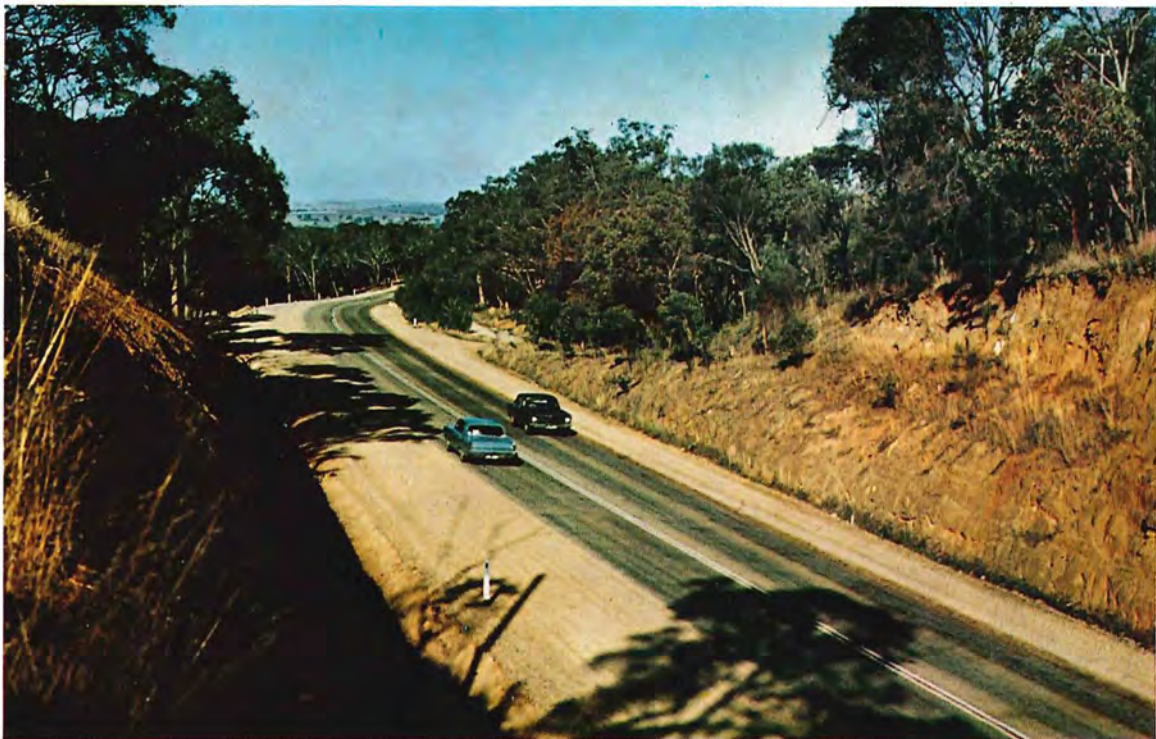
The Ballan-Daylesford Road, reconstructed in the Shire of Ballan.
