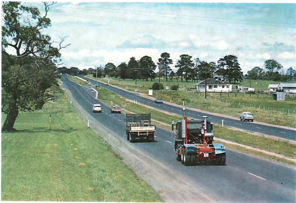
Dual carriageways constructed on the South Gippsland Highway.
