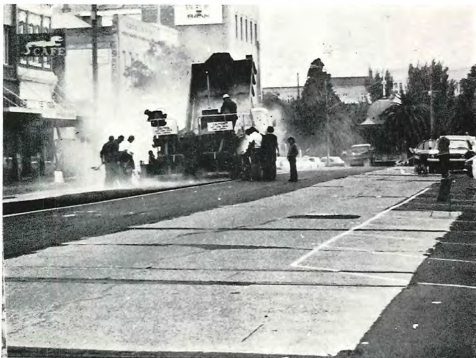
Plate 19—Malop Street—Geelong Placing special asphalt mix over old concrete pavement
