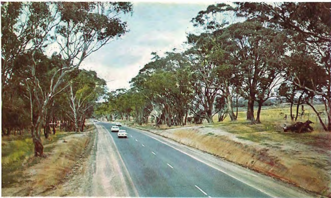
Reconstructed section of the Calder Highway south of Ravenswood.
