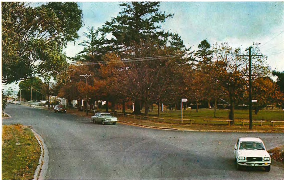
Eureka Street, Ballarat City, reconstructed with financial assistance from the Board.
