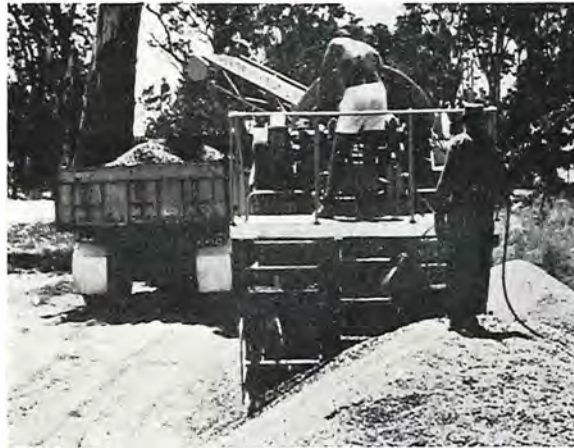
Plate 25—Old method of precoating using hand held spraying lance.
