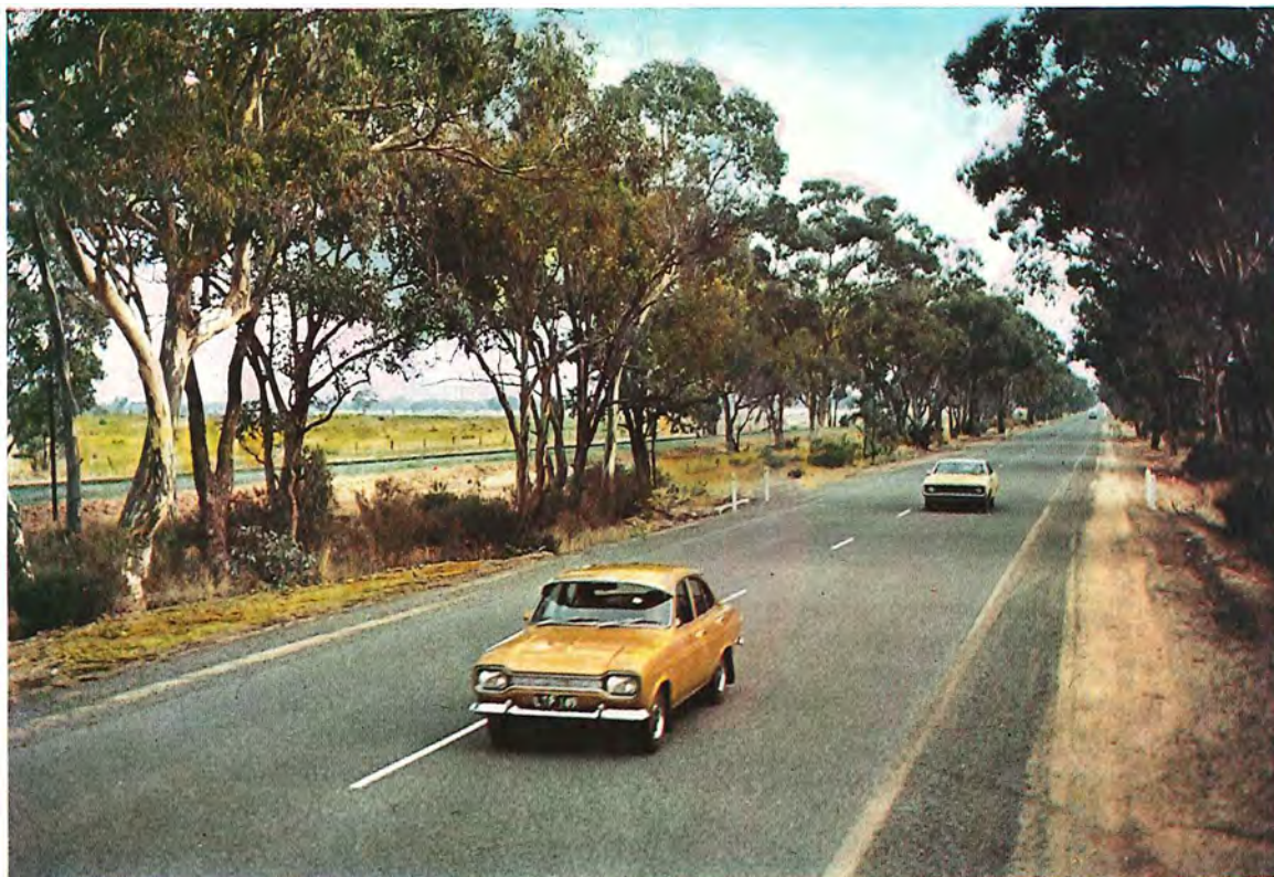
Section of the Calder Highway reconstructed near Kurting, between Bendigo and Charlton.
