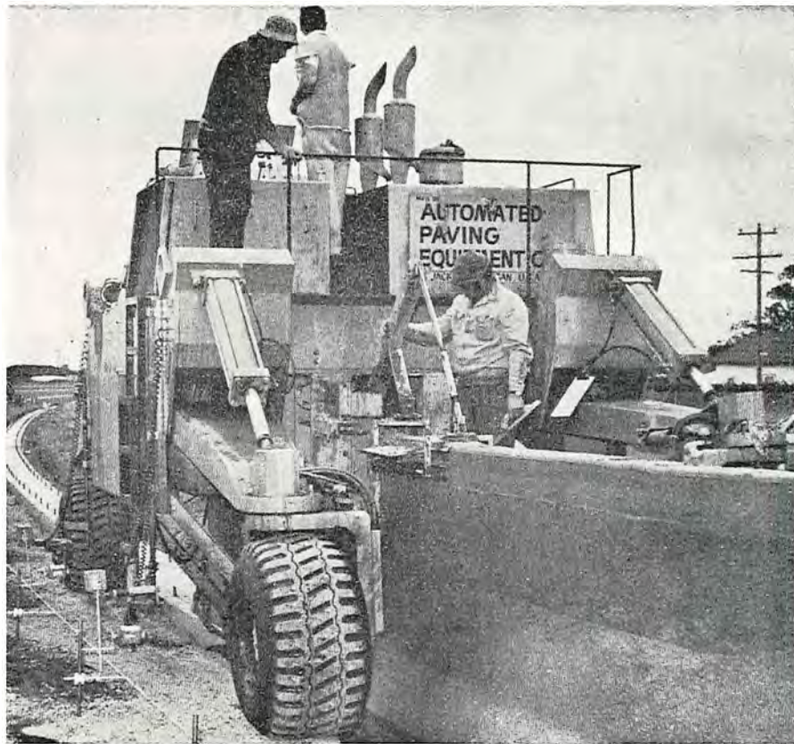
Plate 27—Showing extrusion in progress. Note sensor units against string line on left of machine
