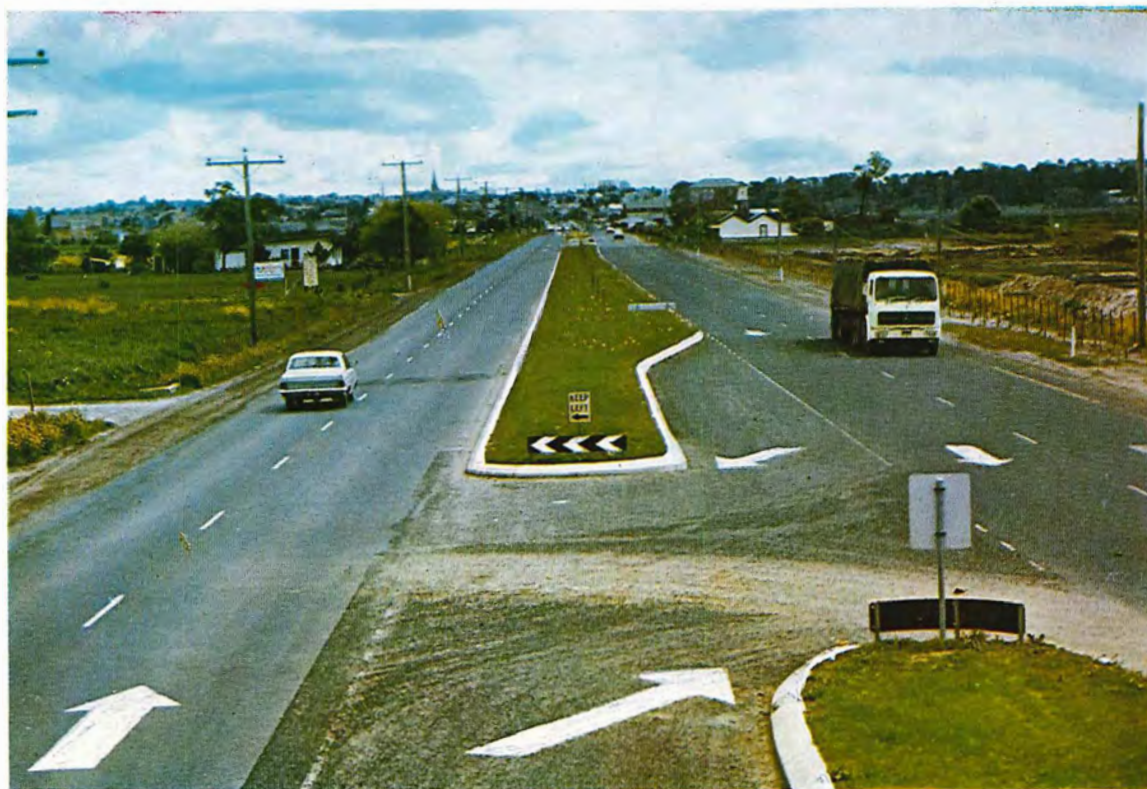
Dual carriageways constructed on the Geelong-Portarlington Road by the Bellarine Shire Council.
