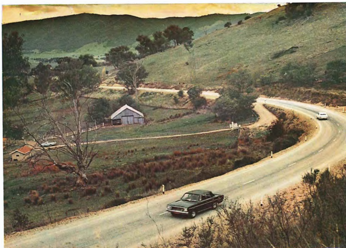
The Omeo Highway, reconstructed north of Noorungong.
