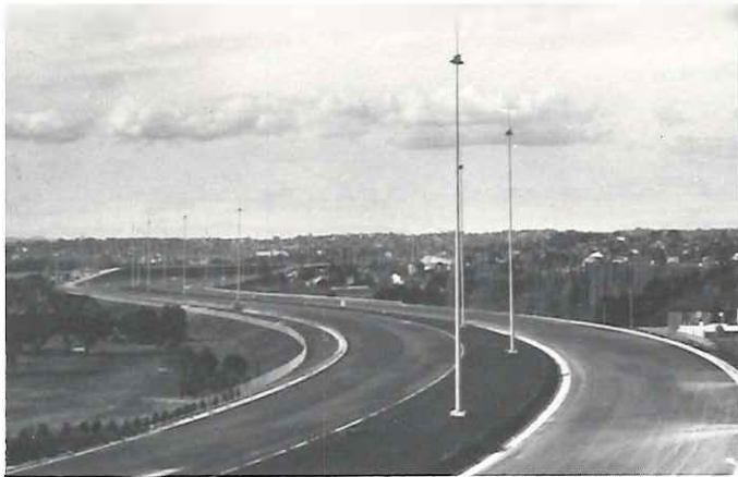
Plate 13: High mast lighting installation on the Eastern Freeway.
