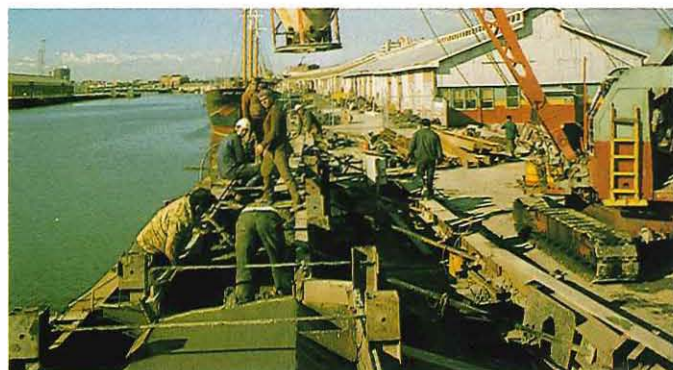
Johnson Street Bridge, South Melbourne.
