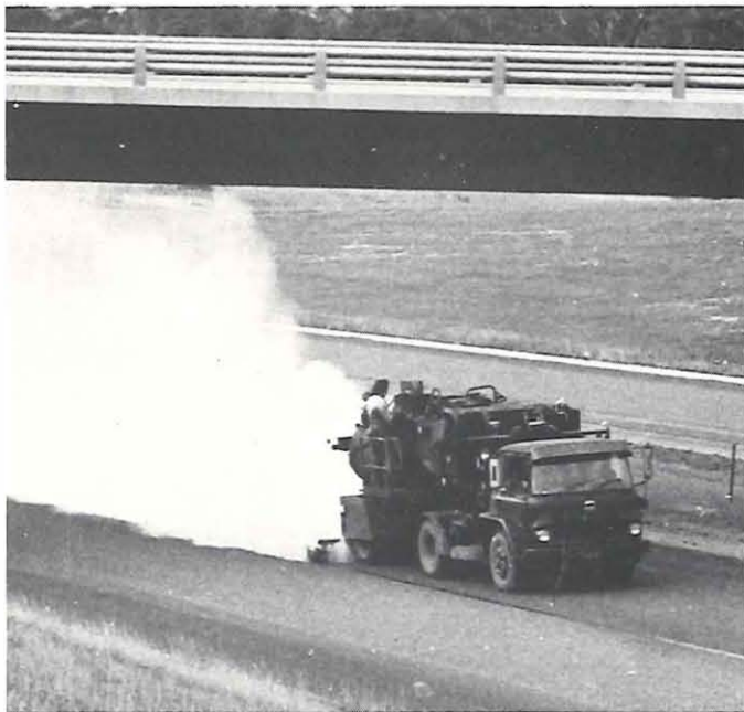
Plate 17: Hume Freeway—Wallan to Broadford. General view of sealing in progress.
