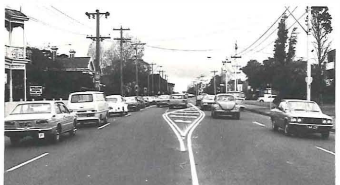
Plate 11: View of improved, Barkers Road/Denmark Street intersection looking east along Barkers Road.
