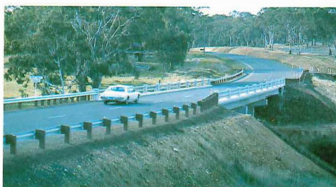
New bridge over Bet Bet Creek, Pyrenees Highway.
