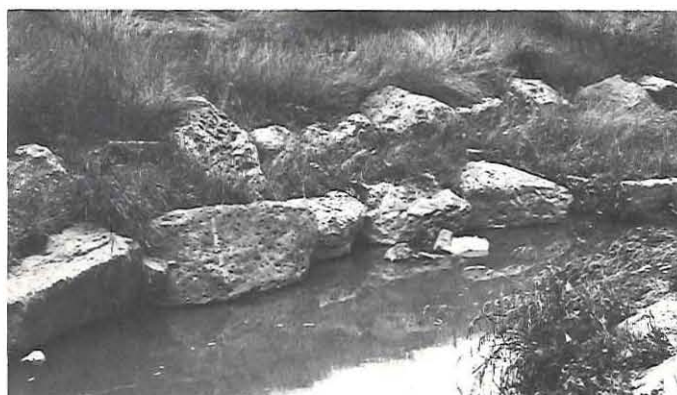
Plate 16: Erosion control treatment on the banks of Glass Creek.
