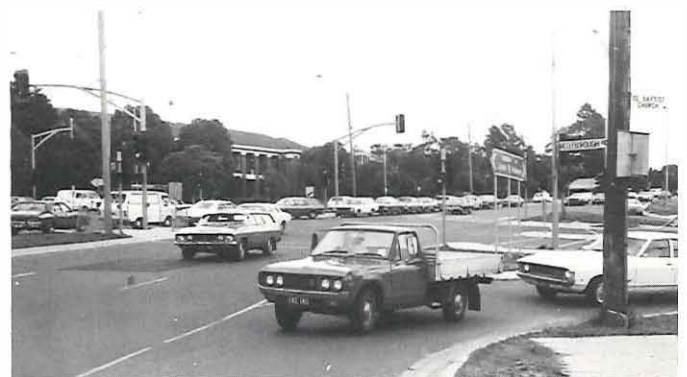
Plate 10: Maroondah Highway—Middleborough Road improvements.
