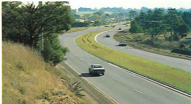
Duplication east of Beaconsfield on the Princes Highway East.
