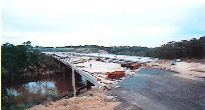
Eastern Freeway-Yarra River Bridge.
