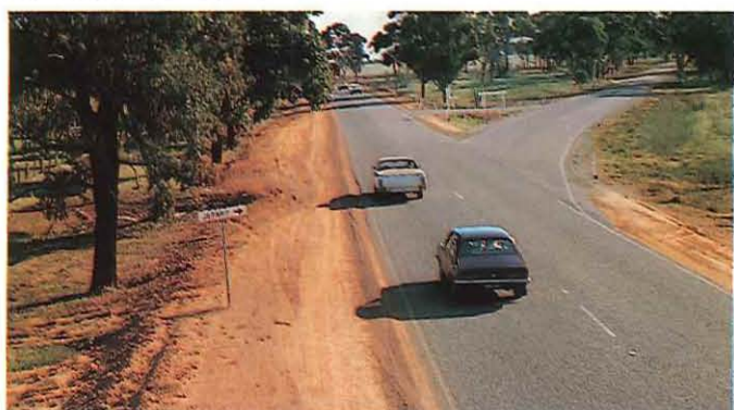
Highways — Western Highway, near Dimboola
