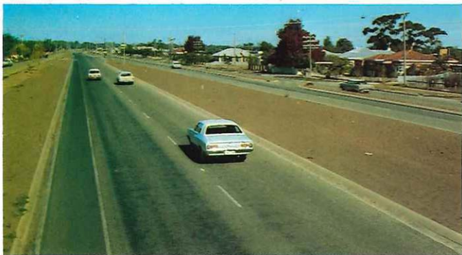
Duplication of the Western Highway, Horsham.
