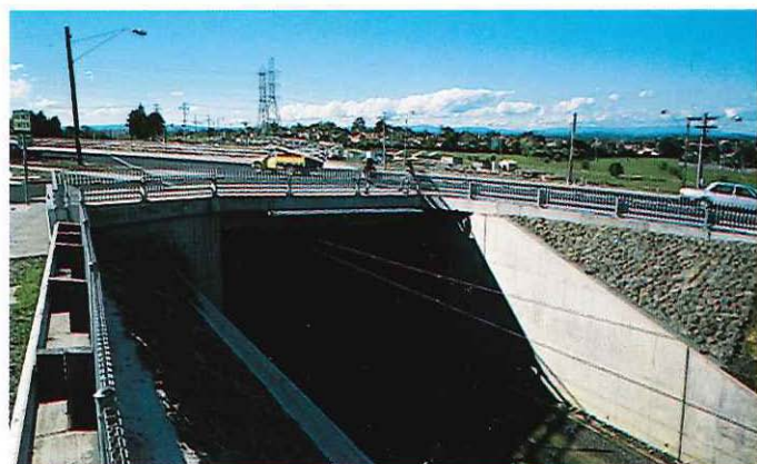
Greensborough Freeway — Watsonia Road overpass.
