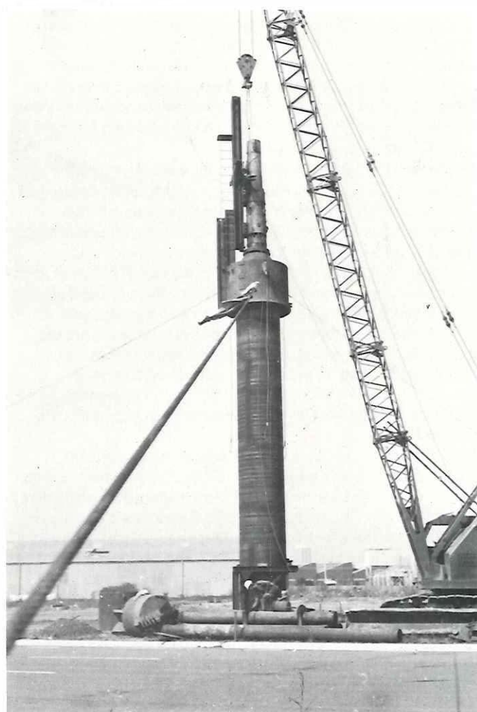
Plate 7: Driving 1500 mm steel casings for bored piles at Johnson Street, South Melbourne
