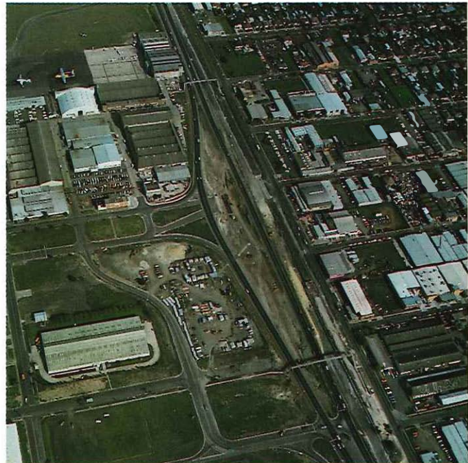
Tullamarine Freeway — upgrading Lancefield Road adjacent to the Essendon Airport.
