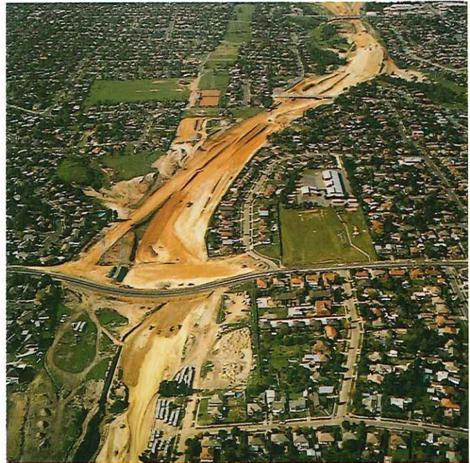
Mulgrave Freeway — under construction between Warrigal Road and Forster Road.
