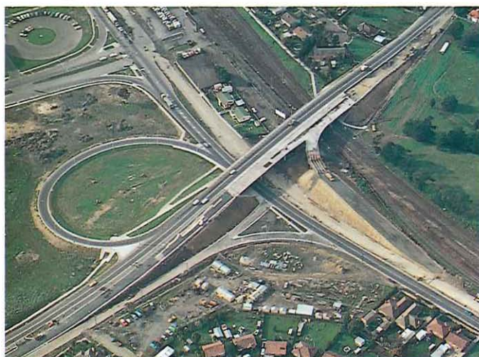
Camp Road, Broadmeadows — elimination of railway level crossing.
