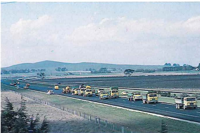
Hume Freeway — asphalt paving south of Wandong.
