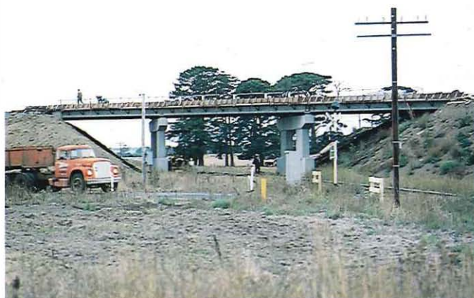
Princes Highway — road over rail overpass under construction at Weerite.
