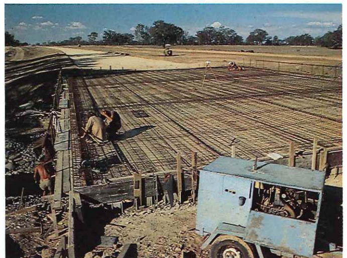
Hume Freeway, Violet Town Bypass — bridge over Honeysuckle Creek.
