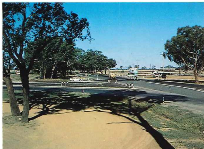
Murray Valley Highway — Benalla-Tocumwal Road intersection.
