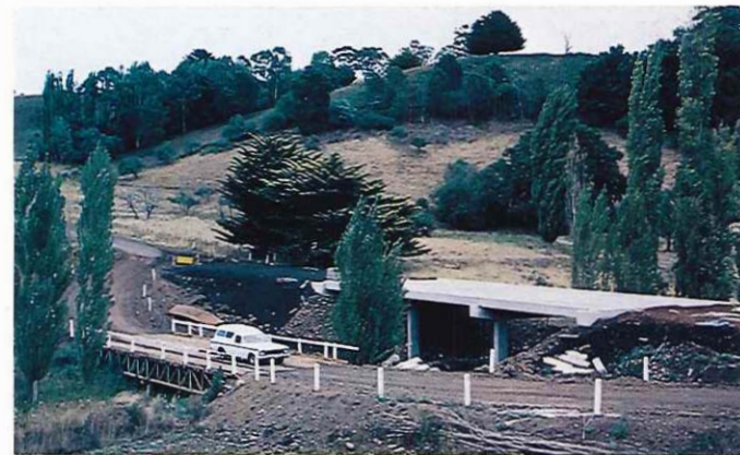
Cobden-Port Campbell Road, Shire of Heytesbury — construction of bridge across Curdies River.
