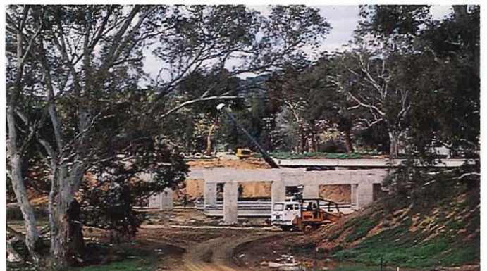
Hume Freeway, Seymour to Avenel Section — bridges over Hughes Creek.
