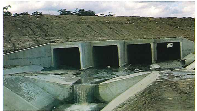
Mulgrave Freeway — Scotchman's Creek Culvert.
