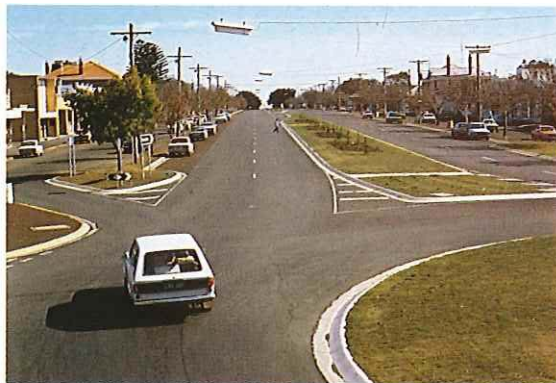
Hamilton Highway—duplication in Mortlake.
