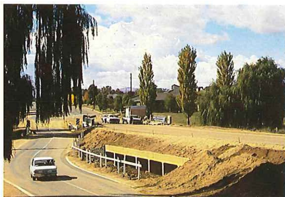
Pearce Street bridge under construction over House Creek in Wodonga.
