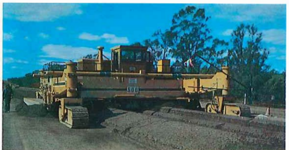
CMI Autograde in operation on the Hume Freeway, north of Avenel.
