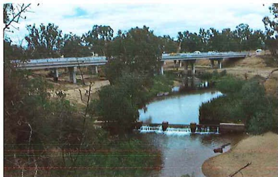
Hume Freeway, Avenel— twin 5 span bridges over Hughes Creek.
