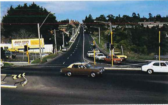
Reconstruction and widening of Princess Street, City of Kew.
