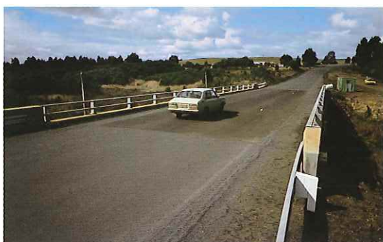
Lavers Hill-Cobden Road, new 4 span bridge over Kennedy Creek, Shire of Otway (Forest Road).
