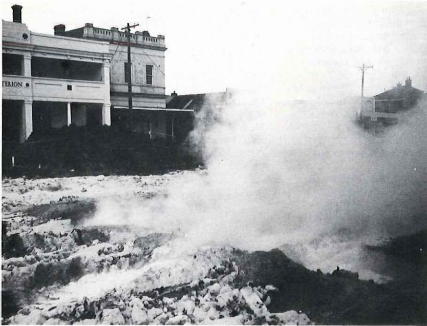
Plate 7: Hydration of quick lime — Princes Highway East of Trafalgar.
