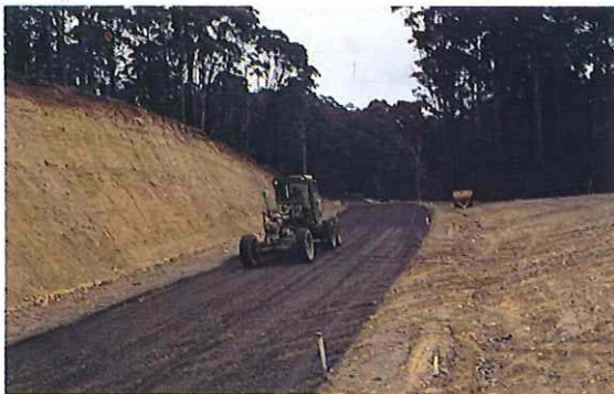
Greendale-Trentham Road, Shire of Balian— reconstruction north of Barry's Reef.
