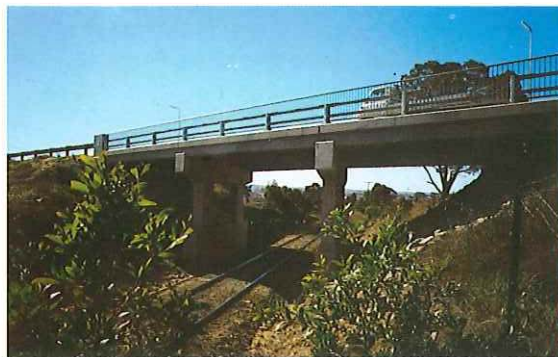
Forge Creek Road bridge over East Gippsland railway, Bairnsdale.
