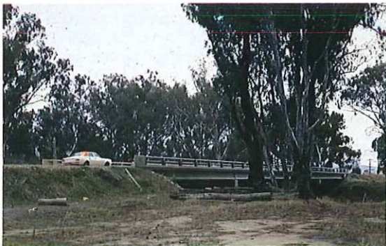
New 2 span bridge on the Violet Town-Dookie Road over the Broken River, Shire of Violet Town.
