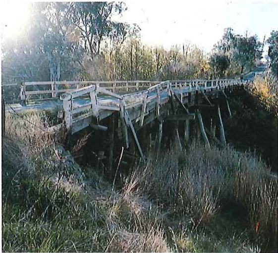
Typical examples of the deterioration in the main road system shown here indicate the need for urgent replacement of a timber bridge and the need for reconstruction of an existing sealed road.
