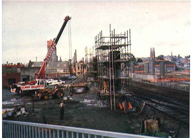
Latrobe Terrace bridge, Geelong
