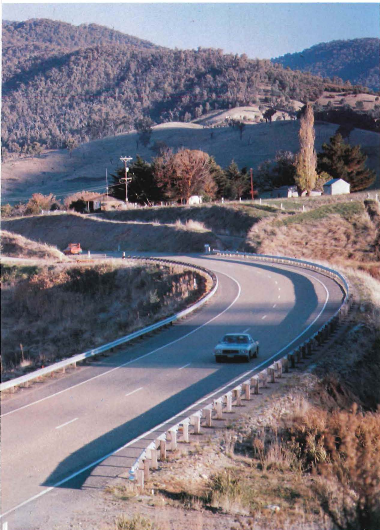
Kiewa Valley Highway at Running Creek — reconstructed section of highway.
