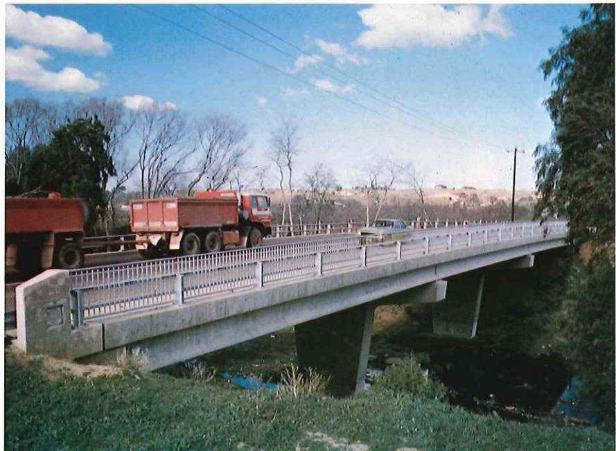
Fisken Street — a new 3 span bridge over the Werribee River, Bacchus Marsh Shire (Unclassified road).
