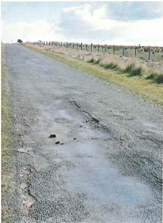
Typical examples of the deterioration in the main road system shown here indicate the need for urgent replacement of a timber bridge and the need for reconstruction of an existing sealed road.
