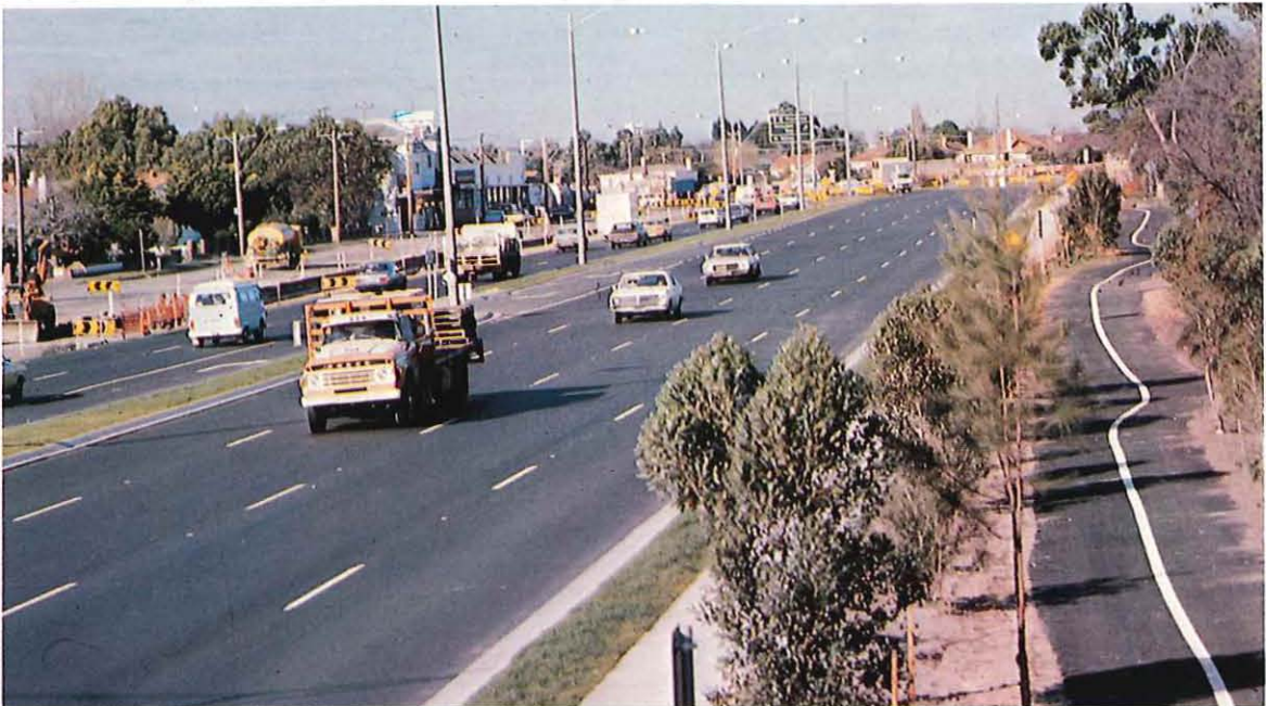
Nepean Highway, East Brighton — newly opened section of divided highway including a bicycle path threading its way through the plantation reserve adjoining the new road.
