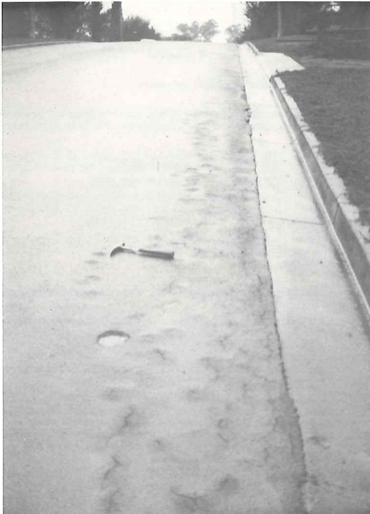
Figure 7 Sulphide affected pavement
