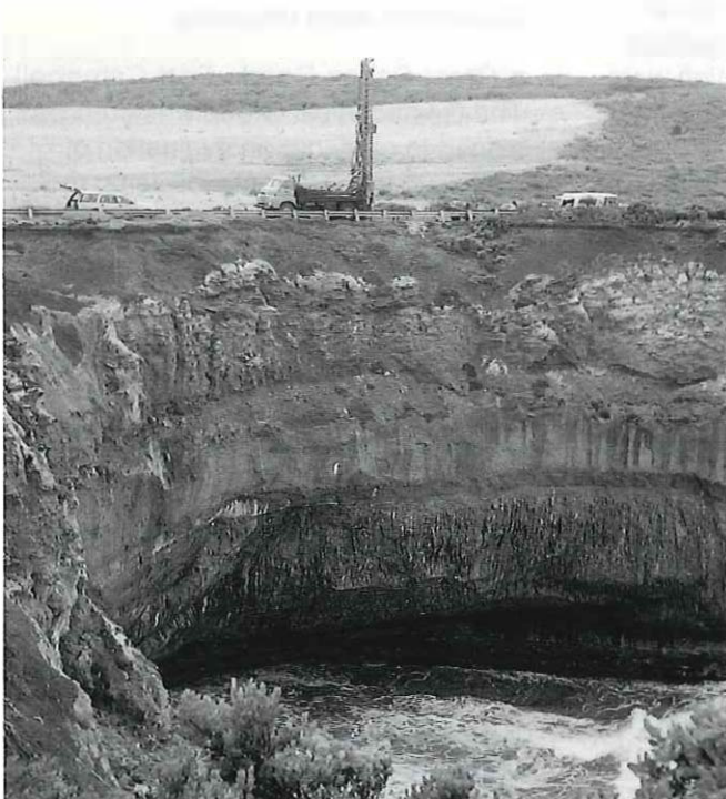
Investigation drilling to define the cavern – Great Ocean Road, Port Campbell.
