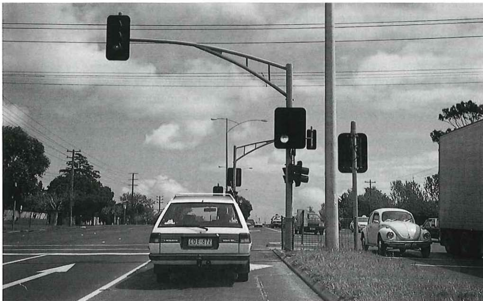
Accident Black Spot treatments: in this situation fully controlled right turn light sequences have been installed to reduce accidents for vehicles turning right across oncoming traffic.
