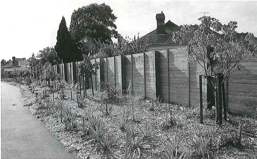
Landscaping of the Princes Highway East at Malvern, incorporating timber noise barriers.
