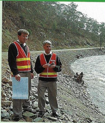
Mitta Mitta River alongside the Omeo Highway, north of Bruthen, is a site where riverbank protection works were carried out following flooding. VicRoads Highway Construction Engineer Carl Hodgkins (left) and Surveillance Officer John Harris (right) are pictured inspecting the results. Photo by Michael McLeod.
