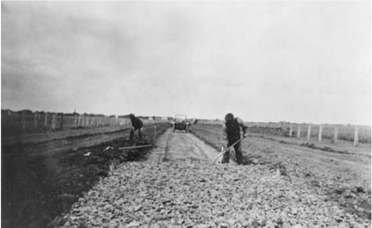
Construction works between Melbourne and Geelong, 1913
