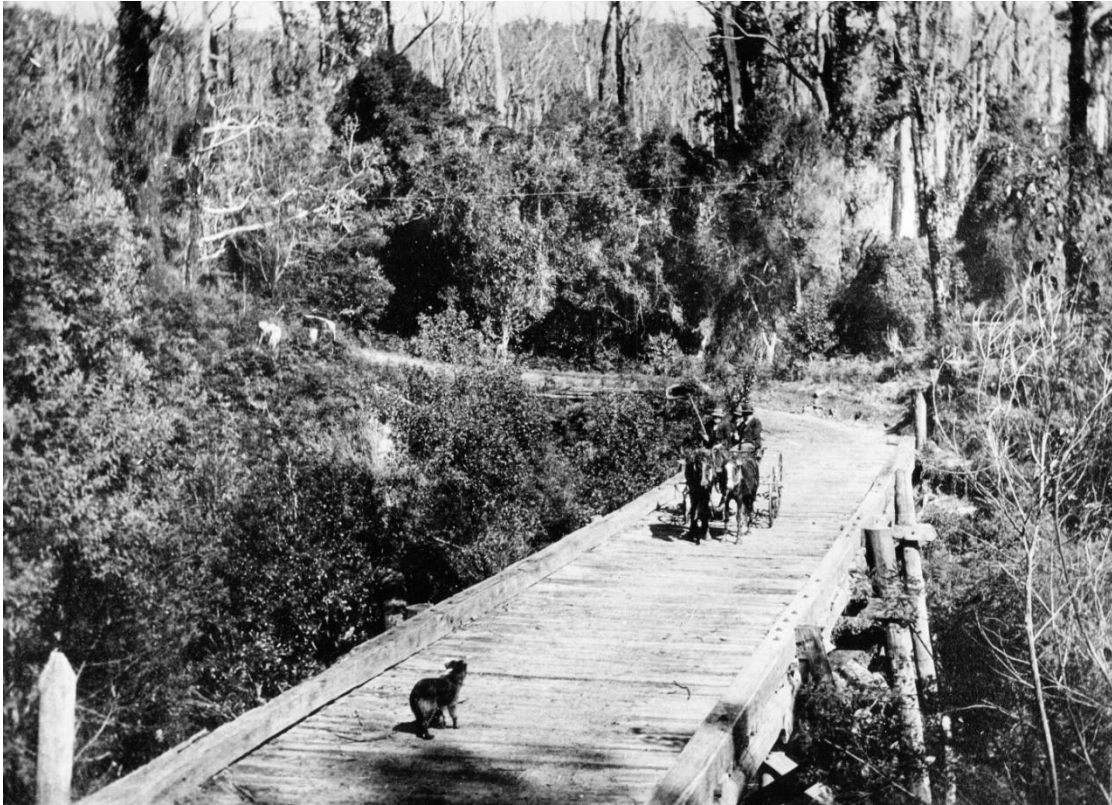
Bridge over Bemm River, Gippsland, 1913
