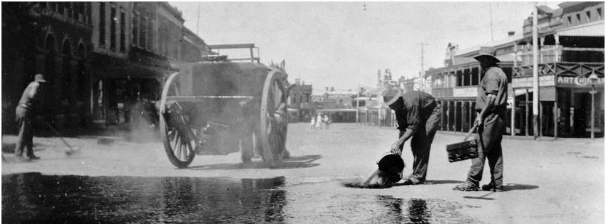
Surface painting with asphalt, Ararat, 1915
