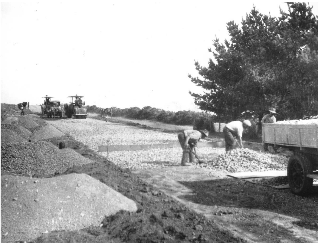
Western Highway, spreading base course at Burrumbeet, 1930
