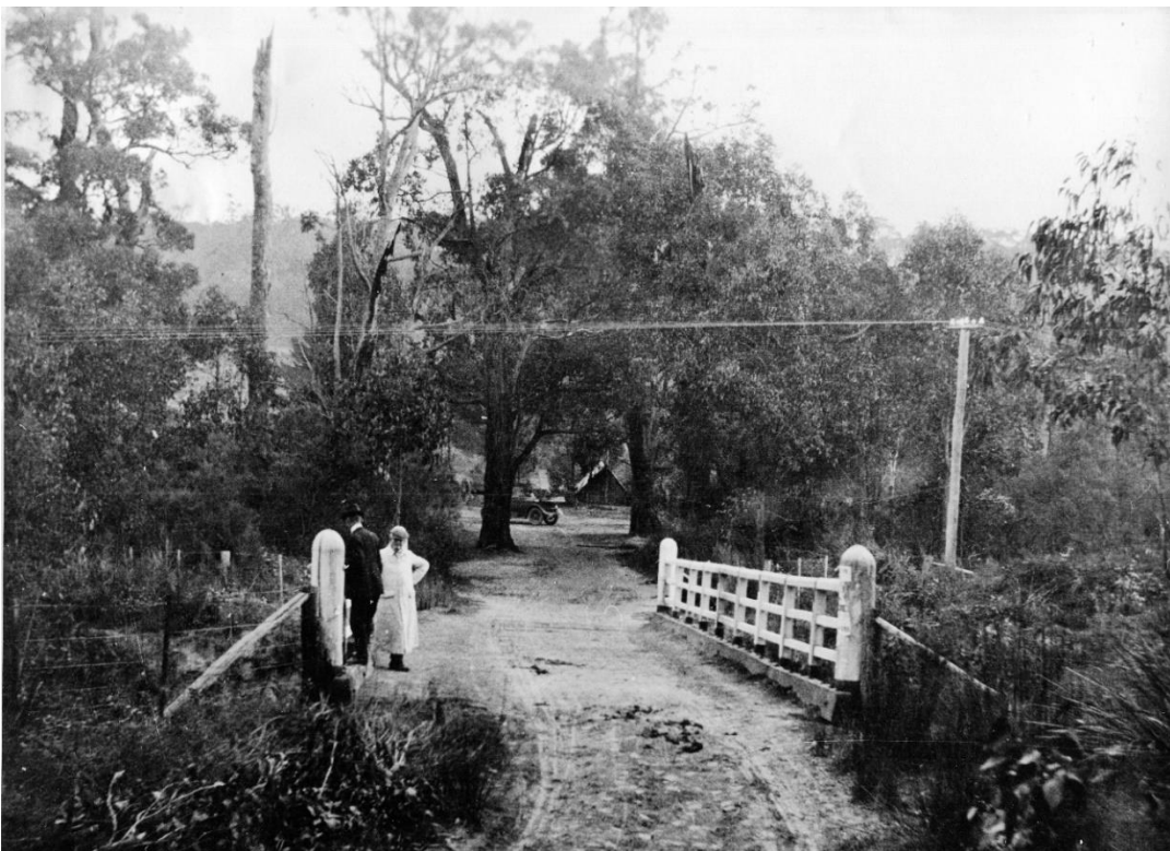
Inspecting bridge over narrow gauge railway, Belgrave, 1914
