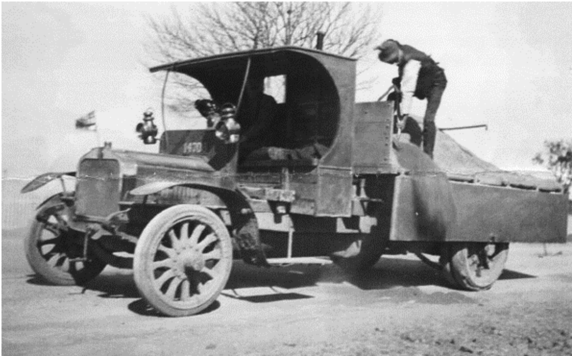
Unloading toppings for tar spraying, Fairfield 1914
