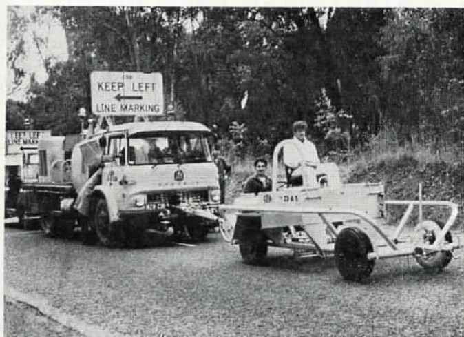
Teething troubles for 23-A-5 on the Warburton Highway. Last year this machine used 22,600 gallons of paint and striped 8,770 miles of standard stripe.
