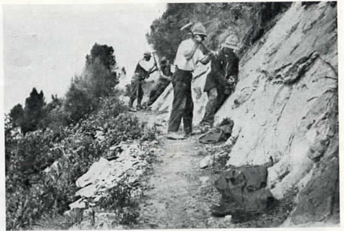
Hand drilling for explosives charges, Ocean Road.
