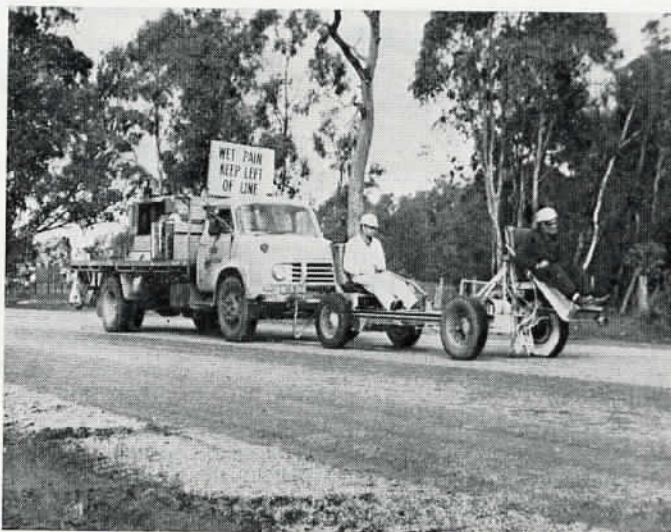
Western Highway near Horsham gets a restripe. This machine's useful life is over — after 27 years on the road.
