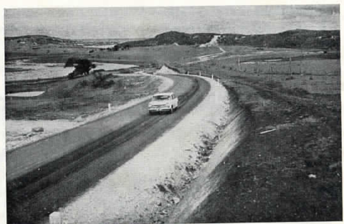
Continued on Page 9 Construction on new alignment north of Princetown.
