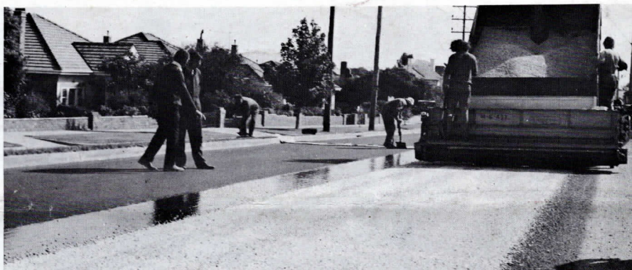
Laying pyrophyllite on North Road, Ormond.
