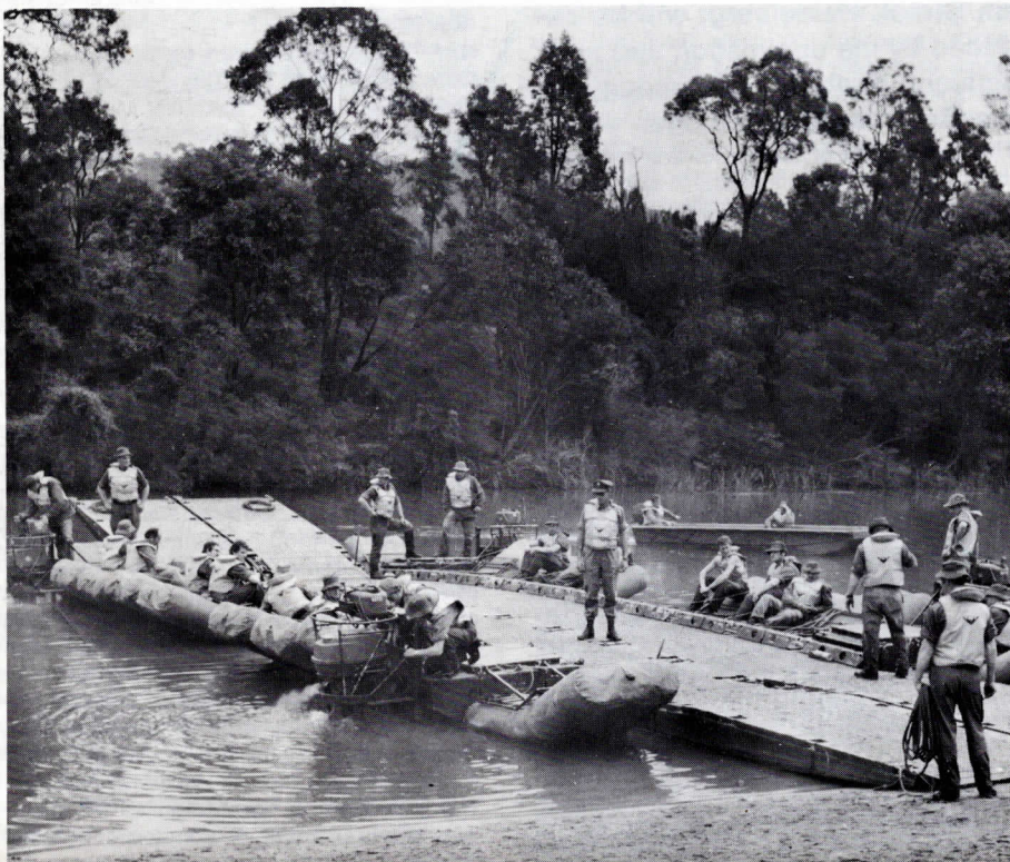
Members of 22 Construction Regiment, Army Reserve (C.M.F.), training on an air-portable bridge during the Annual Camp held in November, 1974, at the School of Military Engineering, Liverpool, N.S.W. Many members of 22 Construction Regiment are staff or employees of the C.R.B. (Army photograph).
