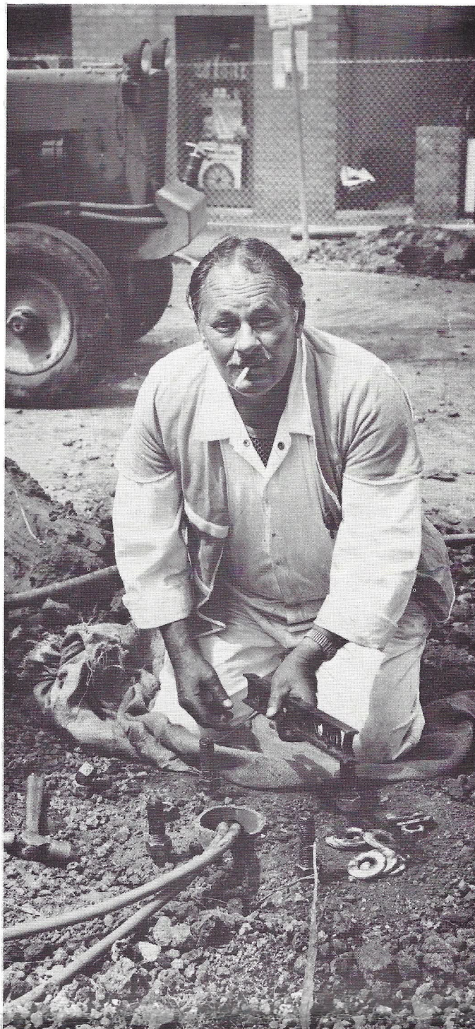
★ Jim Palasz (Syndal) levels bolts for signal pedestals.
