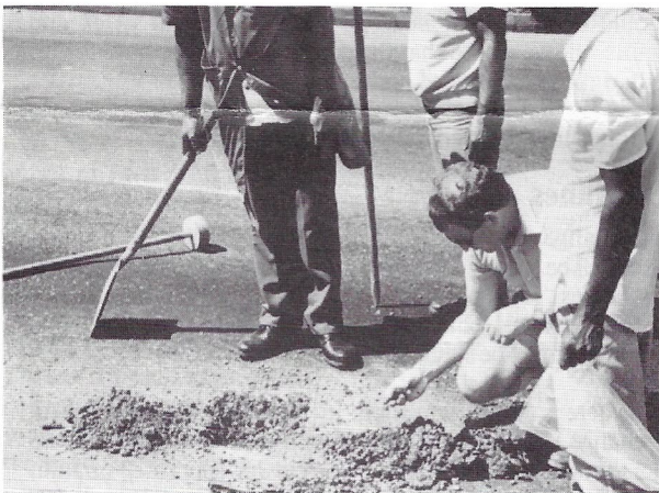
• 'So, that's how roads are made.' A curious Geoff Hose inspects a road.
