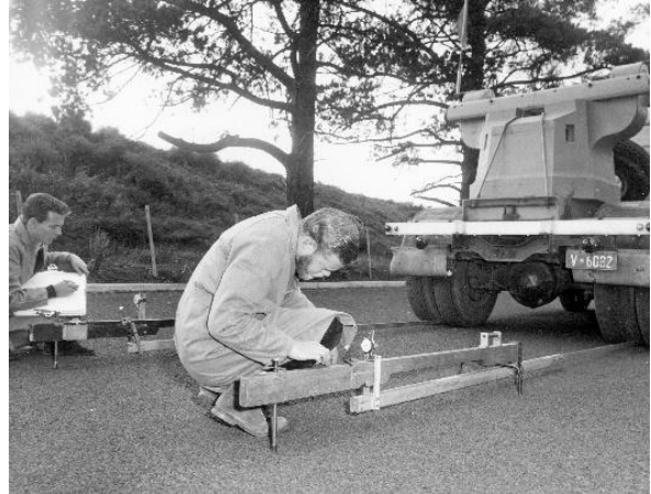
Benkelman Beam with Operator Peter Konings testing the Maltby Bypass, Princes Highway West
