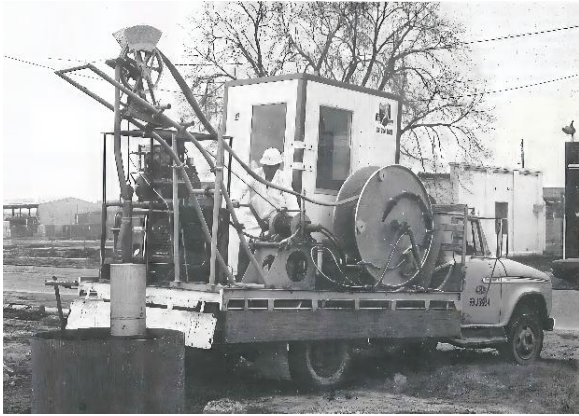
Lowering SID into the cylindrical pile casing
