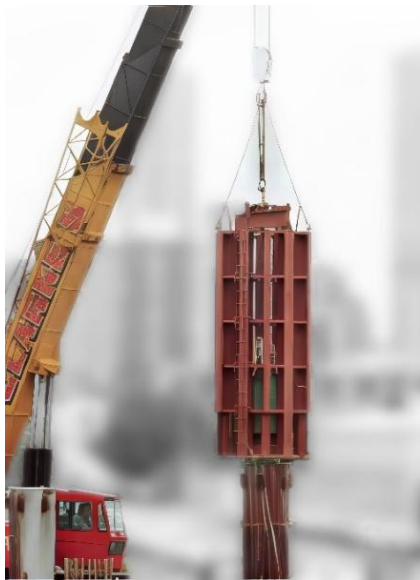
20-tonne hammer dropping onto pile
