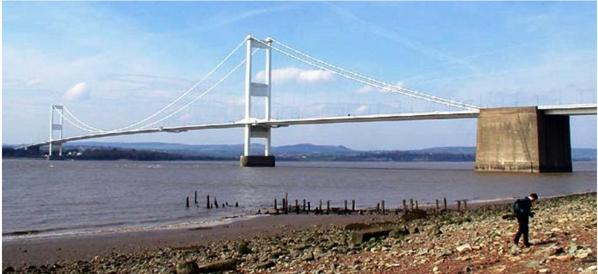
View of the Severn Bridge designed by FFP and opened in 1966.
