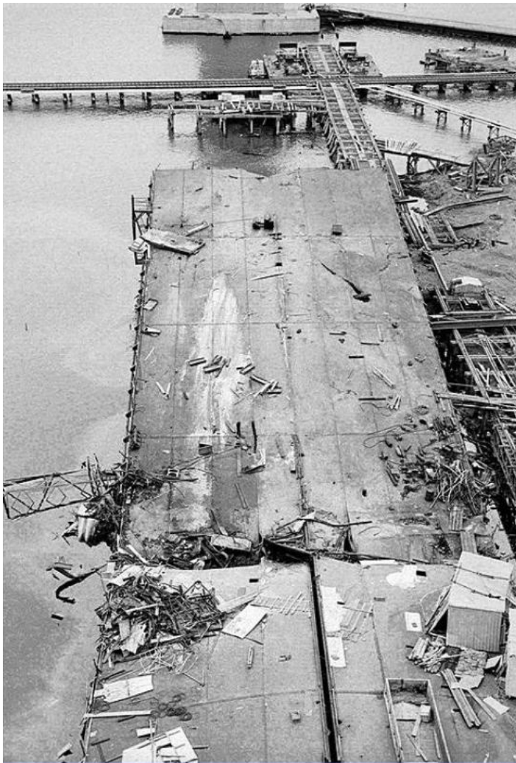
Looking down onto the fallen span from the top of Pier 10. (Images courtesy of Rob Morgan ARPS)
