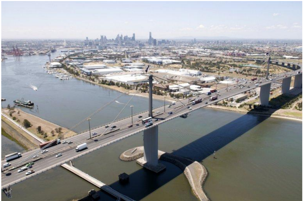
An aerial view of West Gate Bridge – date unknown
