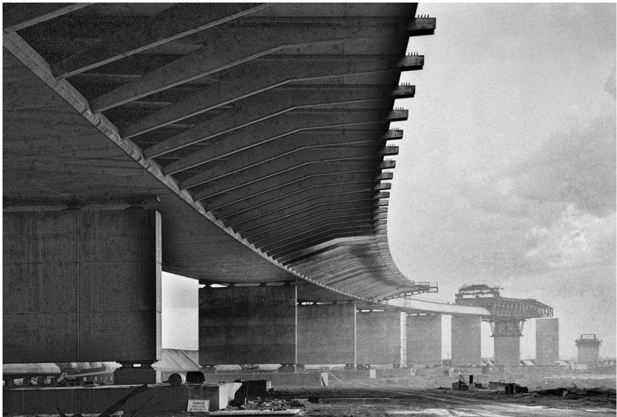
The eastern concrete approach spans being built, viewed from near Todd Road – May 1970. (Image courtesy of Rob Morgan ARPS)
