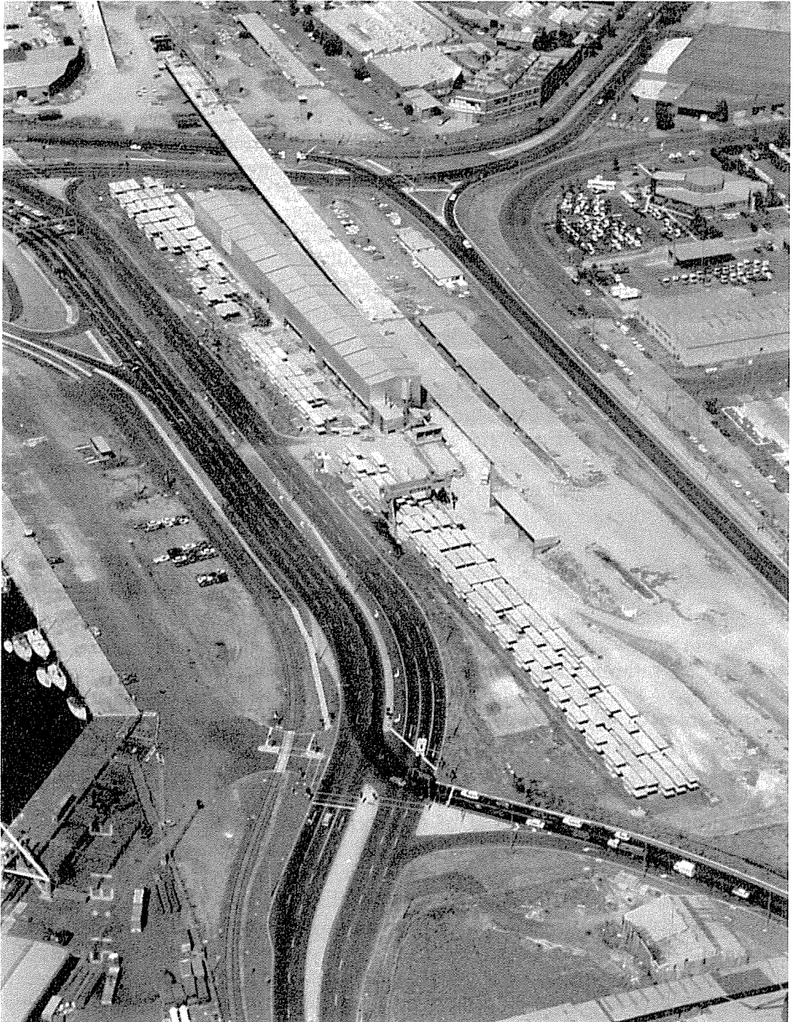
Fig. 19. Casting factory and segment storage yard
