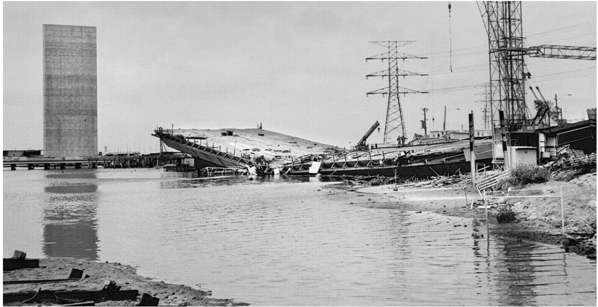
The fallen span beside Stony Creek, with Pier 12 on the left.
