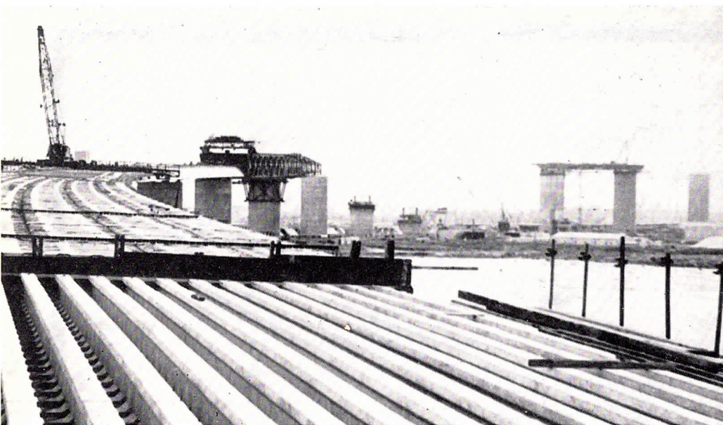
Eastern Approach with T beams over the east abutment in foreground.
