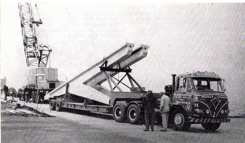
Concrete cantilevers arriving on site.
