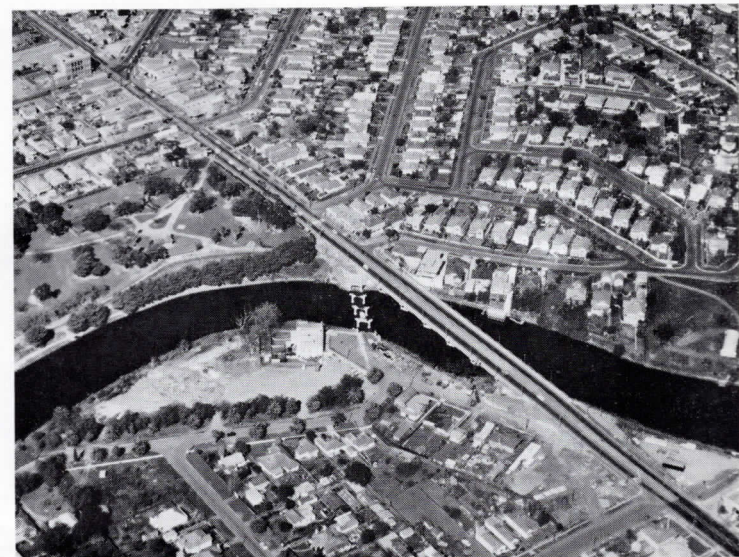
Aerial view of the new Maribyrnong Bridge. The alignment of the old bridge is clearly shown by the piers in the river before removal.
