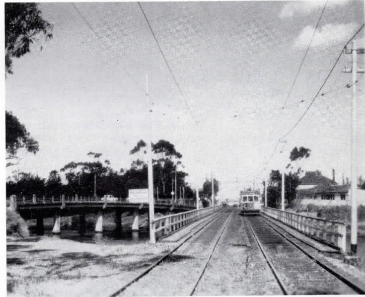
The old temporary tramway bridge with the road bridge on the left.
