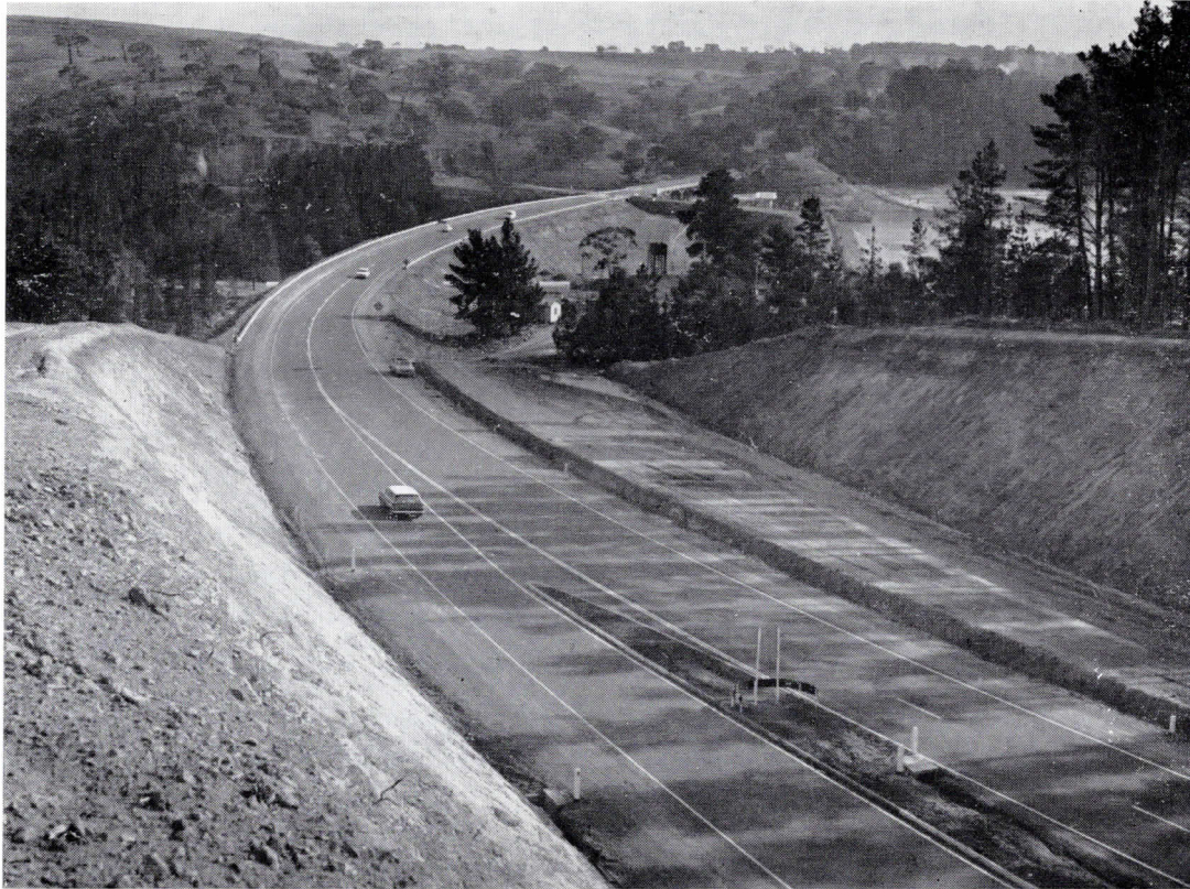
Western Highway at Pyke's Creek deviation looking west towards the spillway.
