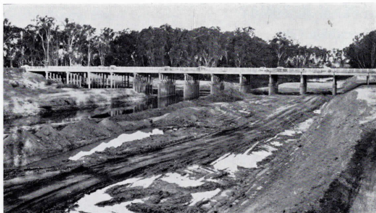
Right: Midland Highway Bridge No. 2 near Shepparton, showing flow of Goulburn River in new channel and strengthening of piles. Below: Map-gram showing Goulburn River diversion.
