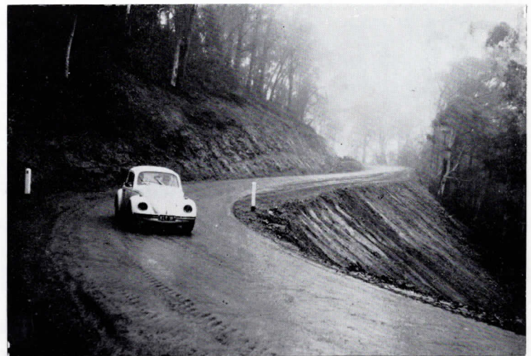
A widened section of the Omeo Highway, north of Mt. Wills in the Shire of Omeo.
