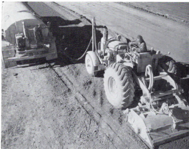
The picture above shows C.R.B. lime slurry operations on the Northern Highway north of Rochester, in the Shire of Rochester.
