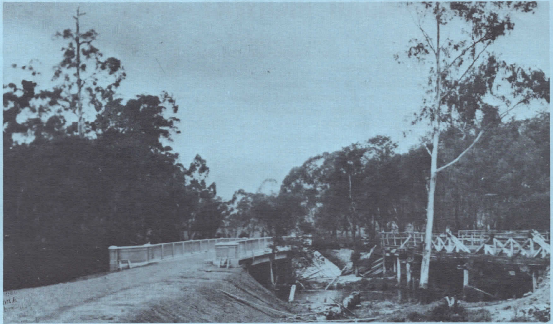
Above: Yesterday— Original bridge over Yarra River (right). Bridge built in 1919 (left) and now replaced by the new Maxwells Hill deviation.
